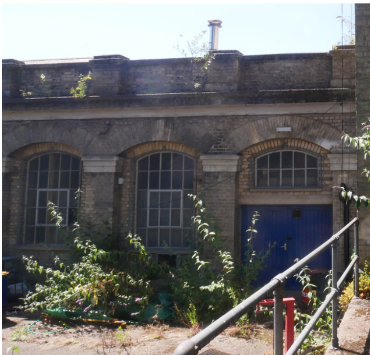
Location: Karslake - Boiler House
