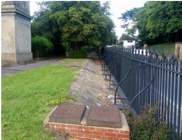
Figure 2.5: Raised ground and manholes (potential underground tank) in the north east corner of the site.
