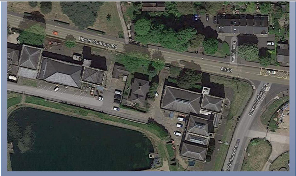
Hampton Water Works - Aerial Photo (Google maps)
