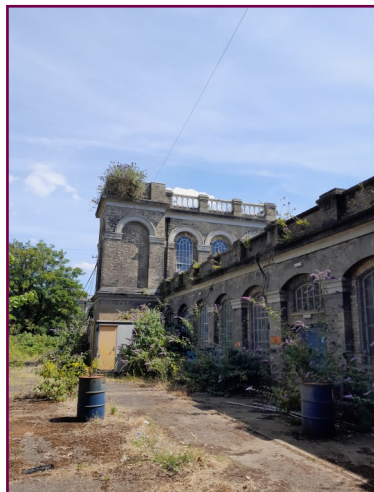
Photograph 5: Scattered vegetation on buildings and ground
