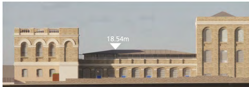
Updated roof extension
