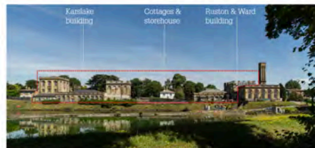
Existing view from Lower Sunbury Rd
