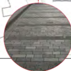
Shared surface paving Subtle paving changes uses size, colour and texture of pavers to denote parking spaces and vehicle movement lines while providing pedestrian priority across the site.
