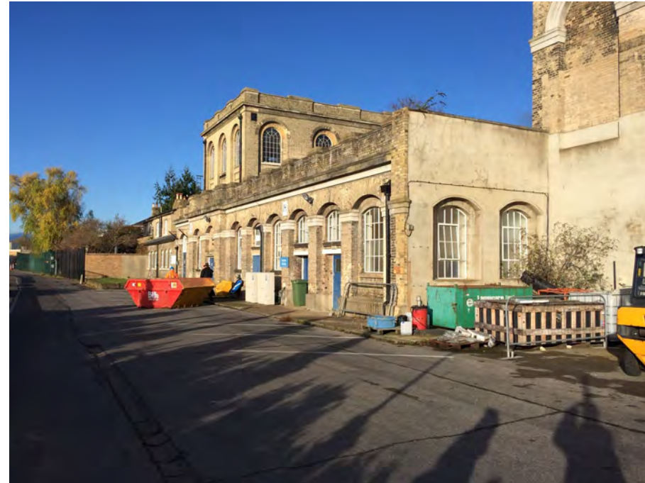
Figure 48: The rear of Karslake Building
