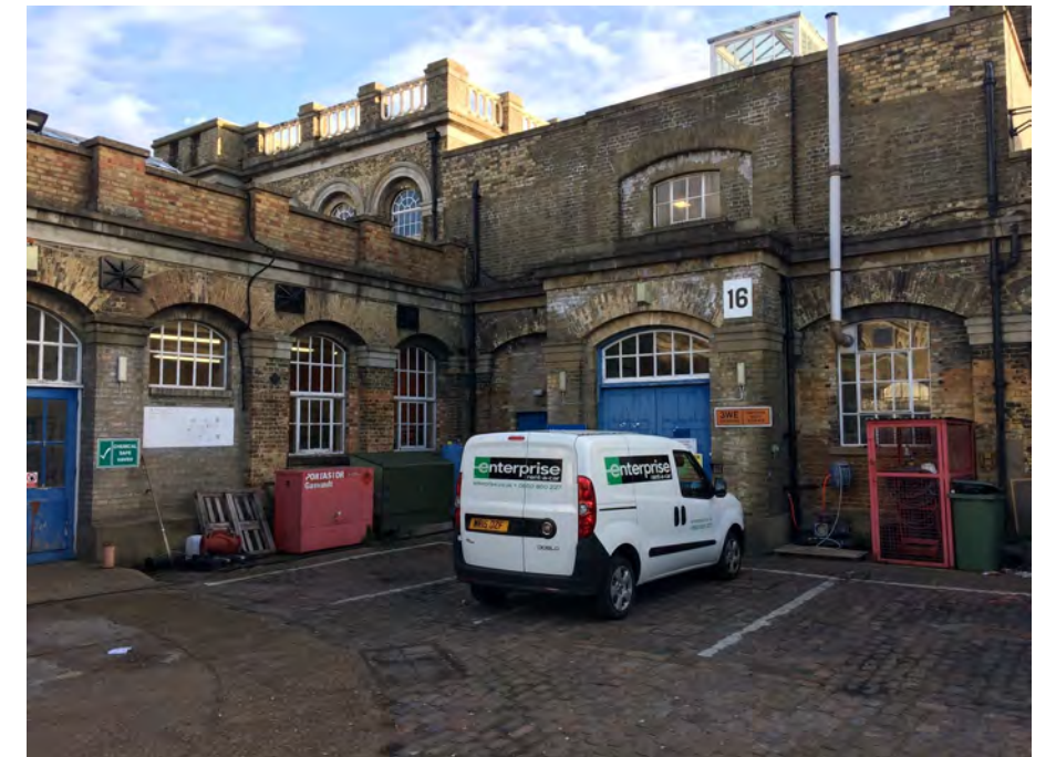
Figure 28: The rear of Ruston Building
