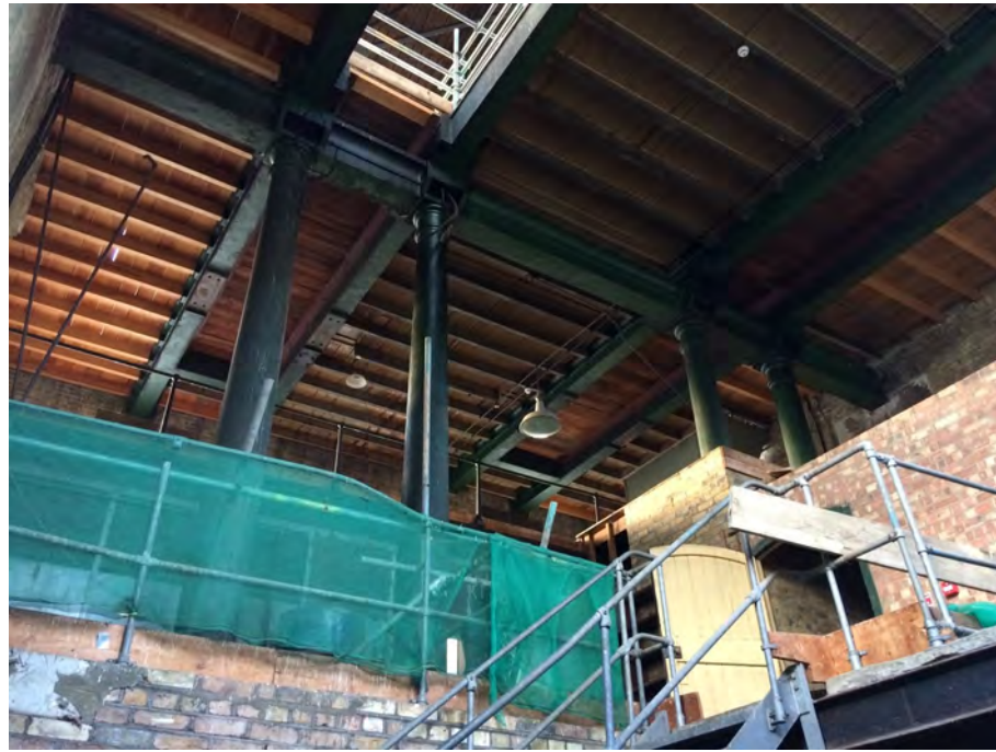
Figure 53 : The interior of Karslake Building's 'The Beam'
