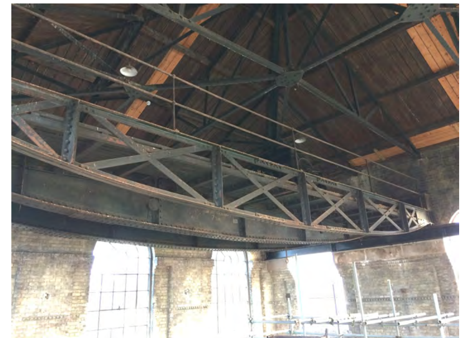
Figure 64: Large steel gantry within The Beam
