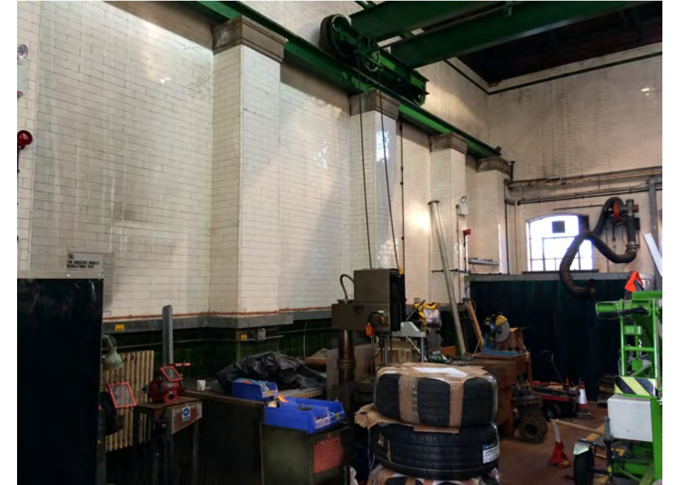
Figure 43: The interior of Ruston Building's southern block with Victorian white and green wall tiles
