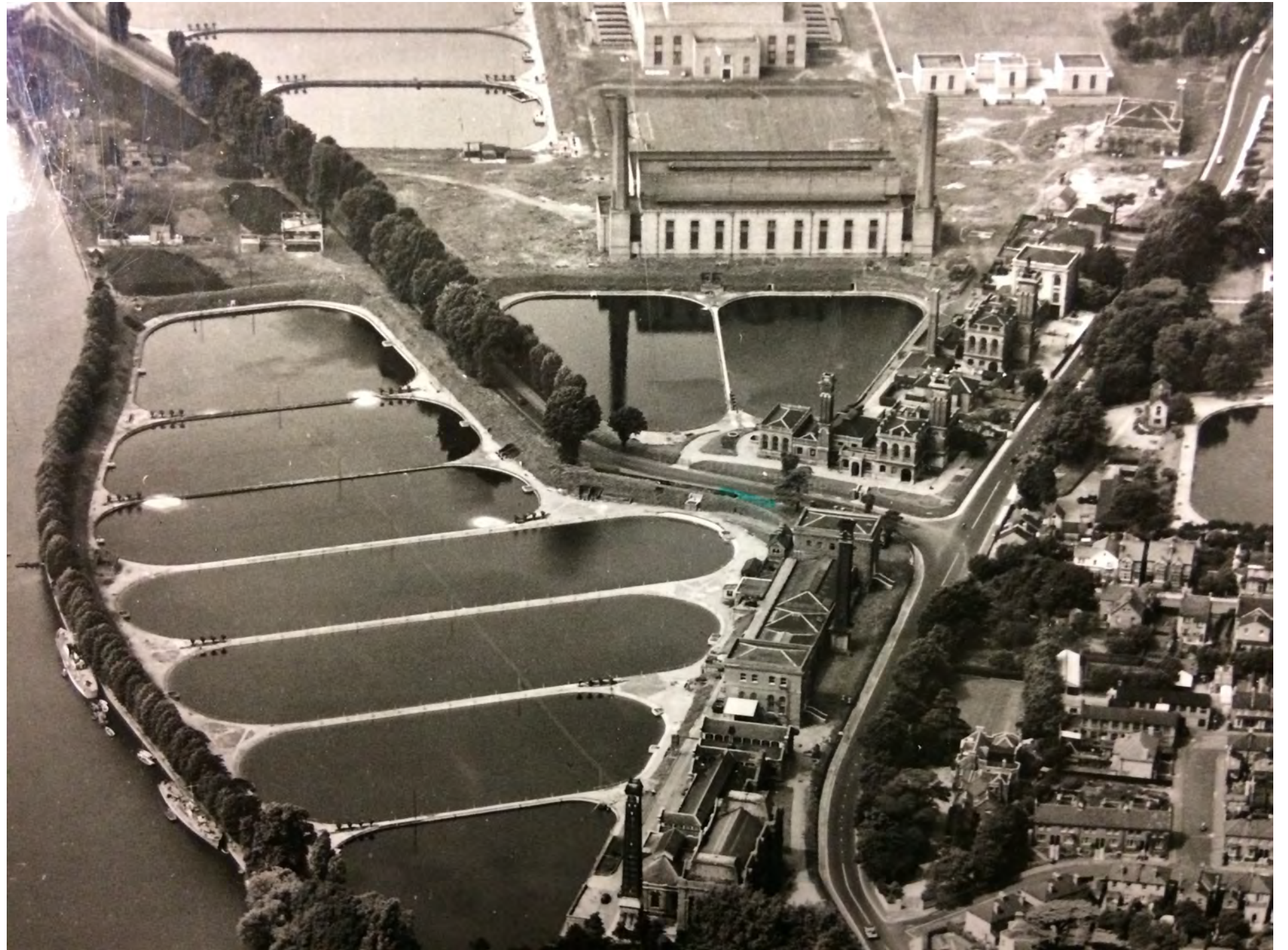
Figure 09: A aerial photo of Hampton Waterworks taken in July 1950 showing the engine pump houses before the demolition of their chimneys and Karslake Building's large nineteenth century rear extension (Richmond upon Thames Local Studies Library and Archive, 1950)
