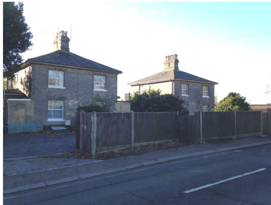
Figure 93: Nos. 6-9 Upper Sunbury Road (Buildings of Townscape Merit)
