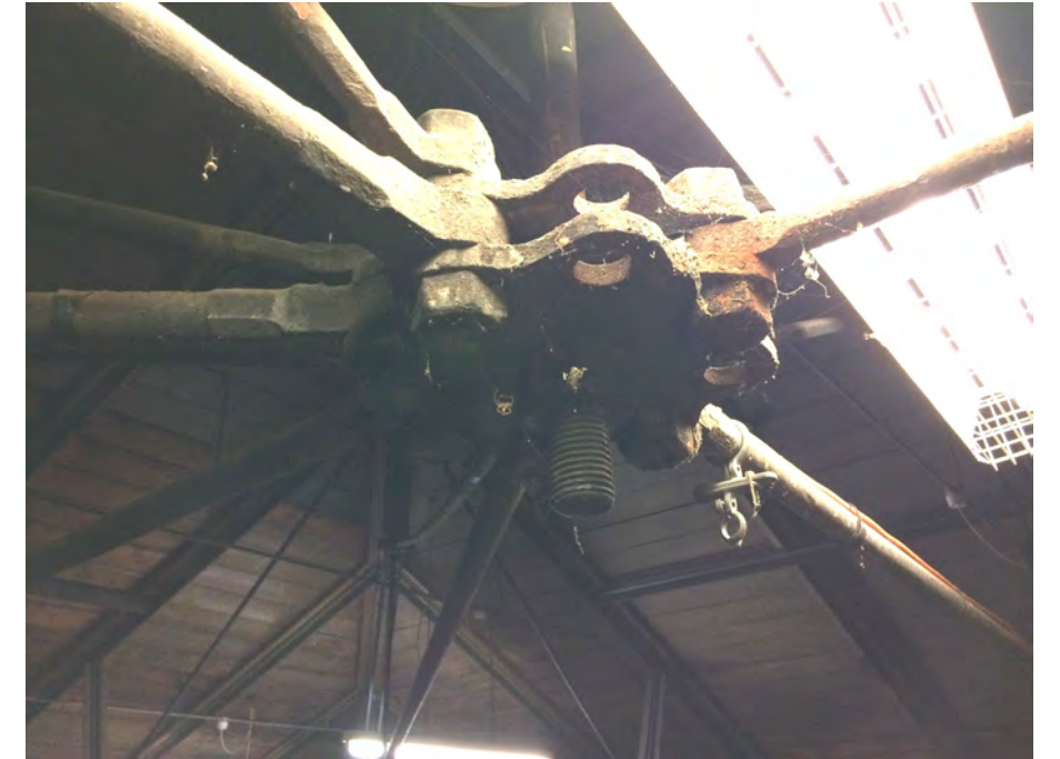
Figure 73: Detail of composite wrought iron truss roof
