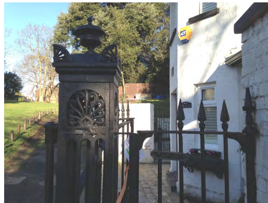
Figure 91: Entrance Gates to Rose Hill (Grade II)
