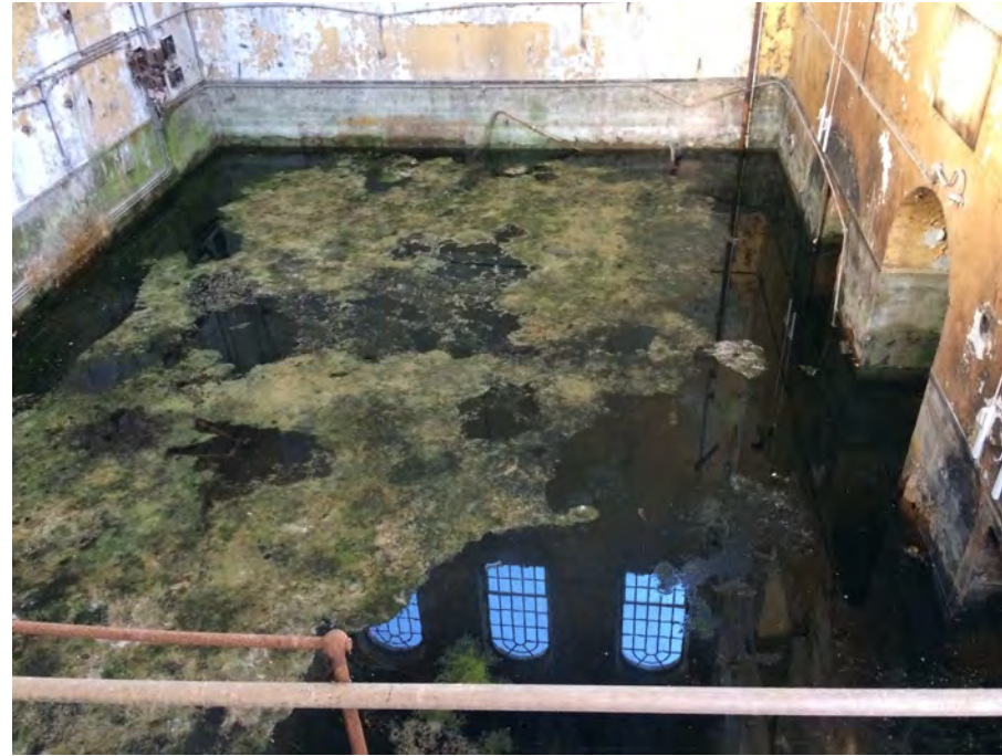
Figure 75: The derelict interior of Karslake Building's eastern engine house
