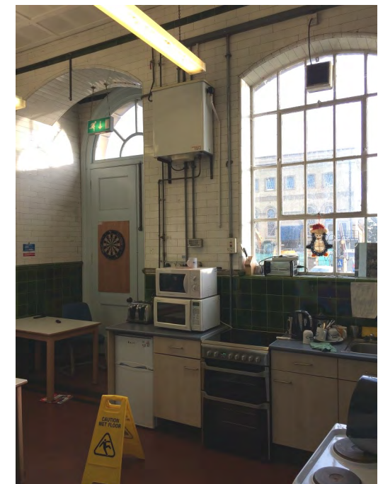
Figure 40: The tile-clad interior of Ruston Building's porch on Lower Sunbury Road which is currently being used as a kitchenette
