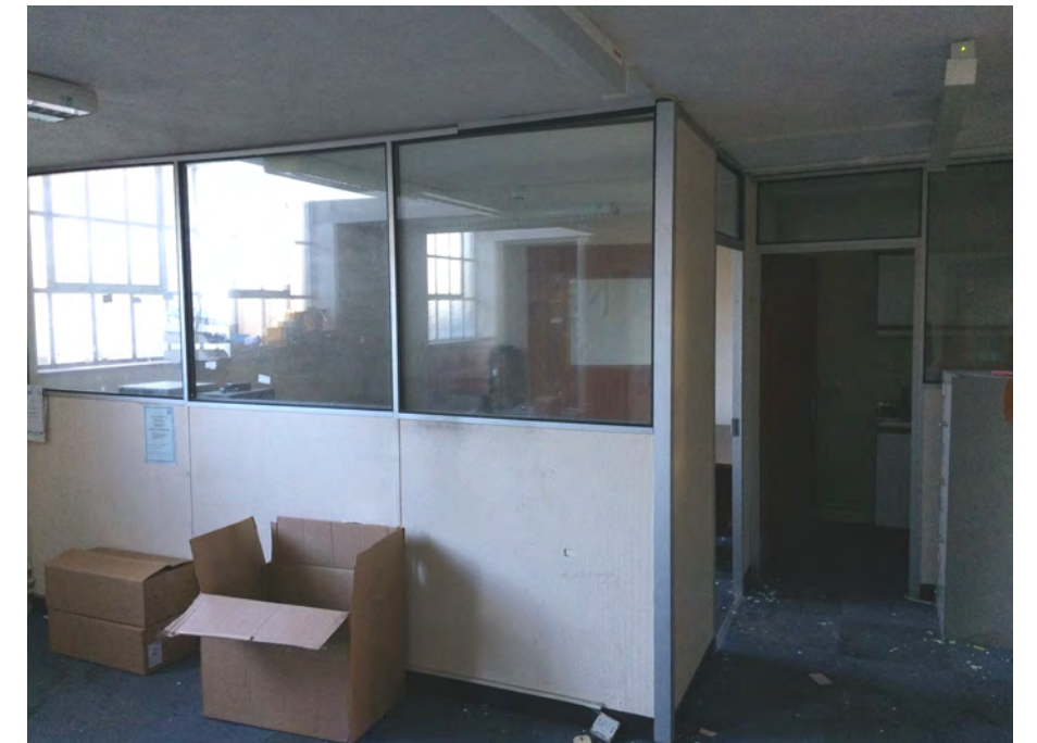
Figure 70: Twentieth century partitions within Karslake Building's boiler house
