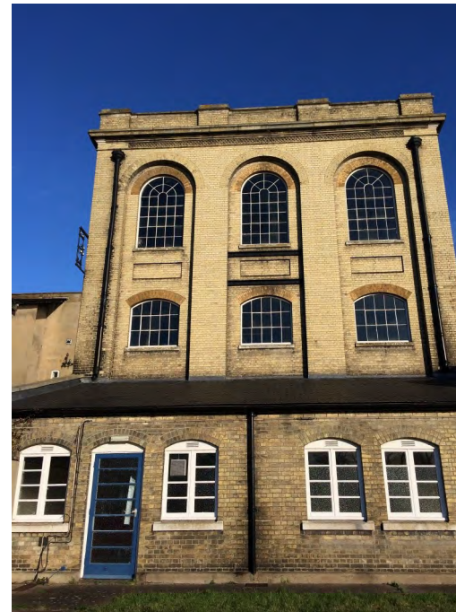
Figure 51: The rear of Karslake Building's western engine house, known as 'The Beam'
