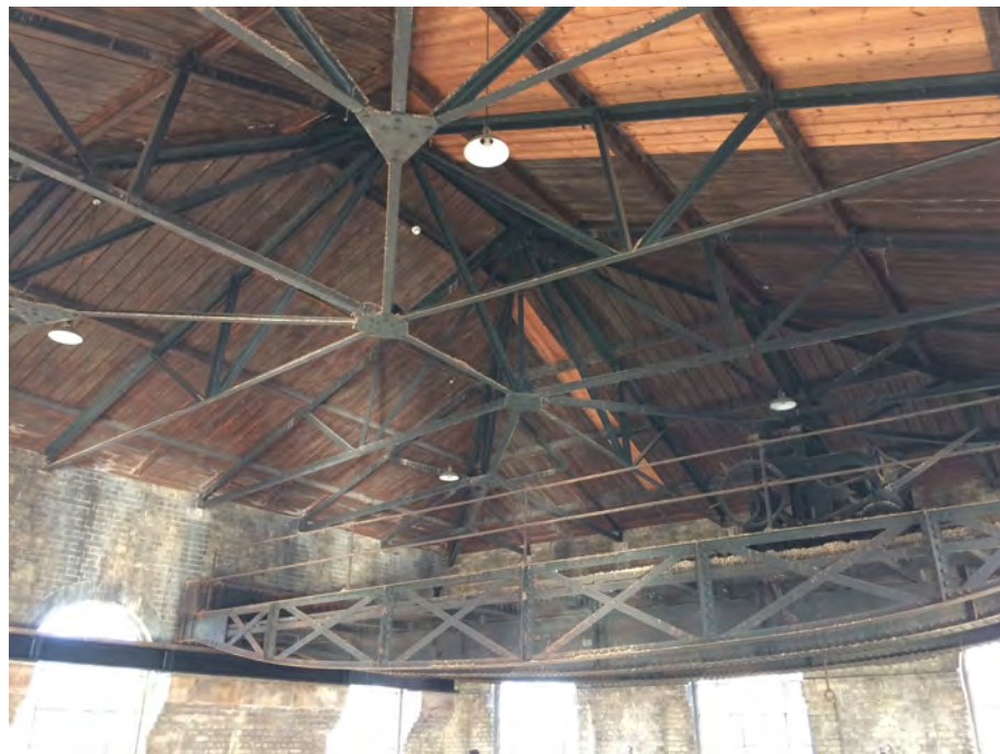
Figure 62: The Beam's steel truss roof
