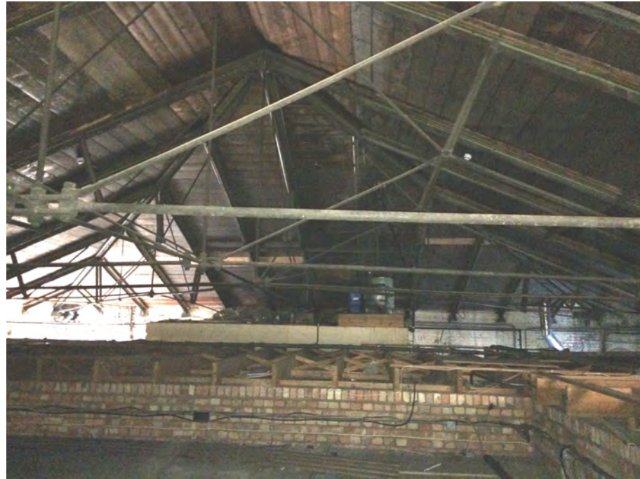
Figure 71: Composite wrought iron truss roof within Karslake Building's boiler house
