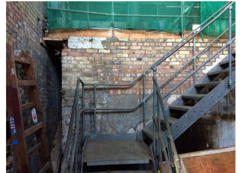
Figure 58: Modern steel staircase leading up to The Beam's first floor
