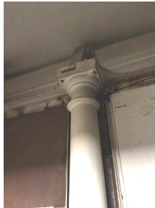
Figure 57: Tuscan order cast-iron columns
