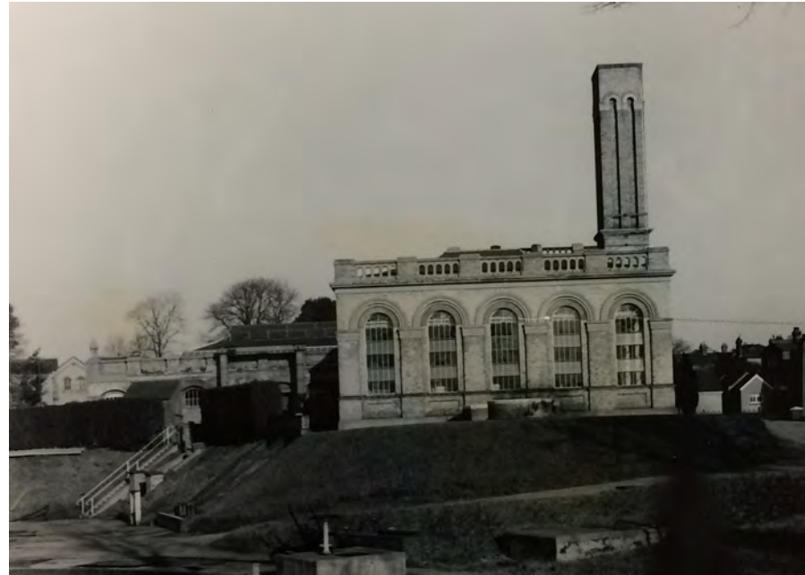
Figure 24: Ruston Building as viewed from Lower Sunbury Road in 1970 (Richmond upon Thames Local Studies Library and Archive, 1970)
