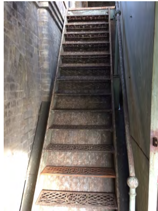
Figure 60: Steel staircase with decorative perforated treads leading up to The Beam's second floor
