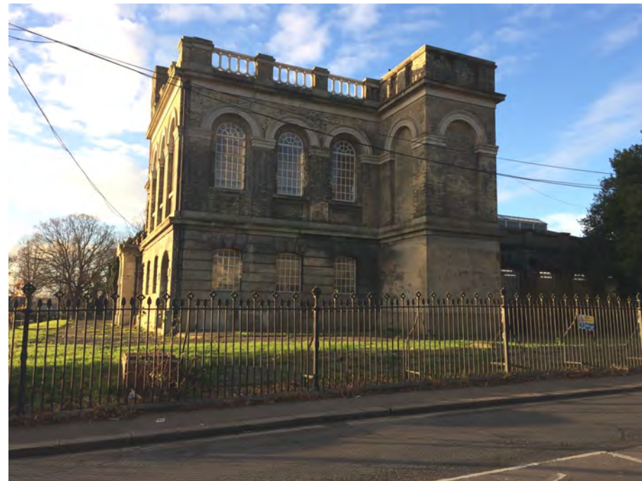
Figure 26: The Grade II listed Ruston Building as viewed from Upper Sunbury Road
