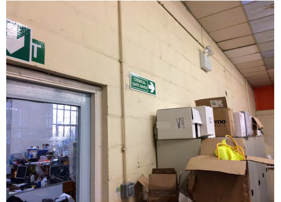
Figure 31: Concrete block subdivisions within Ruston Building's boiler house
