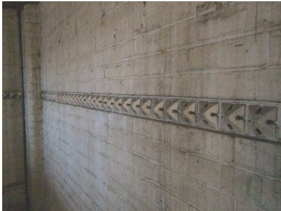
Figure 56: Dog-tooth detailing set within the walls
