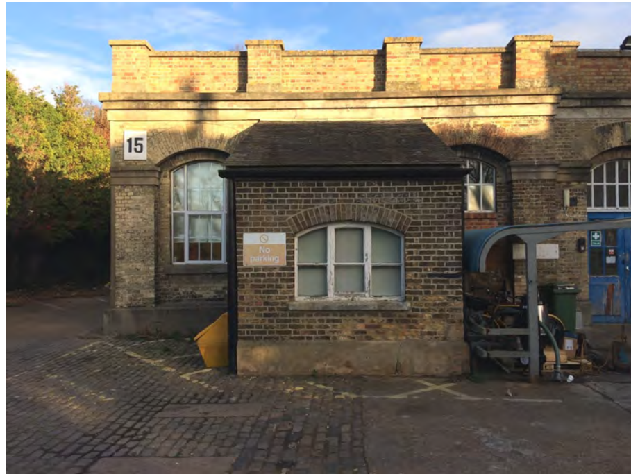
Figure 29: The rear of Ruston Building with a late-nineteenth century lean-to extension
