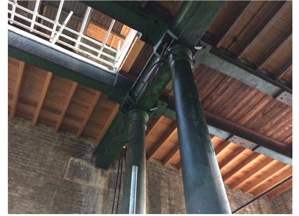
Figure 55: Tuscan order cast-iron columns
