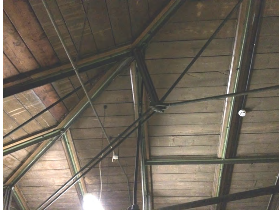
Figure 72: Composite wrought iron trusses and timber sarking boards
