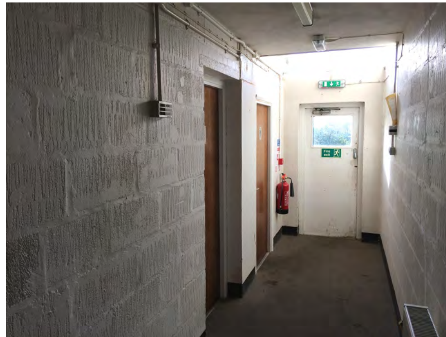
Figure 69: Twentieth-century concrete-block subdivisions within Karslake Building's boiler house
