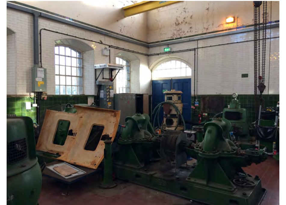
Figure 37: The interior of Ruston Building's engine house with non-original steel windows and Victorian white and green wall tiles
