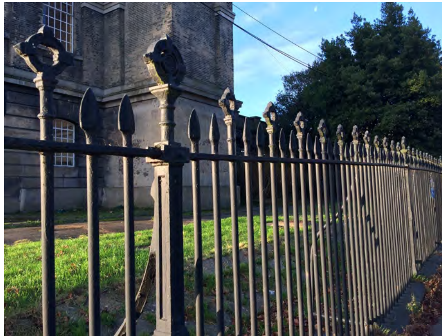
Figure 27: The Grade II listed cast iron railings that bound Ruston Building to the north and east
