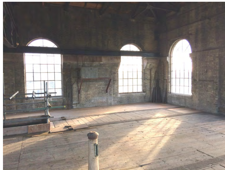
Figure 63: The Beam's second storey with cast-iron round-headed windows
