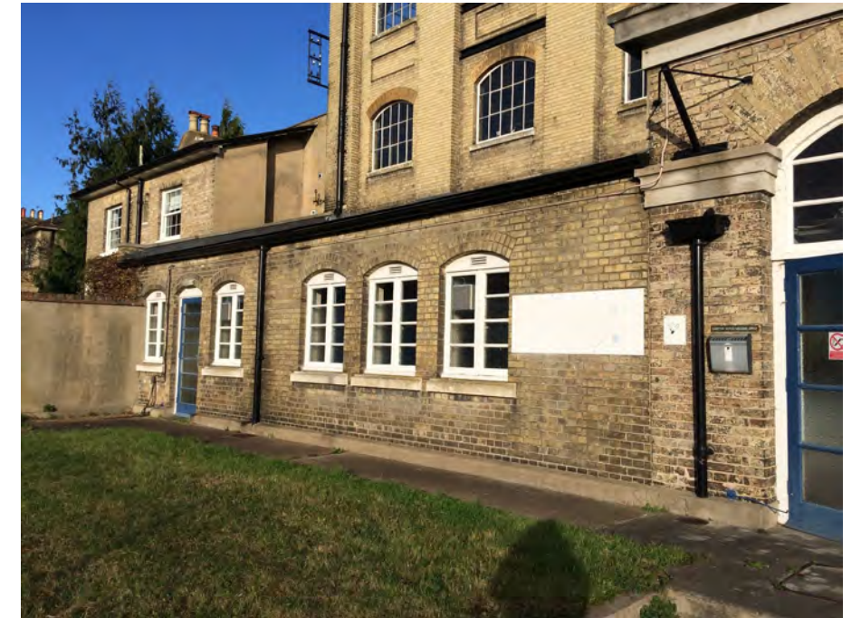
Figure 52: The rear of Karslake Building's western engine house, known as 'The Beam'
