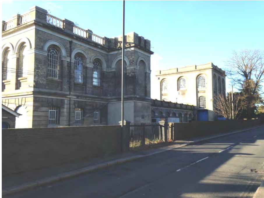
Figure 47: Karslake Building as viewed from Upper Sunbury Road
