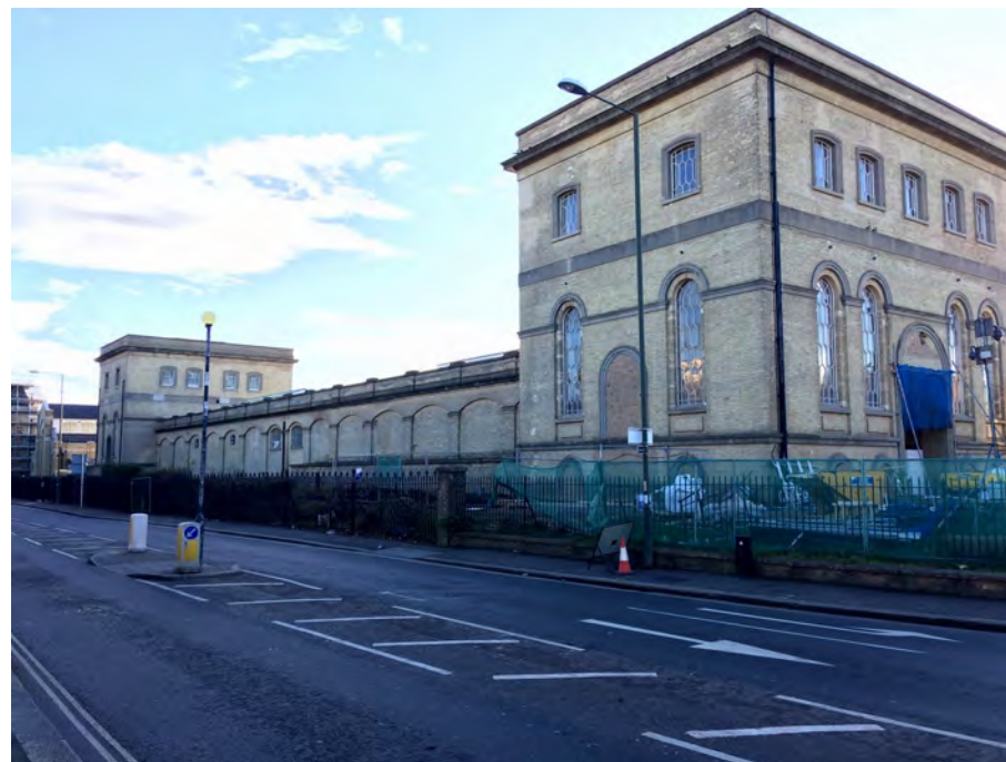
Figure 87: Morelands Building (Grade II)
