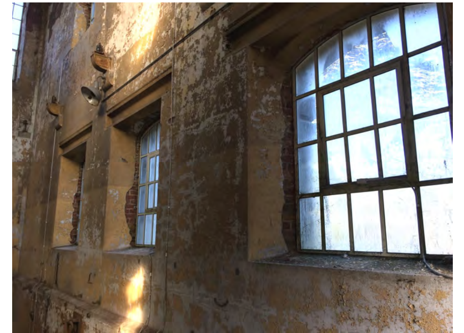
Figure 76: Non-original steel windows within Karslake Building's eastern engine house
