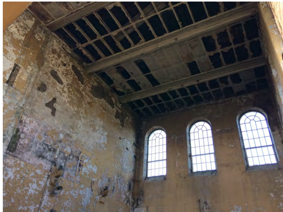
Figure 74: The derelict interior of Karslake Building's eastern engine house with non-original steel round-headed windows
