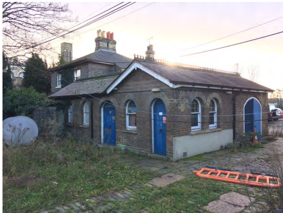
Figure 84: L-shaped storage building
