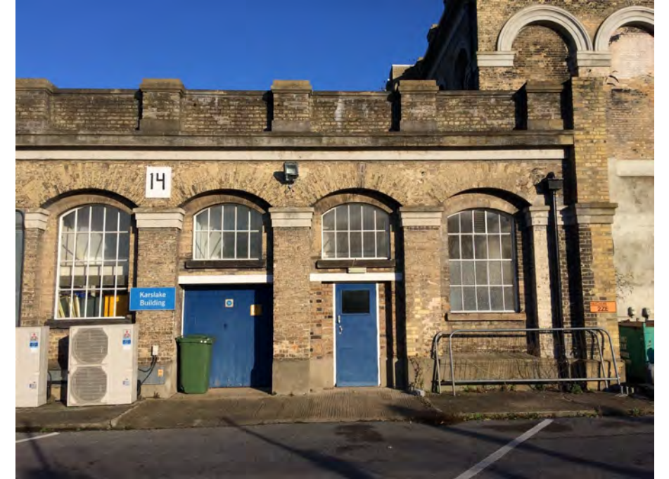
Figure 49: The rear of Karslake Building's central block
