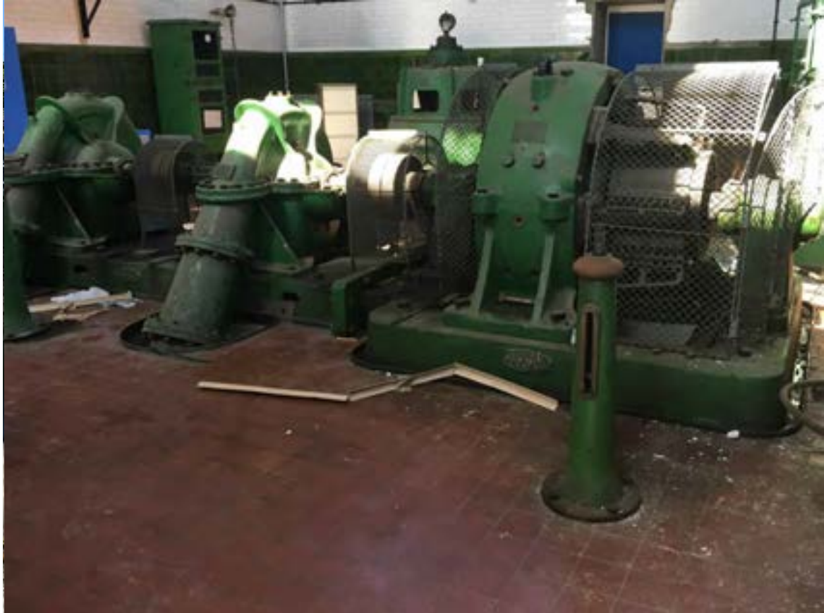
Plate 11: 2019 View of surviving machinery within Ruston & Ward building
