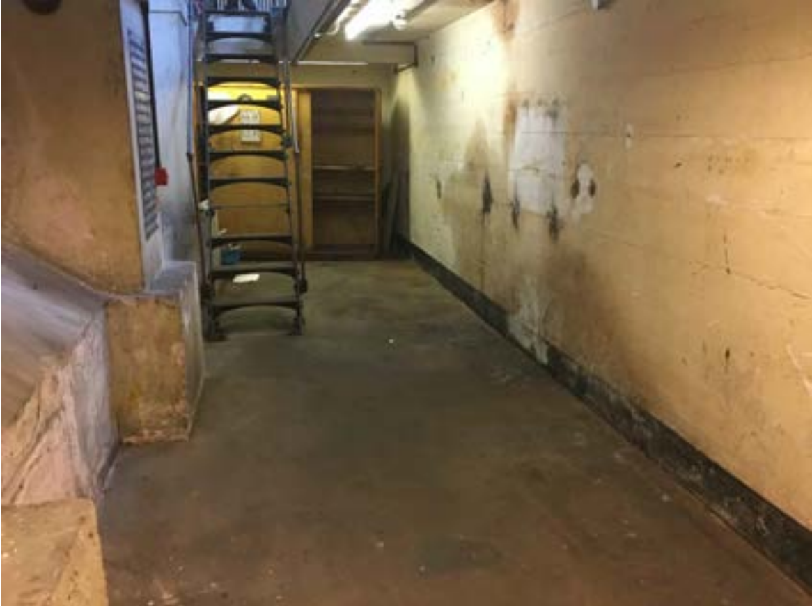
Plate 13: 2019 View within existing basement within central area of Ruston & Ward building
