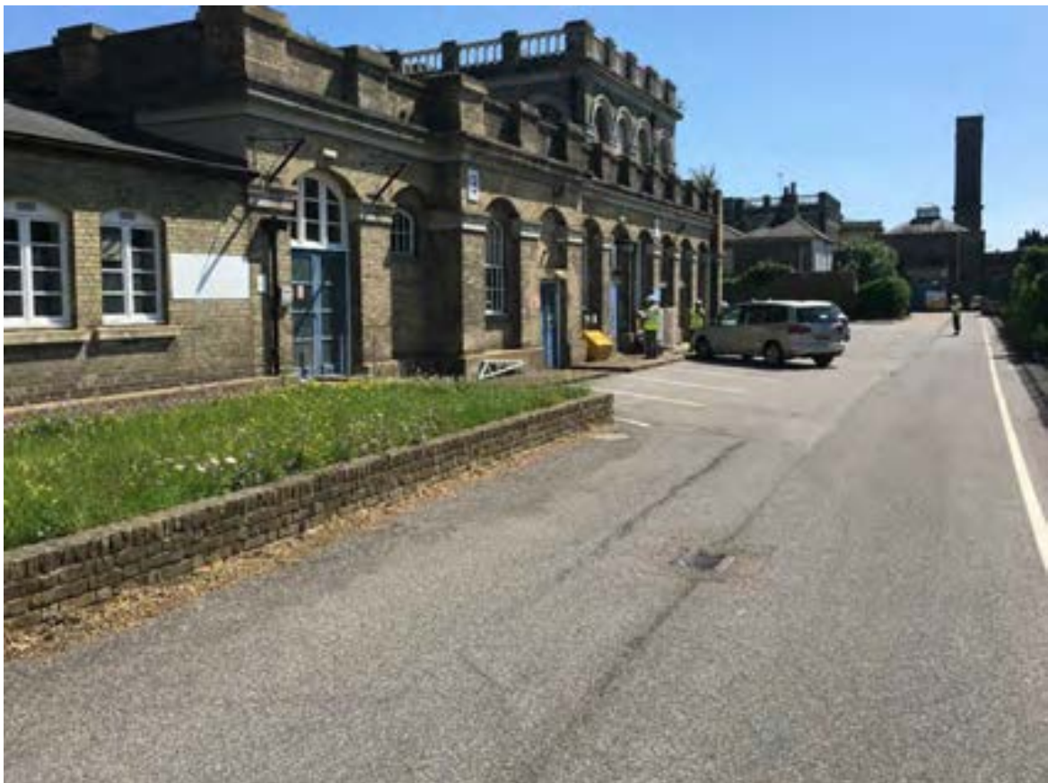
Plate 8: 2019 View facing east along southern site boundary
