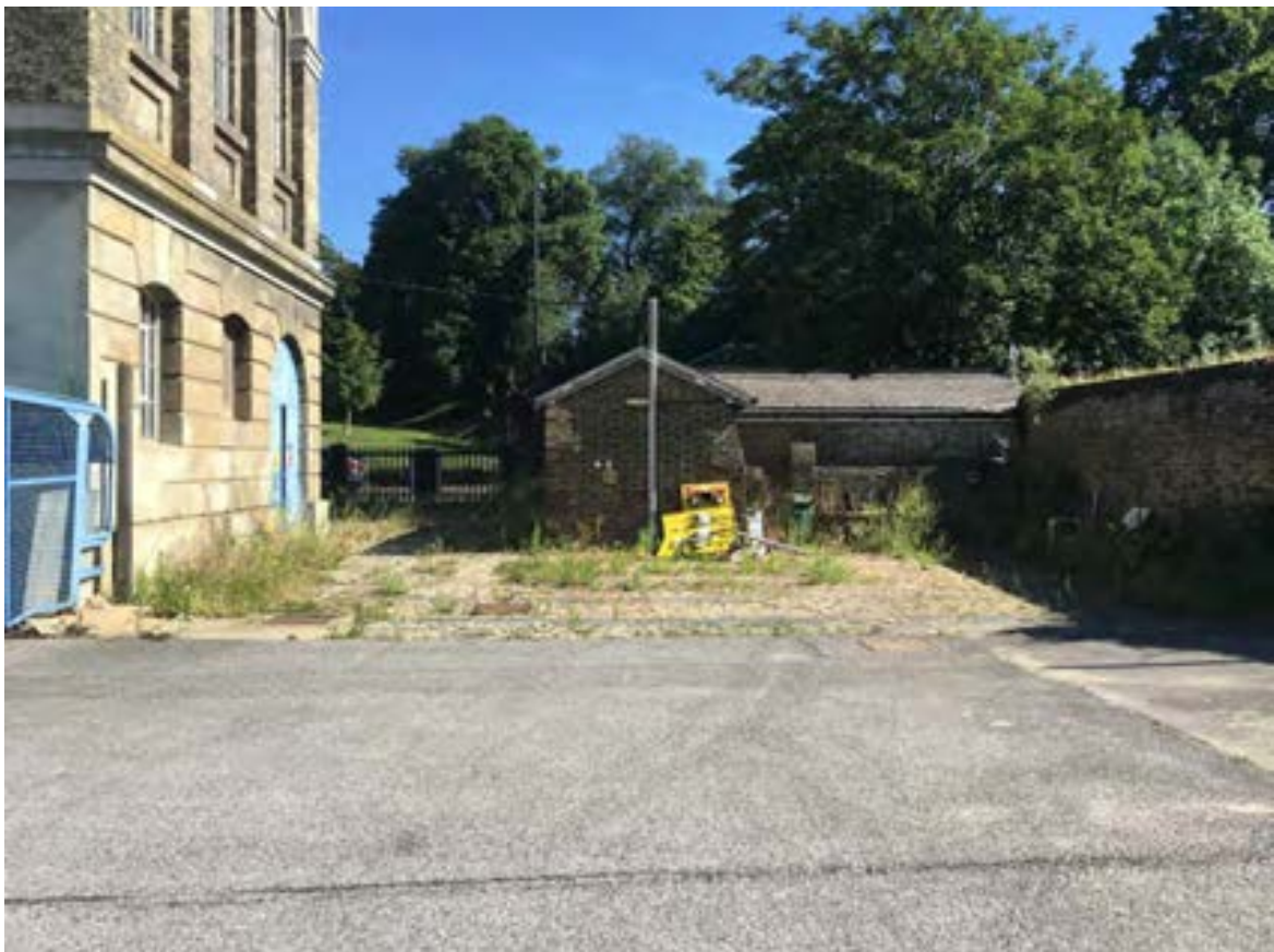
Plate 10: 2019 View of buildings in central area of site
