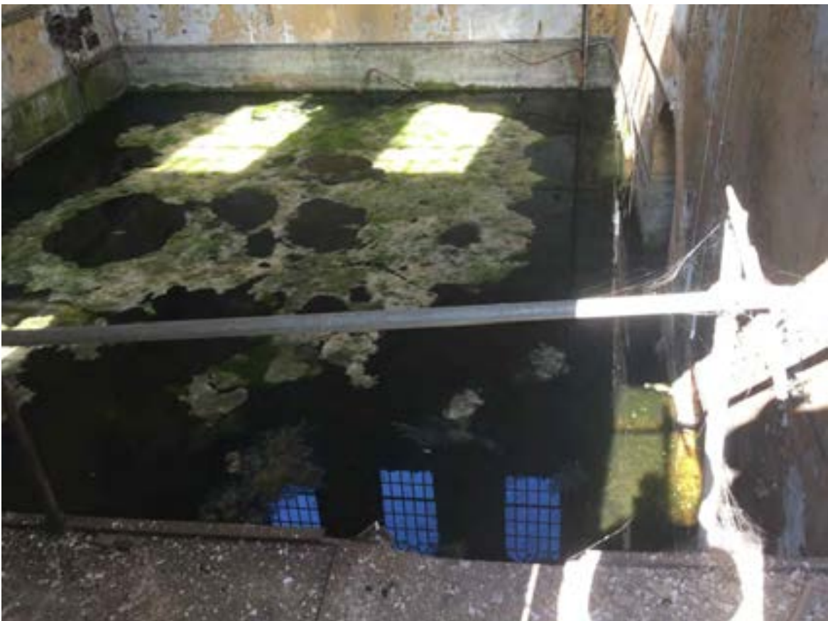
Plate 14: 2019 View of existing basement tank within Karslake building
