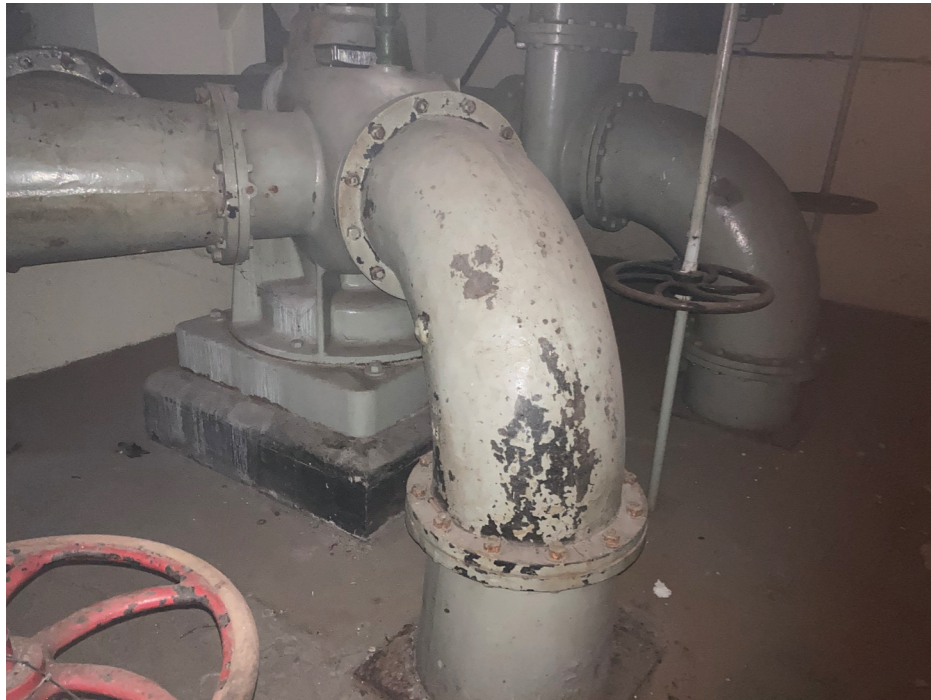
Figure 2 & 3: Pipework for 1932 Harland electric centrifugal pumps below ground floor level, accessed below ground floor level, Ruston & Ward Engine House. This is considered to be of low-medium significance.
