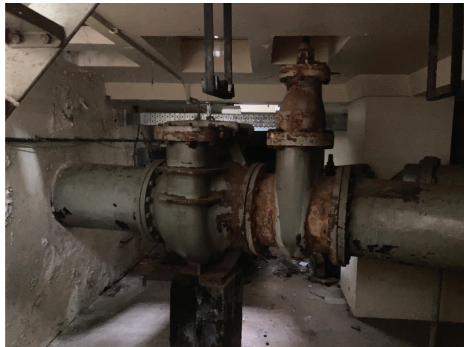
Figure 2 & 3: Pipework for 1932 Harland electric centrifugal pumps below ground floor level, accessed below ground floor level, Ruston & Ward Engine House. This is considered to be of low-medium significance.
