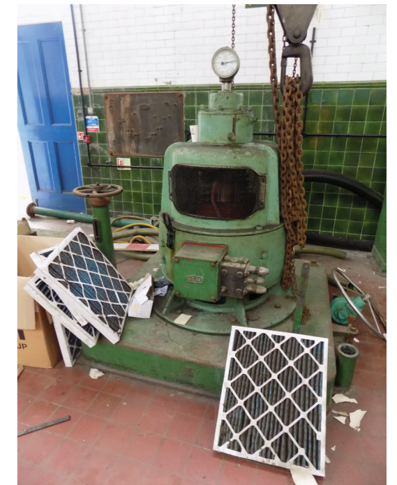
Figure 9: 1932 Harland DC motor, Ruston & Ward Engine House (low to medium significance)
