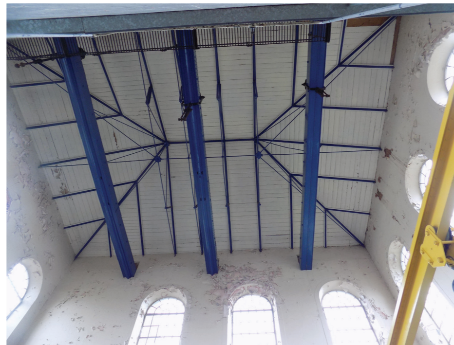
Figure 25: Primary wrought-iron roof, Ruston & Ward Engine House (medium significance)
