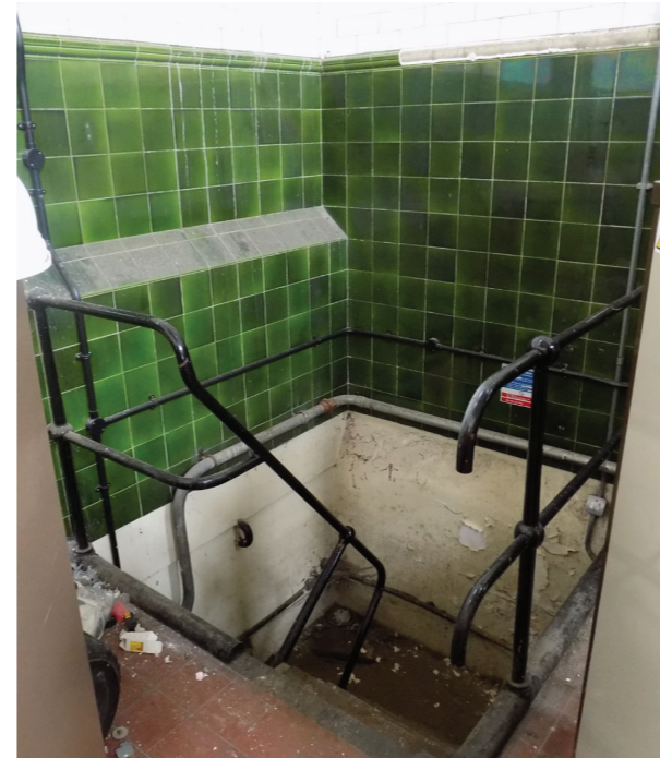
Figure 14: 1932 steps and handrails to basement, Ruston & Ward Engine House (low significance)
