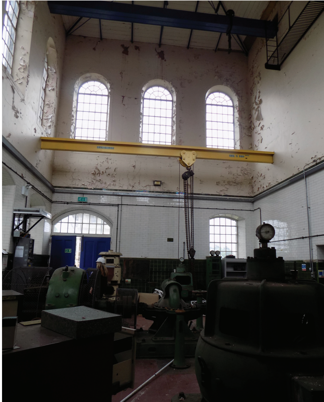
Figure 13: General view of interior of former Bull Engine House, showing 1932 Harland electrical pumping equipment and 1932 lifting beam, Ruston & Ward Engine House (low to medium significance)
