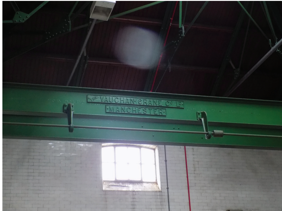
Figure 35: Maker's name on 1932 Vaughan gantry, former Ruston engine house (originally Sheffield's Boiler House) (medium to high significance)
