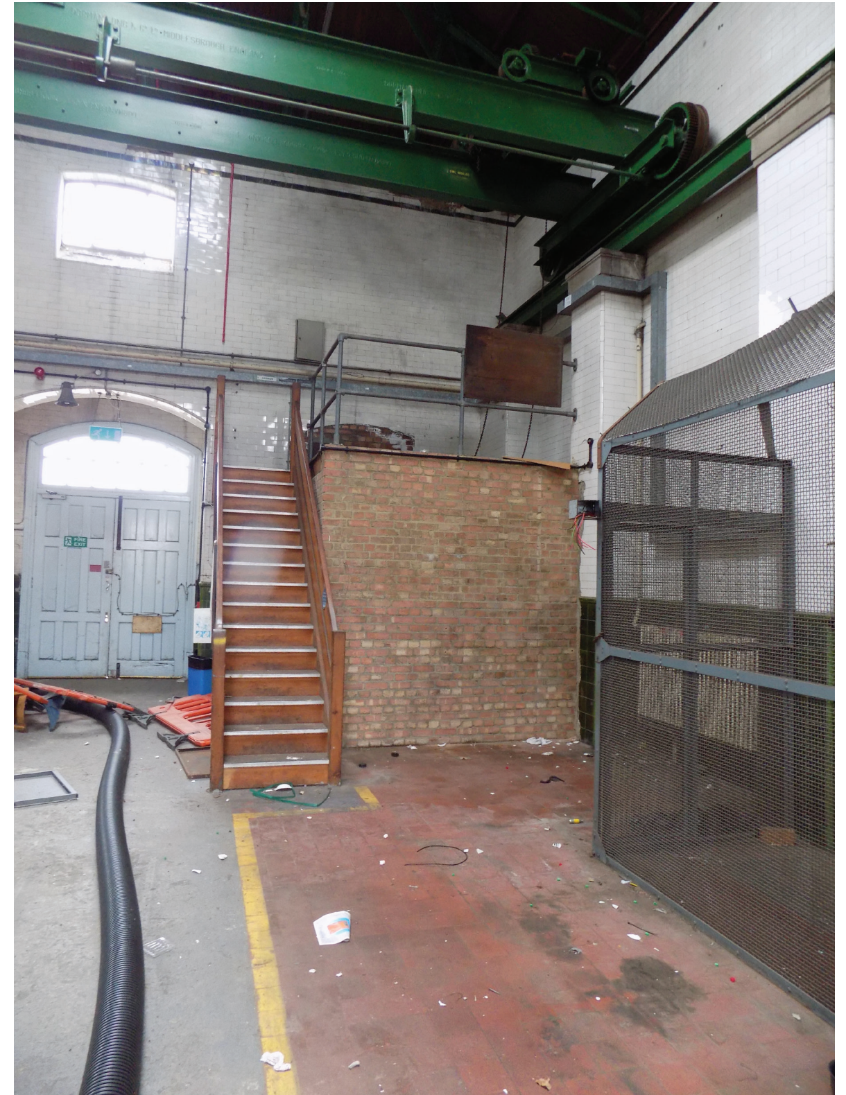
Figure 37: Brick-built later 20th-century enclosure in former Ruston engine house (originally Sheffield's Boiler House) (no significance)
