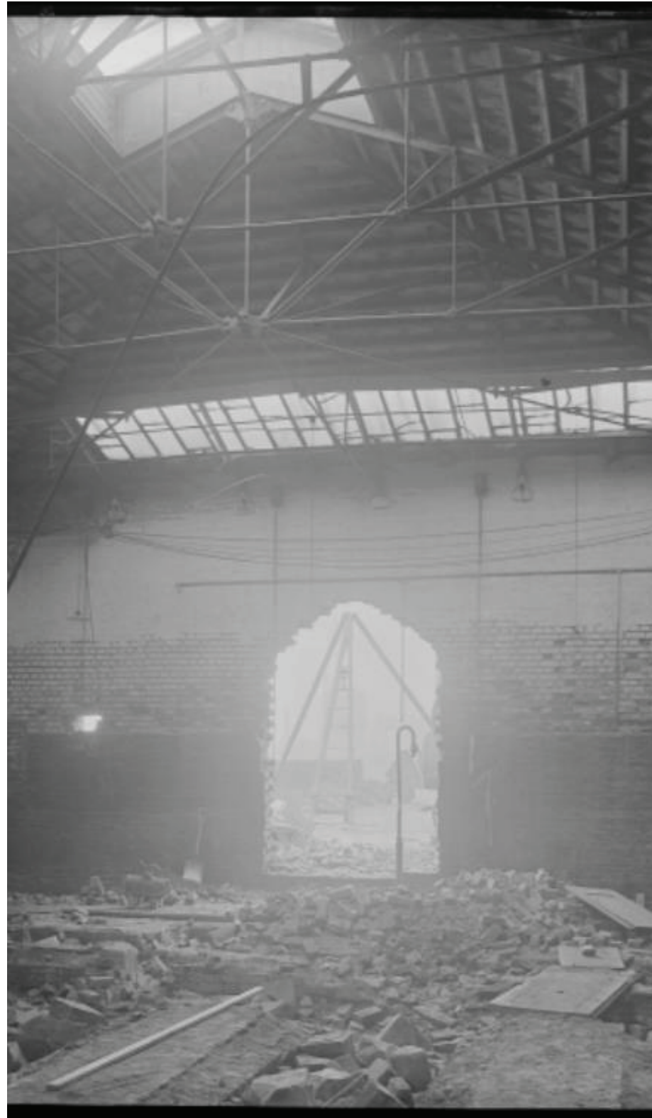
Figure 48: Ruston & Ward Former Ruston Engine House: Gutting of former Sheffield's boiler house in 1932, in preparation for adaptation to house Ruston & Hornsby diesel generator set
