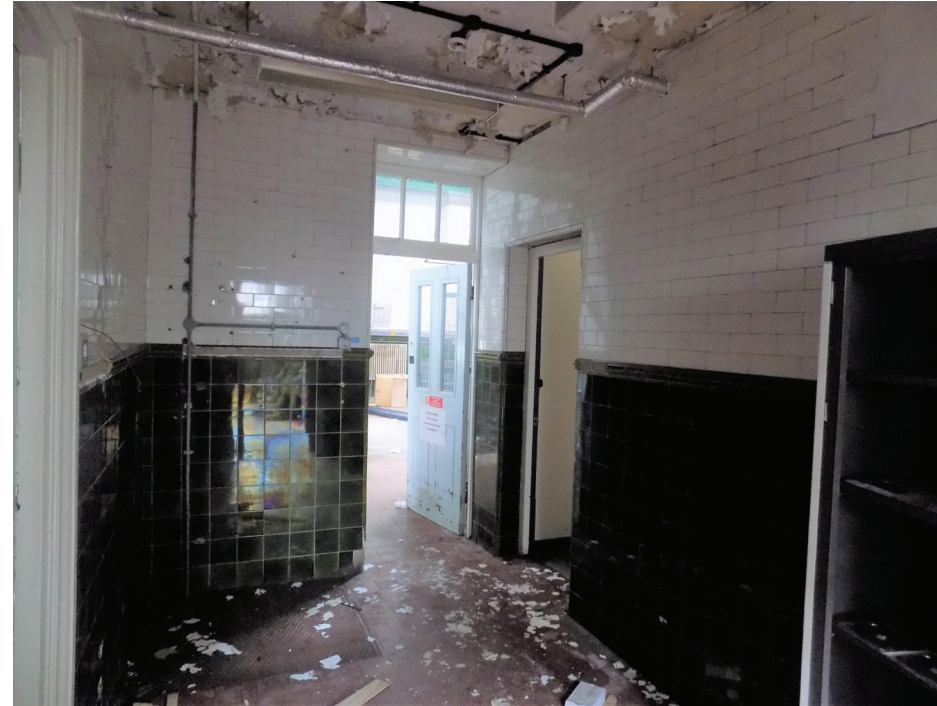
Figure 41: 1932 tiles and doors (medium significance)
