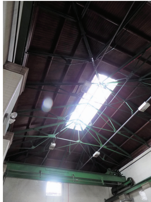
Figure 36: 1932 roof structure, former Ruston engine house (medium significance)
