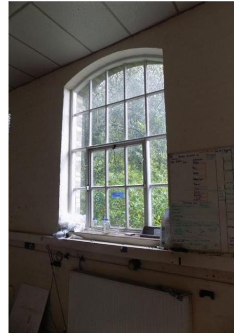
Figure 62: Replacement 1932 steel window, low significance.
