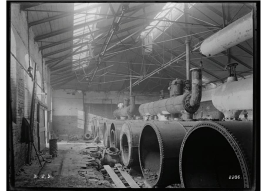
Figure 51B: Ruston Boiler House with boilers in course of removal showing the radial roof structure and former skylights, prior to the introduction of the north facing windows.
