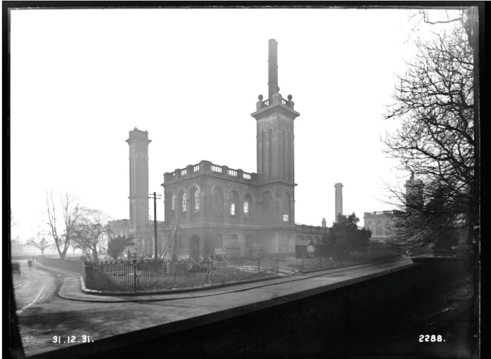
Figure 66: 1931 view of Ruston & Ward, immediately prior to removal of boilers and steam engines, showing pump head building in situ.
