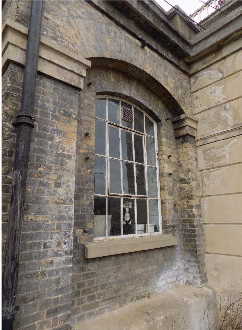
Figure 60: Brickwork detail and primary cast-iron window: Former Ruston Engine House (originally part Sheffield's Boiler House). Bolts of unknown purpose around window opening (medium significance)
