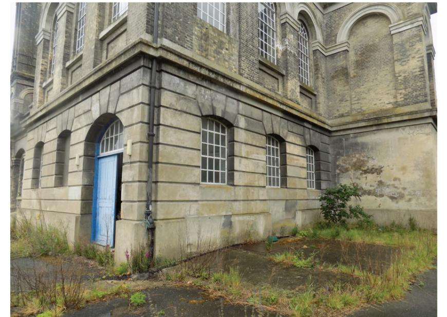
Figures 64 to 65: Exterior detail of Ruston & Ward Former Bull Engine House, showing cement repairs to base of pump head building.
