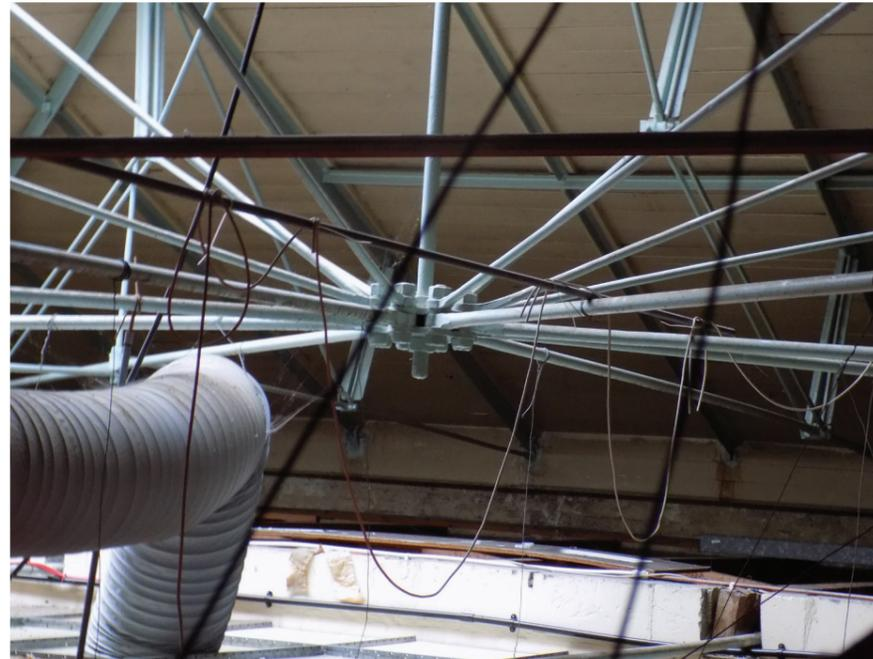
Figure 51A: Detail of primary wrought-iron roof (radial ties), Ruston & Ward Former Boiler House (medium significance)
