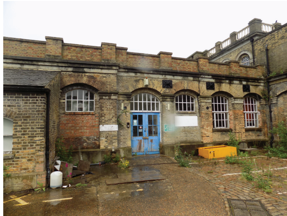
Figures 72 and 73: South side of the Former Boiler House, with course of coal railway visible as a concrete scar in the historic stone setts
