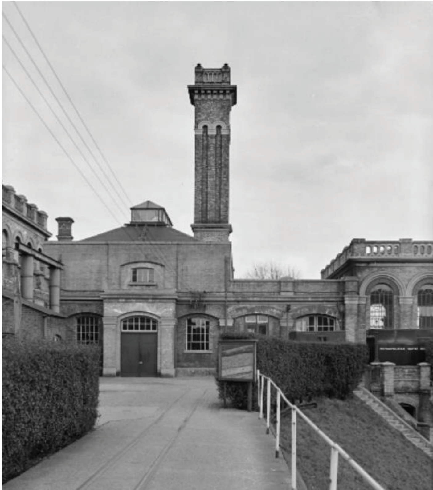
Figure 70: Post-1932 view of the west elevation of Former Ruston Engine House (originally part Sheffield's Boiler House), following raising of roof. Note railway for coal supply
