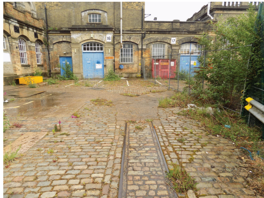
Figure 75: West elevation of Former Ruston Engine House (originally part Sheffield's Boiler House) showing fragment of railway for coal supply
