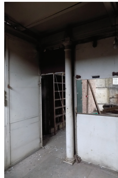
Figures 82 to 83: Middle mezzanine (cylinder) floor, with cast-iron columns and staircase (high significance - steel wall panels of no significance)
