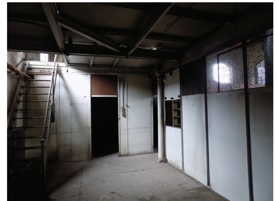
Figures 82 to 83: Middle mezzanine (cylinder) floor, with cast-iron columns and staircase (high significance - steel wall panels of no significance)
