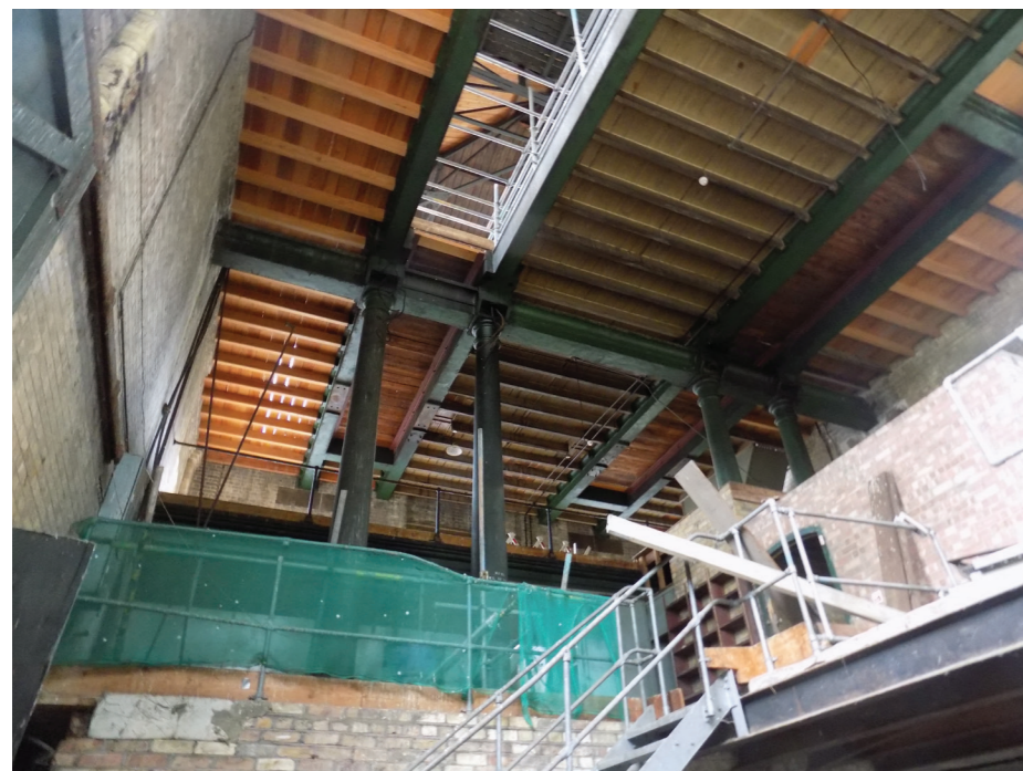
Figures 77 to 79: Surviving beam support structures (cast-iron columns and entablature), staircases and handrails, mezzanine and beam floor (spring beams and flooring) (all of high significance)
