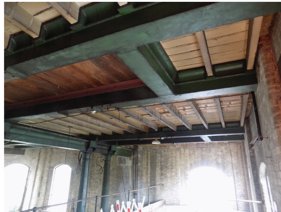
Figures 77 to 79: Surviving beam support structures (cast-iron columns and entablature), staircases and handrails, mezzanine and beam floor (spring beams and flooring) (all of high significance)
