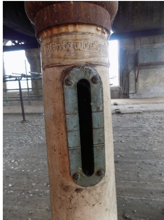
Figures 91 to 94: Cast-iron Blakesborough level indicators (two of, ex-situ) (high significance)
