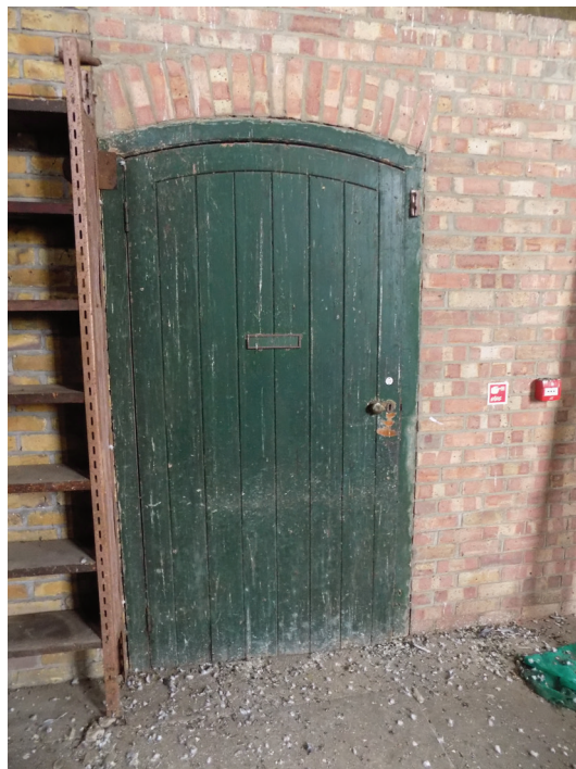
Figure 90: Re-located primary door on middle mezzanine (cylinder) floor (see Figure 81 above)
