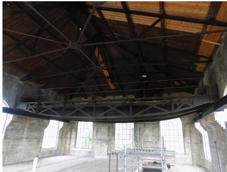
Figures 88 to 89: Beam loft floor and spring beams, gantry and cast-iron windows (all high significance)
