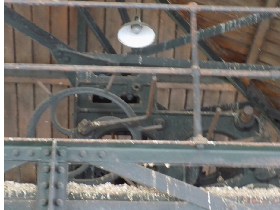
Figure 98: Hand-cranked gantry traveller (high significance)
