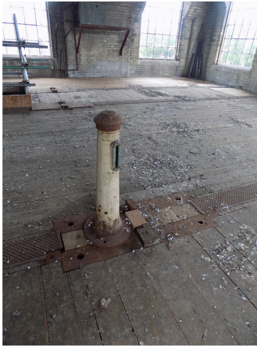
Figures 91 to 94: Cast-iron Blakesborough level indicators (two of, ex-situ) (high significance)
