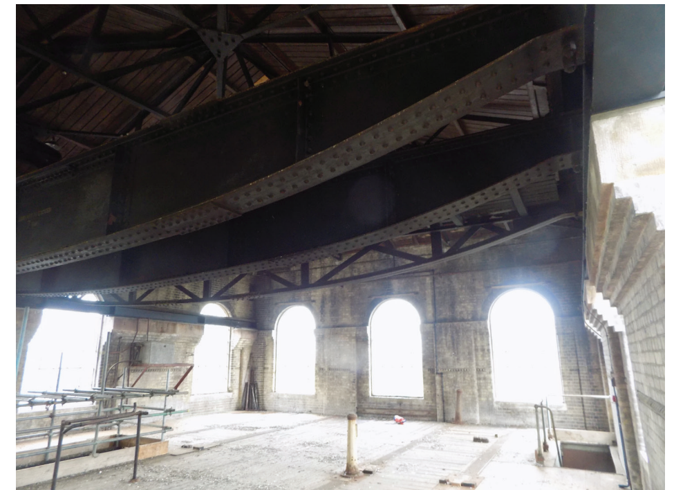
Figures 88 to 89: Beam loft floor and spring beams, gantry and cast-iron windows (all high significance)
