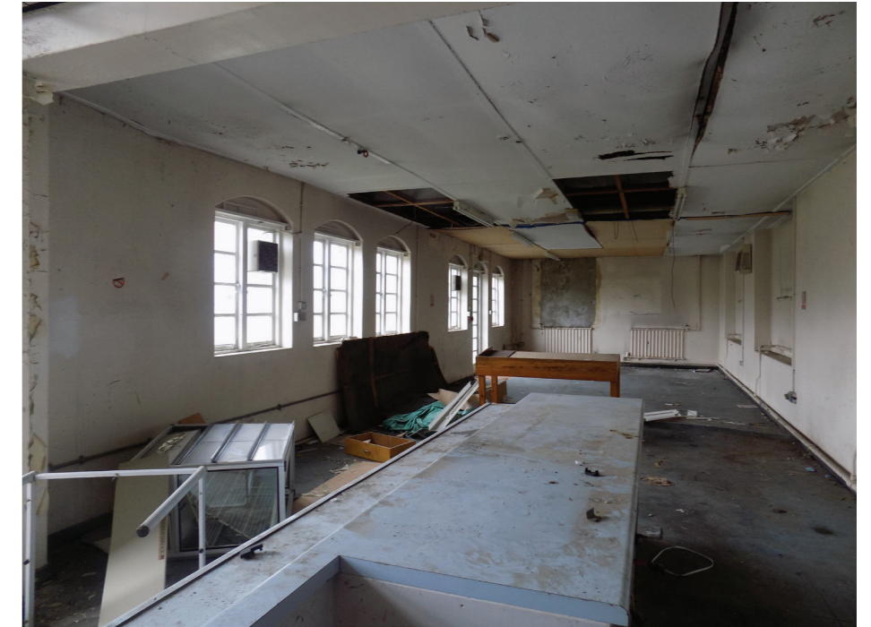
Figures 110: Primary timber casement windows in 19th-century extension south of Beam Engine House (medium significance)
