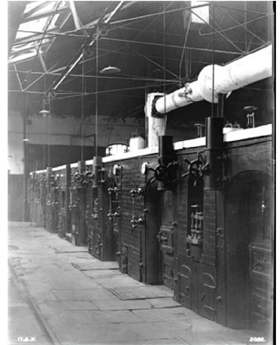
Figure 117: Karlsruhe Boiler House, prior to removal of boilers and conversion to offices.
