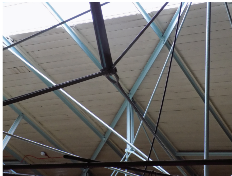
Figure 116: Detail of primary wrought-iron roof elements (medium significance)
