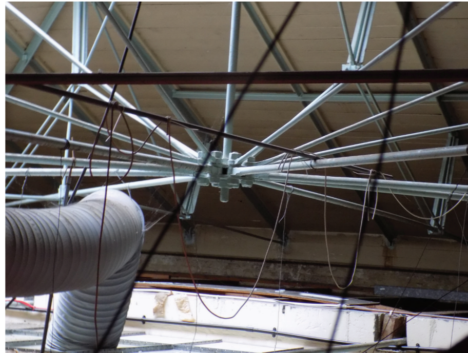
Figure 115: Boss of primary wrought-iron roof (radial ties) (medium significance)
