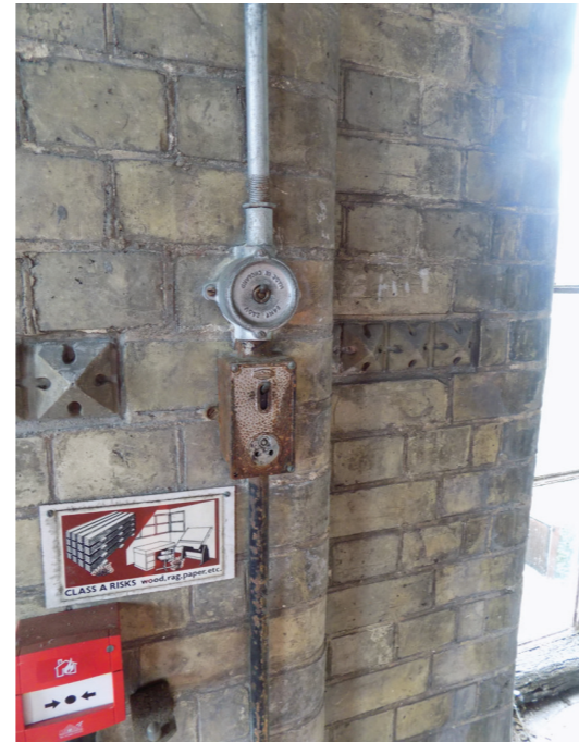
Figures 103: 1930s electrical conduits, switches and sockets (low significance)
