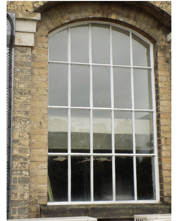
Figure 128: Karslake Boiler House, South Elevation. Cast Iron window, likely from 19thC.
