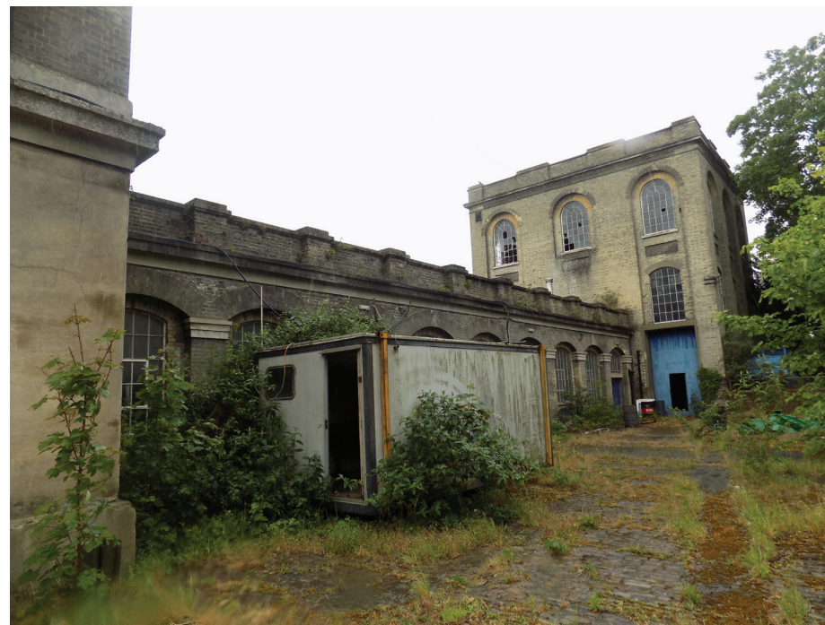
Figure 123: Former Boiler House set between the former Karslake Engine Houses.
