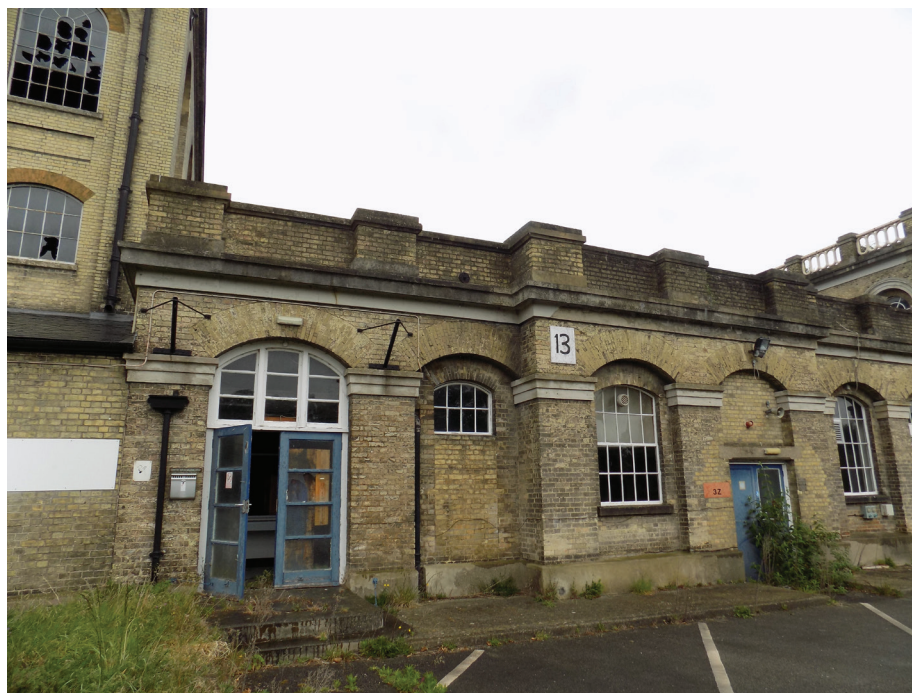
Figure 131: Karslake Boiler House, South Elevation showing bricked-in apertures and variety of window types.
