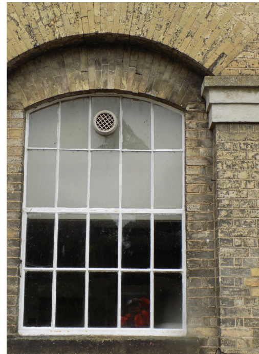
Figure 126: Karslake Boiler House, South Elevation. Cast Iron window, likely from 19thC.
