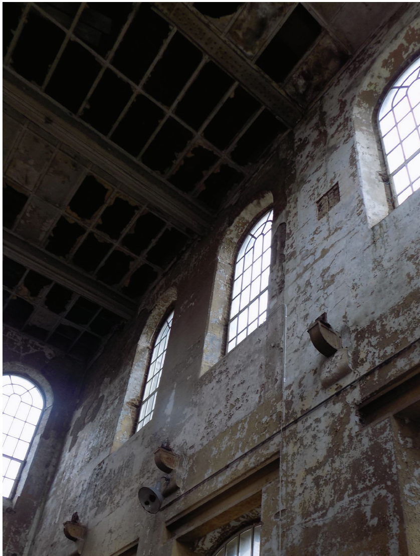
Figure 139: Interior detail showing corbels for engine lifting beams. These are the last remnants of the Bull Engine and therefore have relatively high level of interest.
