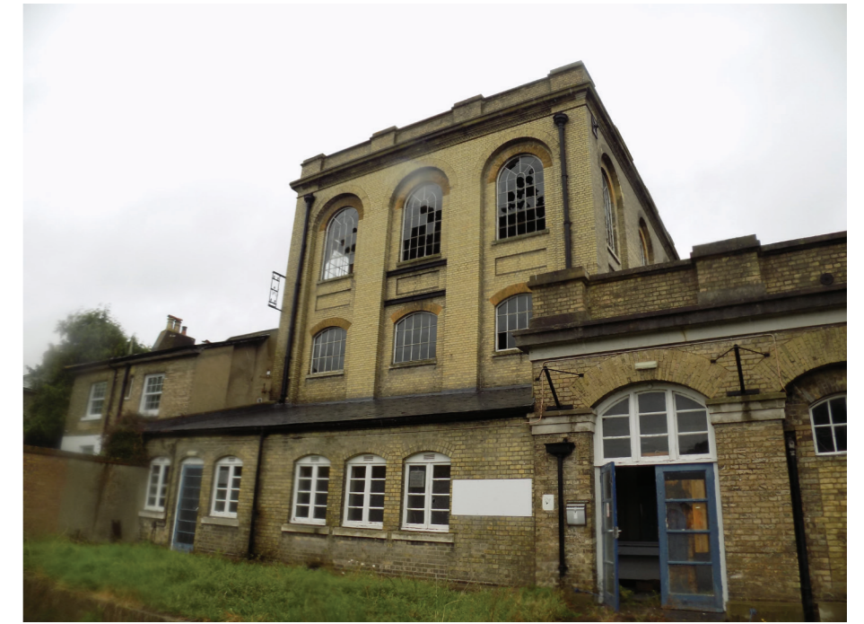
Figure 134: Karslake West Beam Engine Building showing Boiler House entry and lower storey welfare area with timber framed windows.
