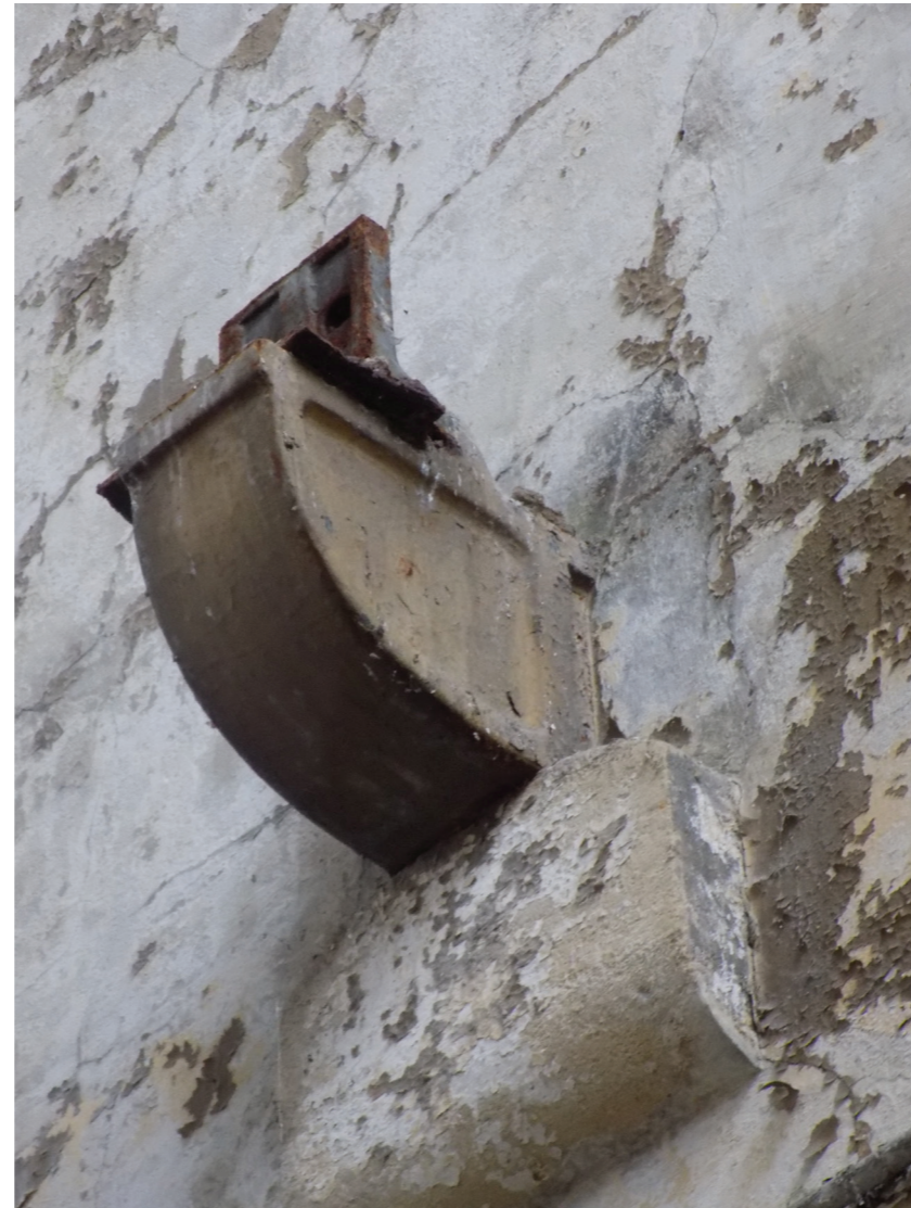
Figure 139: Interior detail showing corbels for engine lifting beams. These are the last remnants of the Bull Engine and therefore have relatively high level of interest.
