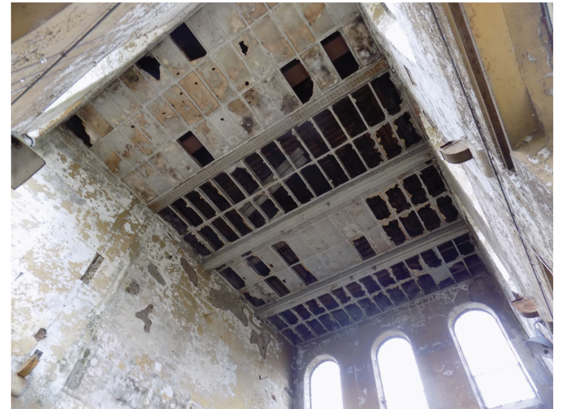
Figure 140: Later, inserted ceiling under sarked roof of low significance,
