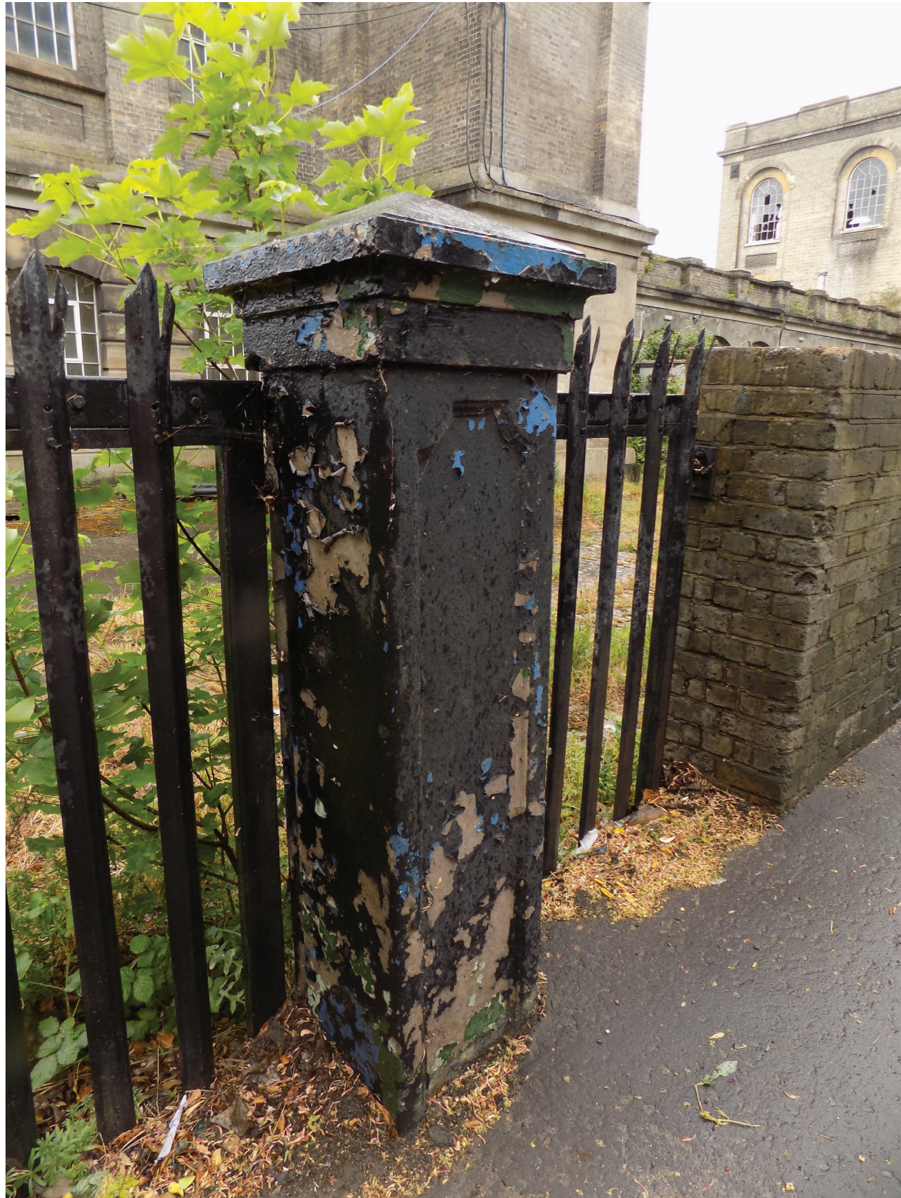
Figures 147-149: Painted, cast iron piers of medium - high heritage interest. Palisade fence considered to be intrusive and later brick wall considered to be of neutral heritage value. The smaller size of these piers demonstrates the historic hierarchy of circulation in to and out of the site.
