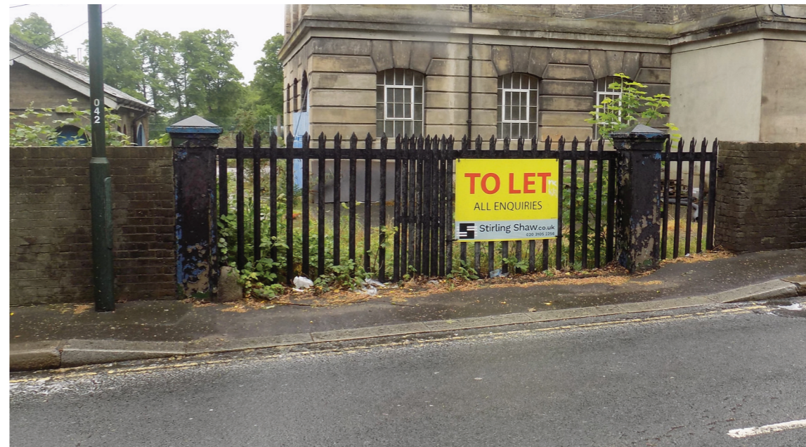
Figures 147-149: Painted, cast iron piers of medium - high heritage interest. Palisade fence considered to be intrusive and later brick wall considered to be of neutral heritage value. The smaller size of these piers demonstrates the historic hierarchy of circulation in to and out of the site.
