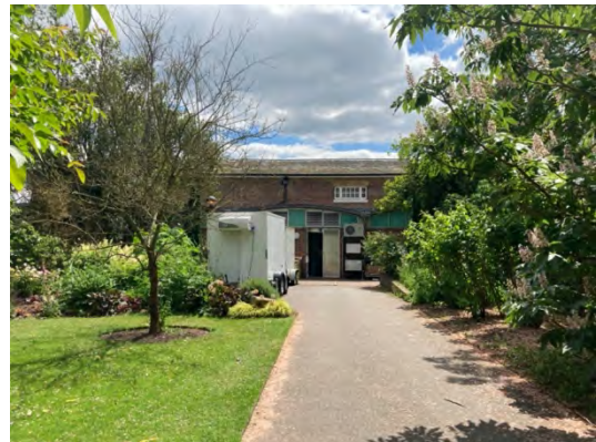
Fig 36 General view looking south towards the north extension
