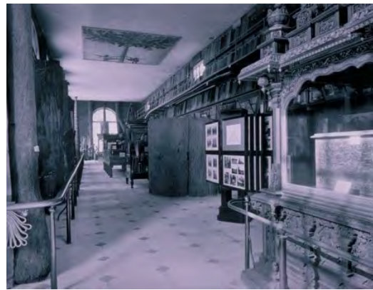
Fig 16 Interior of No.3 Timber Museum looking west
