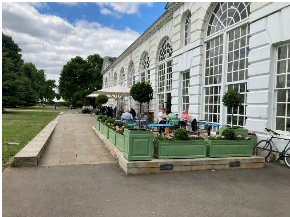
Fig 11 South terrace looking west
