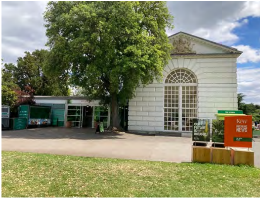
Fig 33 West elevation showing north extension
