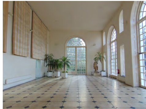
Fig 5 View looking east
