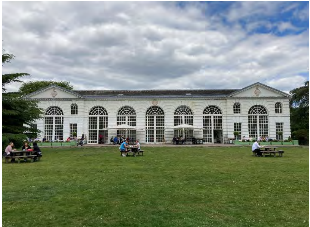
Fig 7 General of south elevation
