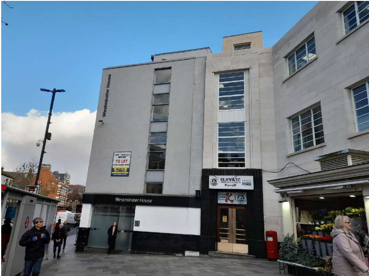
Plate 1: Westminster House. Looking to the north from the forecourt of Richmond Station.
