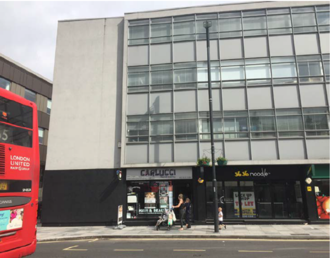
North West Corner
