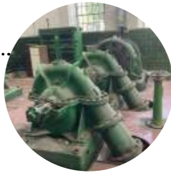
Item 4 Harland twin impellar electric centrifugal pump set Low to medium significance
