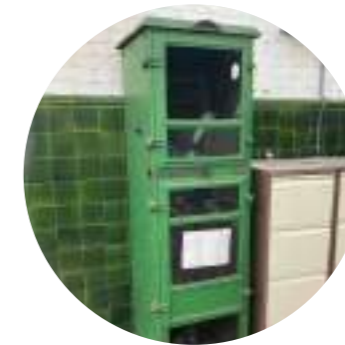
Item 7 Harland double leaf control cabinet for electric centrifugal pump Low to medium significance
