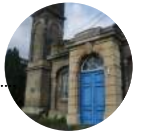
Prominent entry at junction utilised for the Workshop
