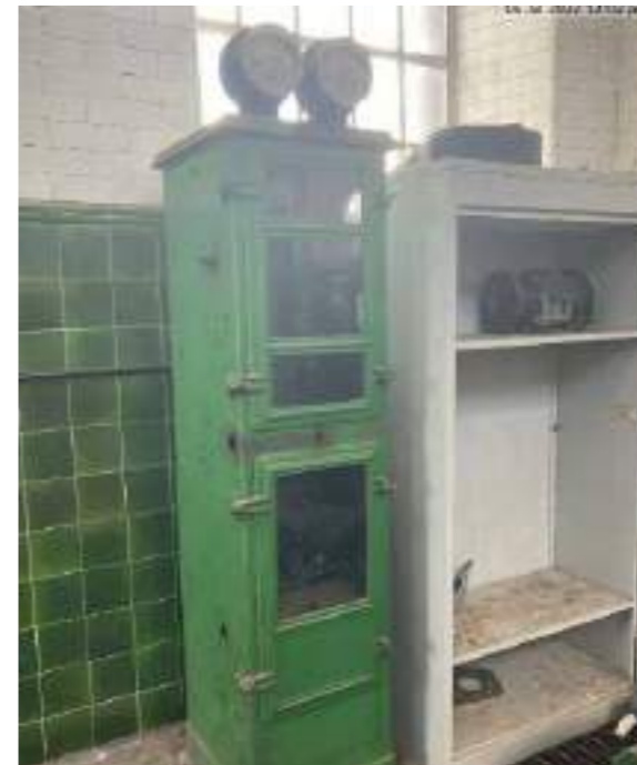
Harland control cabinet for electric centrifugal pump Date: 1932 Size: 0.5m x 0.5m Single Leaf Report comment: Low to medium significance
