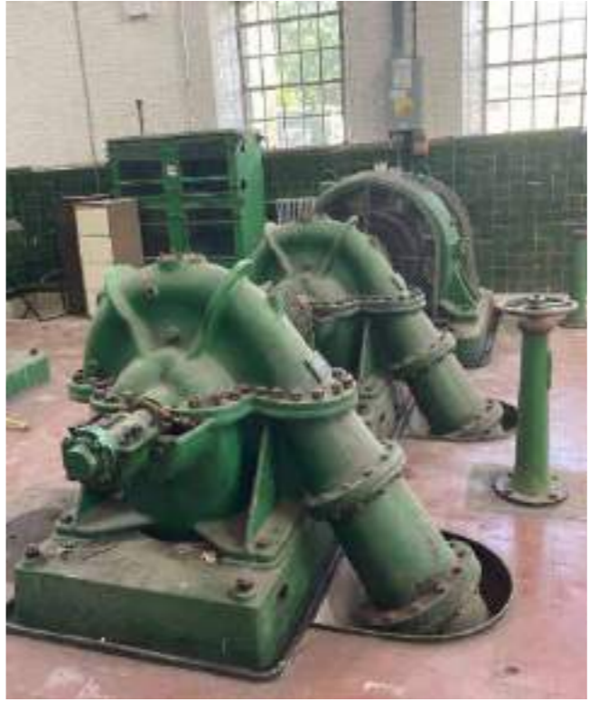
Harland twin impellar electric centifugal pump set Date: 1932 Size: 5.8m x 2.5m Report comment: Low to medium significance
