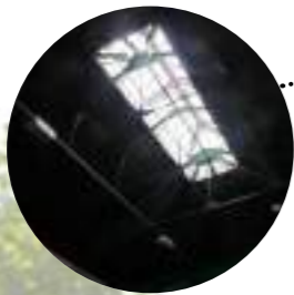
Roof trusses & glazed roof light retained
