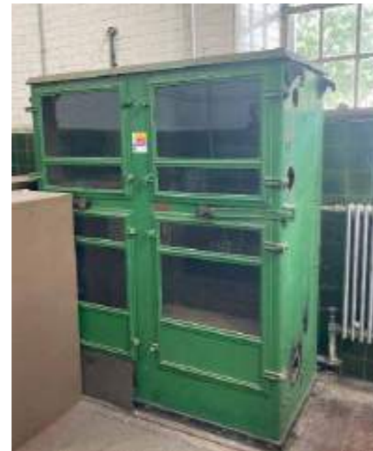
Harland control cabinet for electric centrifugal pump Date: 1932 Size: 0.9m x 1.7m Double leaf. Report comment: Low to medium significance
