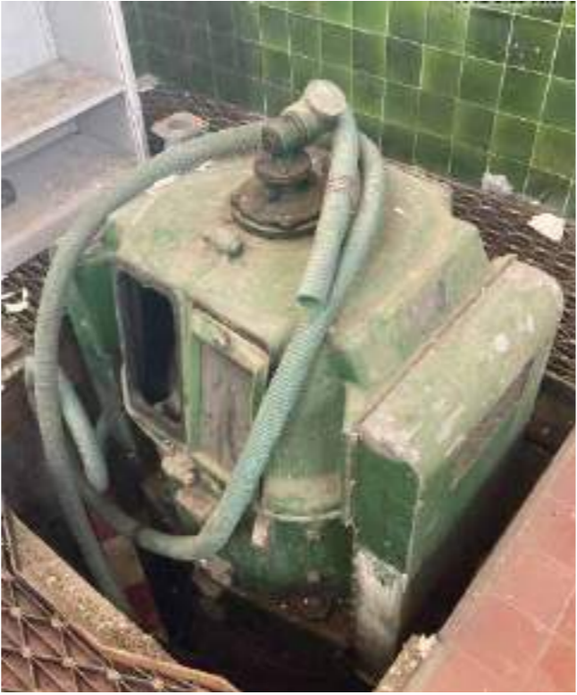
Harland DC Motor Date: 1932 Size: 1.6m x 1.6m x 3 (Recessed) Report comment: Low to medium significance
