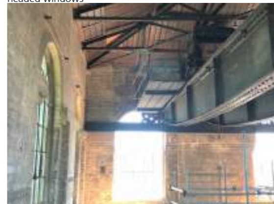
Top level 3 of the western block, 'The Beam,' with a large steel gantry crane at the right
