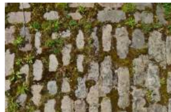
Existing cobblestones within the landscape - to be retained as part of the landscape proposal
