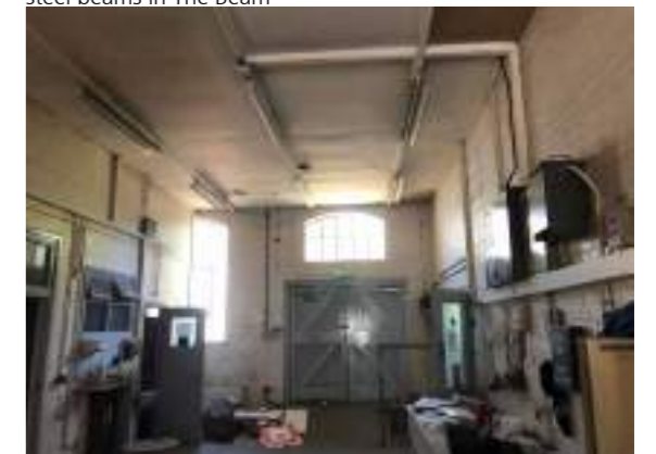
The central block has been subdivided with concrete block and aluminium partitions in the late-twentieth century
