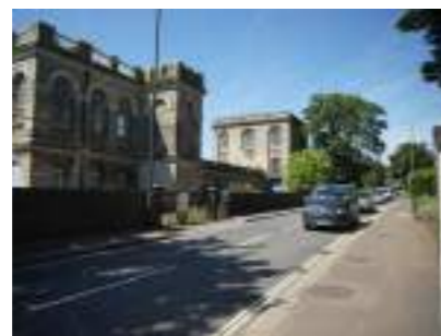
Site edges (-) Upper Sunbury Rd is busy & intersection with Lower Sunbury Rd / vehicle traffic noise
