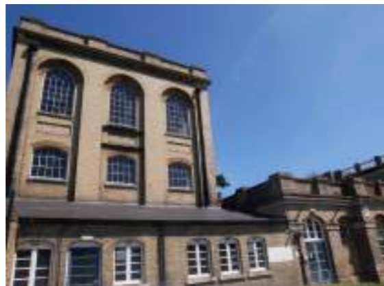
Southern view to the western block with the single storey lean-to extension at the front
