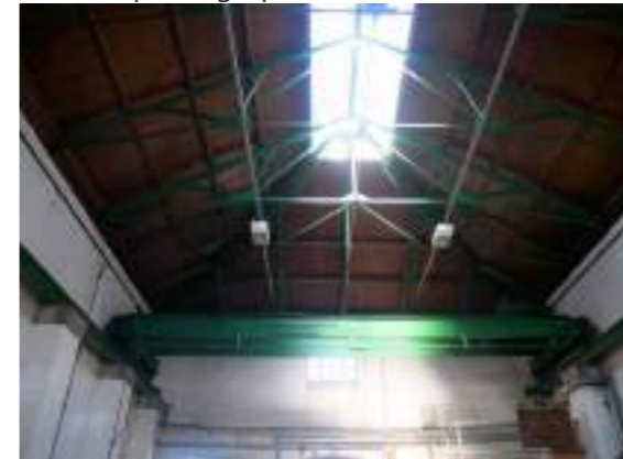
Workshop interior with glazed roof light in the southeast part of the building
