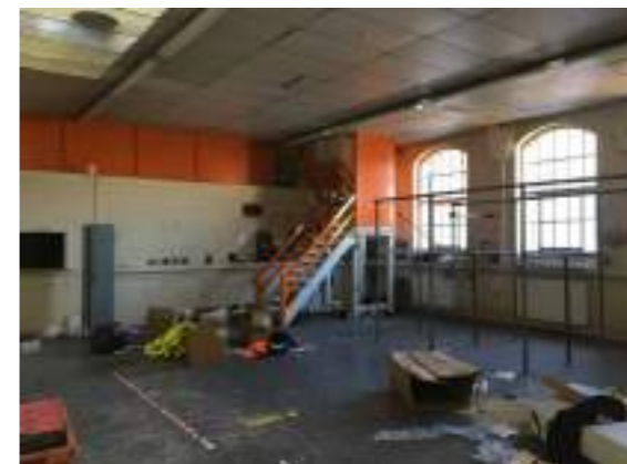
20th century alterations to the interior of Ruston & Ward building
