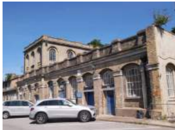
Southern facade of the single storey central block
