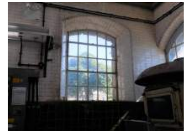
Ceramic glazed tiles to the window reveals of the pump house
