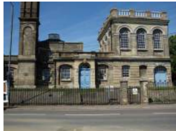
Pedestrian entry off of Lower Sunbury Rd
