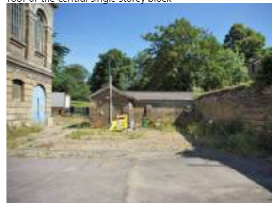
Southern view of the small Storehouse building, with Karslake to the left
