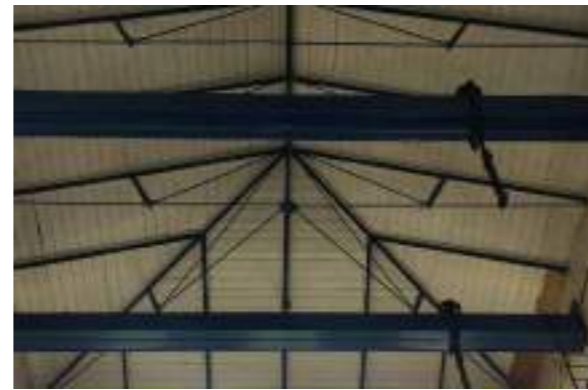
Large steel beams & composite wrought iron trusses
