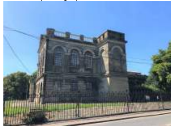
Large pump house on the northeast corner
