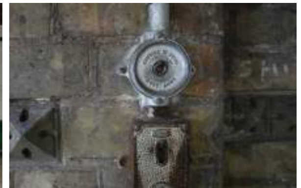
Western pump house in Karslake retains the most original features
