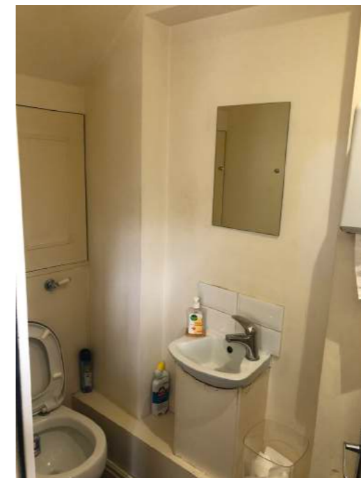
Existing ground floor WC
