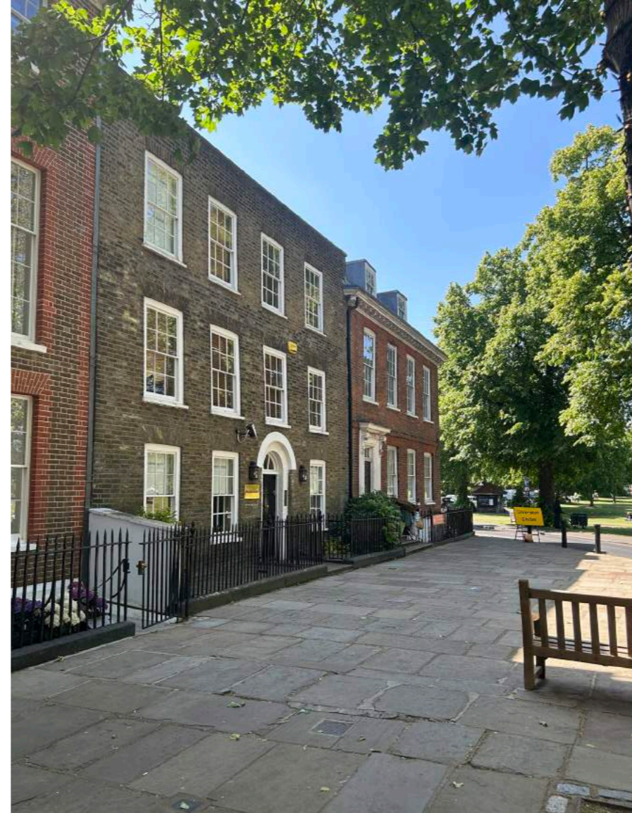
31 The Green looking from the Prince of Wales pub
