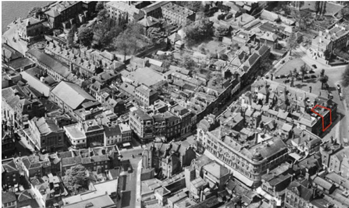
Aerial Photo (c)Britain from Above - Image shows 31 The Green with a flat roof. Image Ref: EPW031989 dated 1928. (curtilage in red)
