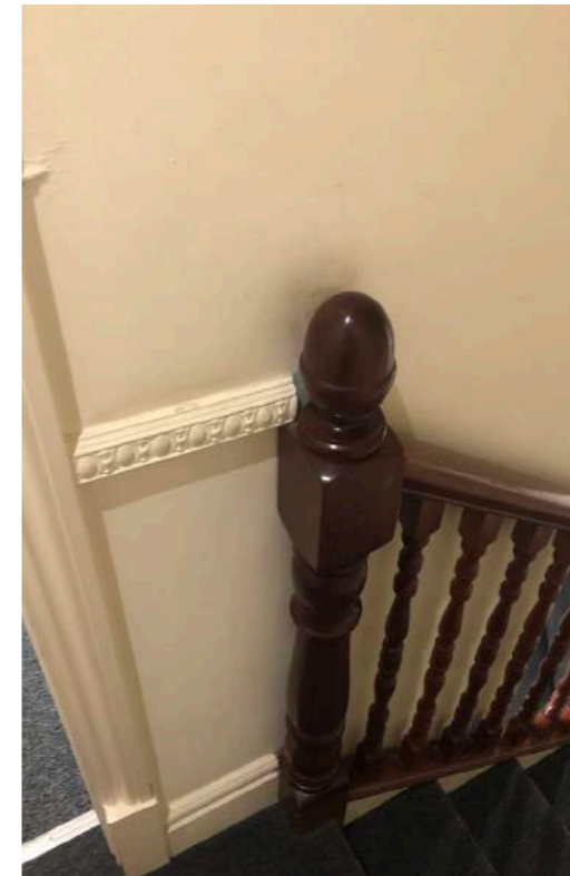
Existing second floor stair
