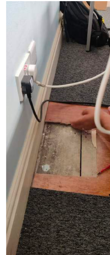
1st and 2nd floors are have 20C timber boards laid over the joists. There are no signs of previous partitions between windows
