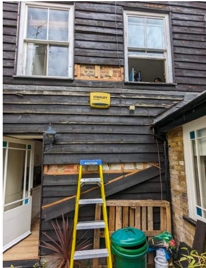
Existing rear elevation - masonry behind cladding (ground and 1st floor)
