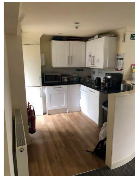
Existing kitchenette to be removed
