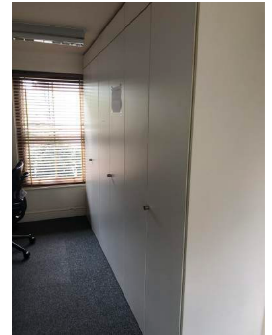
Existing cabinetry to be removed
