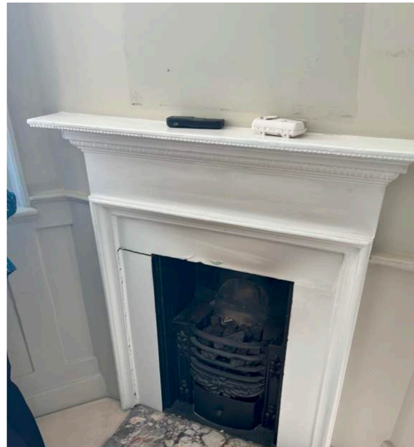
Corner Fire Places and all fires on the second floor - proposed surrounds to match the above image which is a period piece in a nearby listed building that would be followed in design. It also features a small Georgian hob grate.
