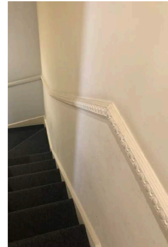
Existing second floor stair
