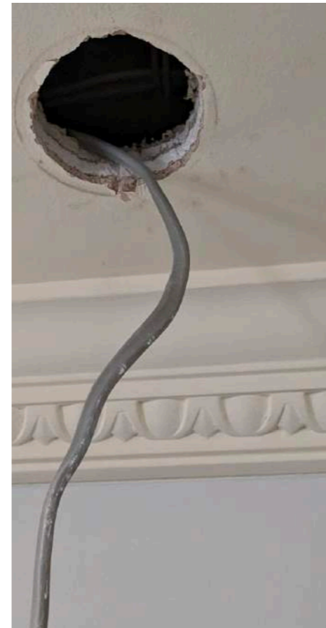
All existing ceilings are lined with modern plasterboard
