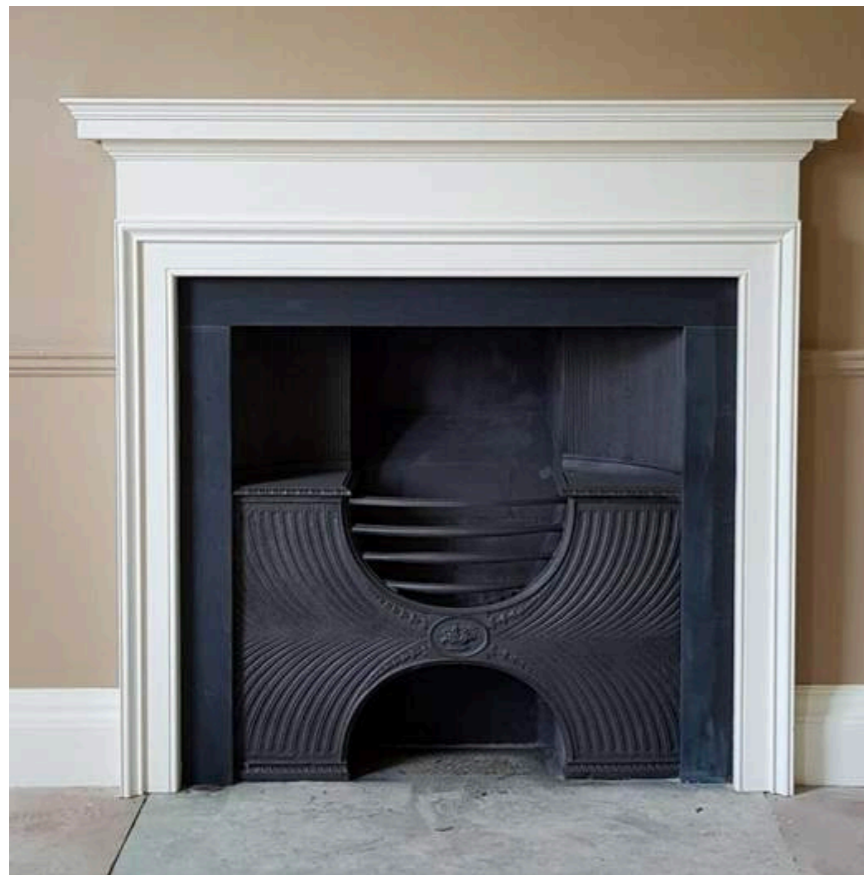
Fireplaces in principal rooms on ground and first floor to be larger and more ornate as per the image above.
