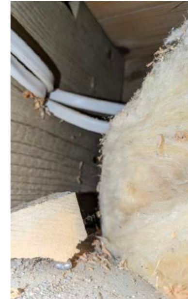
First and second floor construction - views through light fitting apertures. Modern plasterboard attached to base of joists, overlaid with timber boards still light in colour on top of square edged joists
