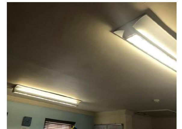
Existing light fittings to be removed
