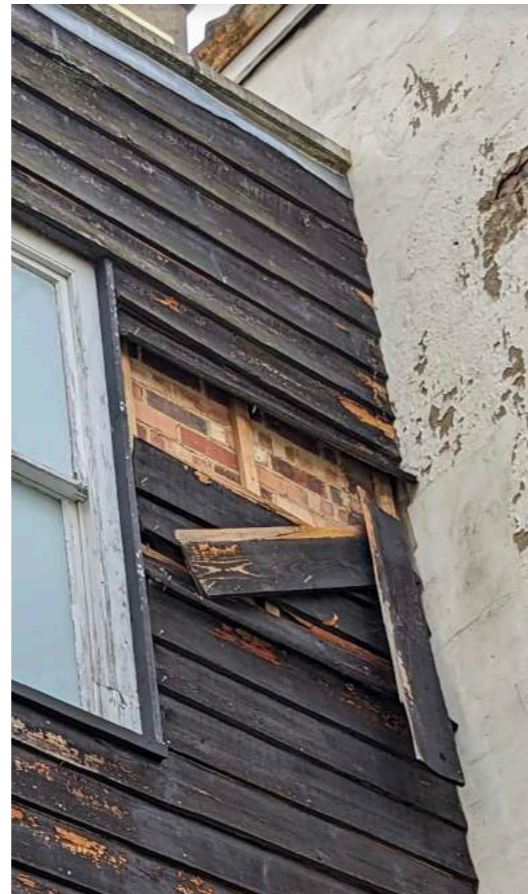
Existing rear elevation - masonry behind cladding (2nd floor)
