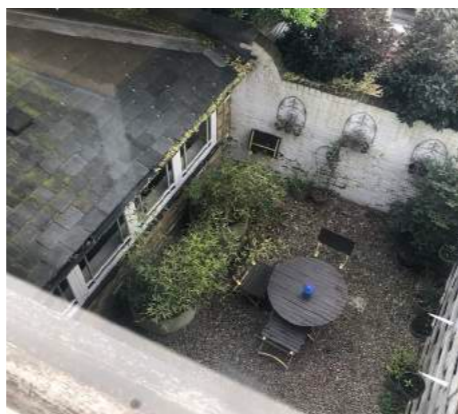
Existing rear courtyard - view from upper floor window
