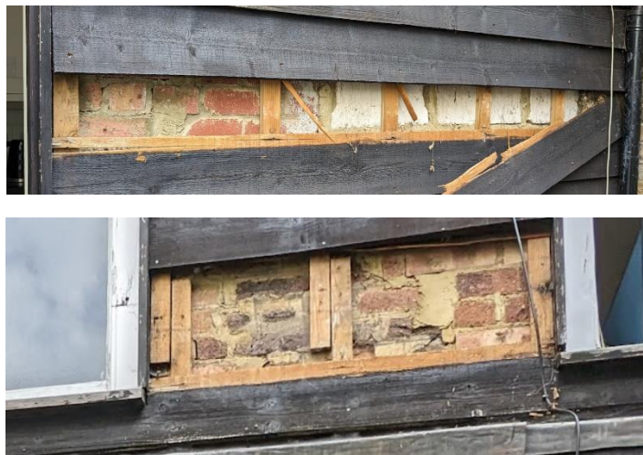
Figures 13 and 14: Existing rear elevation during the investigation works 2023 © MJA
