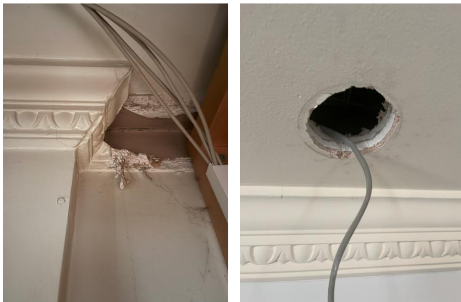
Figures 24 and 25: Modern cornices and plasterboard ceilings present at 31 The Green
