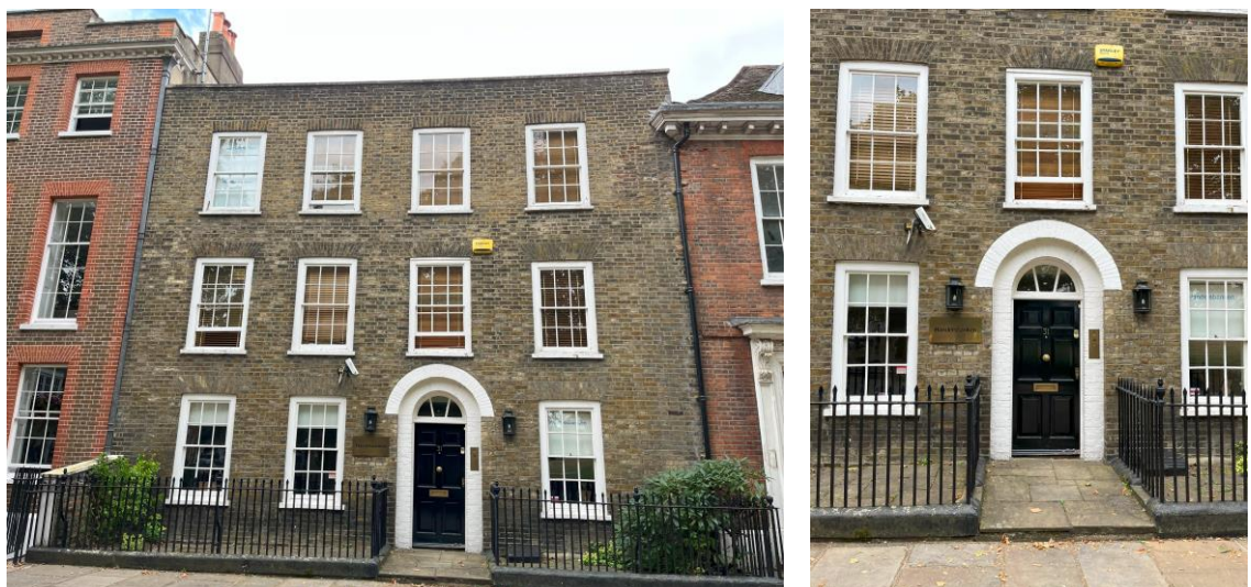
Figures 16 and 17: Front elevation and area railings of 31 The Green
