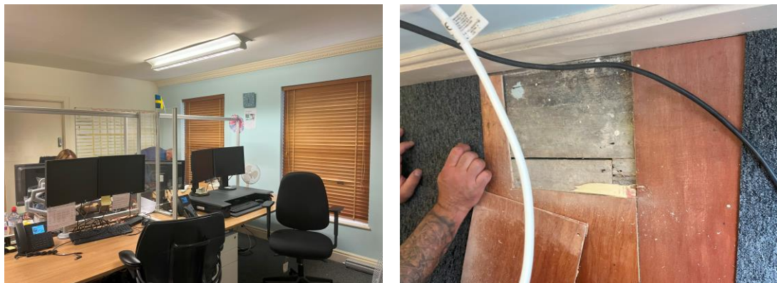
Figures 28 and 29: Second floor main office (left) and 20 th century floorboards present beneath the modern floor at second floor level
