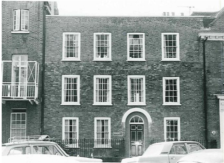
Figure 12: 1971 photograph of 31 The Green showing the very clear difference in brickwork between the original 18 th century brick and different brick to the upper floor
