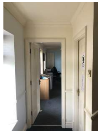
Existing wall in to office
