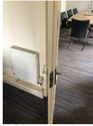
Existing double door to be retained and restored
