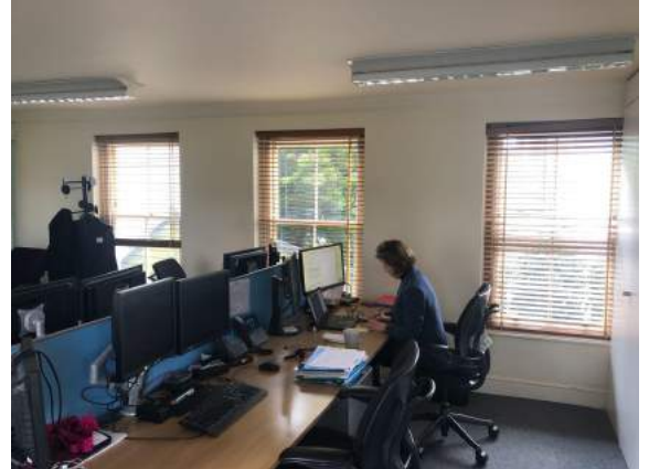
Existing windows - East side
