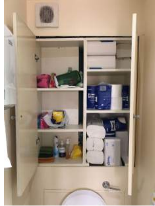
Existing cupboard behind WC
