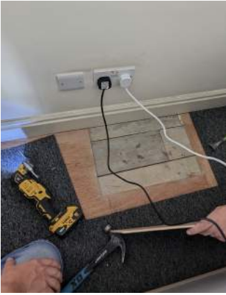
Existing 20C floorboards beneath carpeting to be retained on upper floors, re-used to infill the change in stair position.
