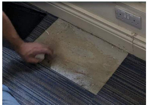
Existing concrete slab across the ground floor
