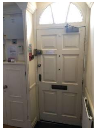
Existing entrance door
