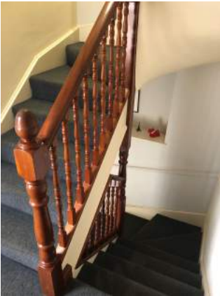
Existing modern staircase and handrail
