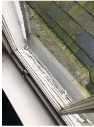
Existing condition of sash window
