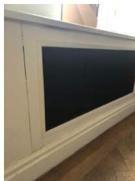
Existing timber radiator cover
