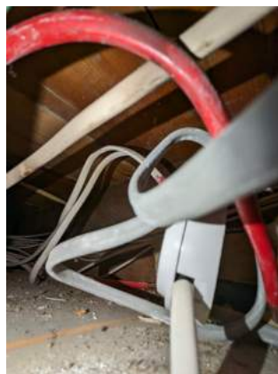
Existing floor buildup
