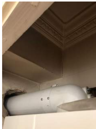
Existing boiler flue
