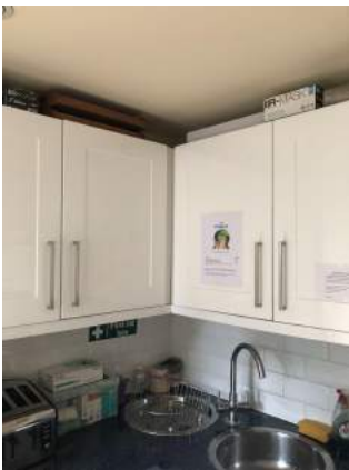
Existing kitchenette joinery
