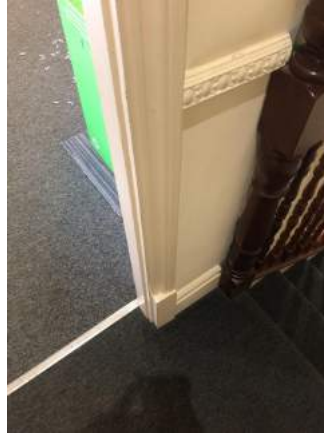
Existing skirting board and Dado
