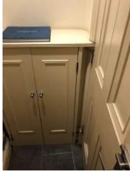
Existing cupboard opposite WC
