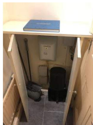
Existing floor tiles
