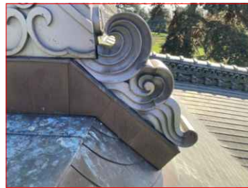
Ridge element slipping slightly
