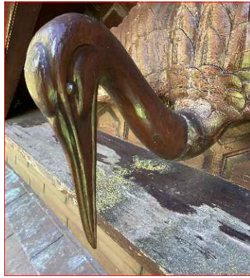
Paint flaking to sculpture
