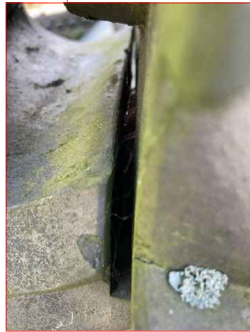
Ridge element slipping slightly
