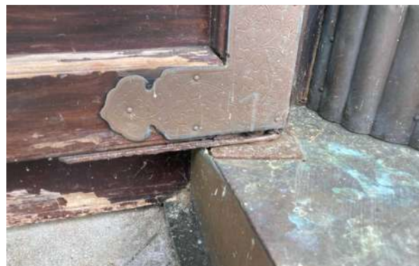
Fig. 7 Degraded decoration on the door on the south elevation
