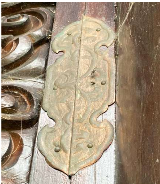
Fig. 10 Copper repousse detail evidence of mirror polish finish on east elevation
