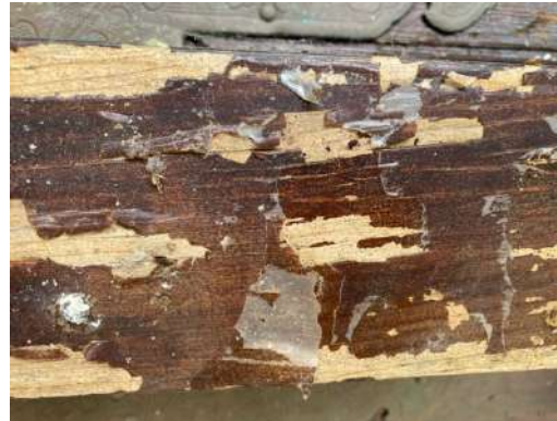
Fig. 5 Degraded decoration on the door on the South elevation
