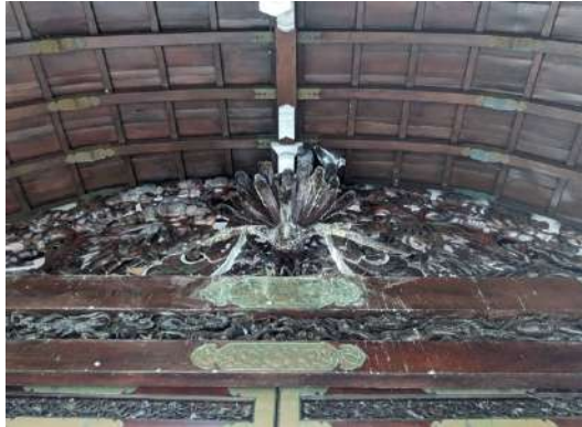
Fig. 4 Guano on high level carvings on the North elevation
