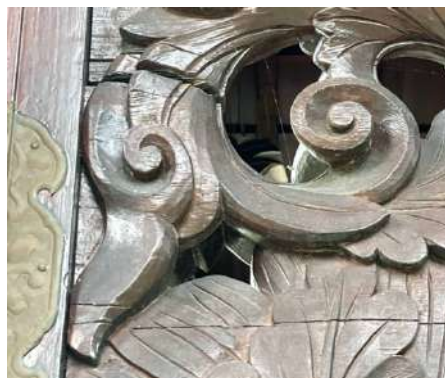
Fig. 6 Split in carving on east elevation
