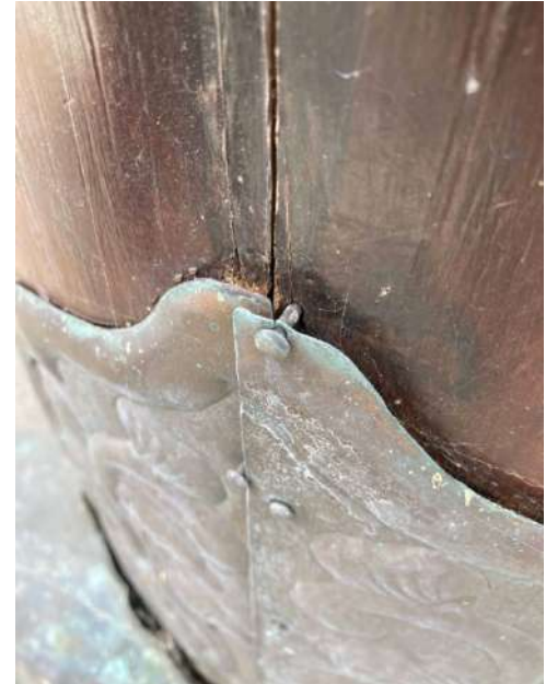
Fig. 9 Copper repousse detail coming away from post
