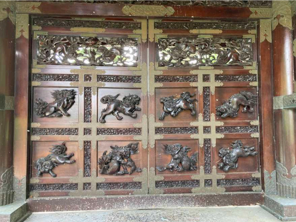
Fig. 17 Doors on north elevations
