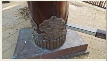
after 100mm of space, as the probe oscillates and then deflects producing anomalous readings. However, in the case of graph 9, the probe continued through nearly 200mm of space, indicating the round posts are almost certainly hollow.
