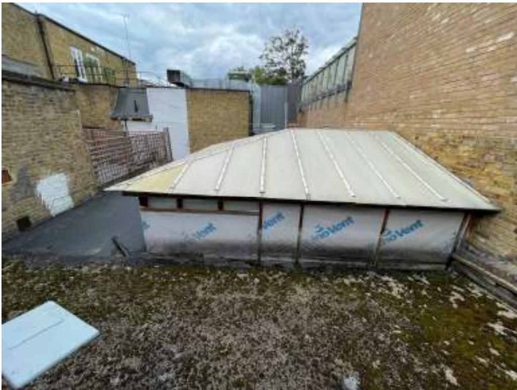
No. 3 Duke Street, Richmond Roof – View from front to rear
