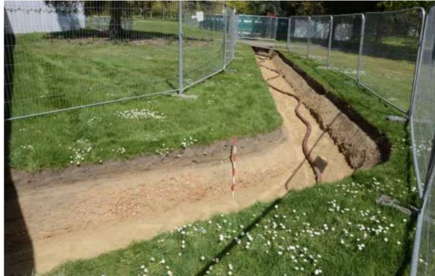
Fig.338: Service trench exiting the southeast of the main Temperate House compound, facing NNE, 0.8m scale Plate 21 - Service trench to the south of Site J from the south looking north-northeast (Aaronson 2018)
