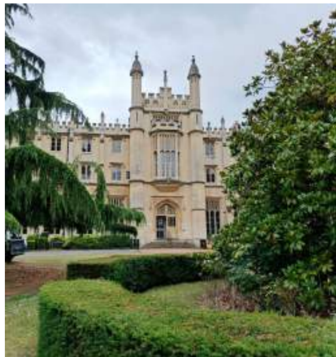
Photograph of main entrance showing stepped approach
