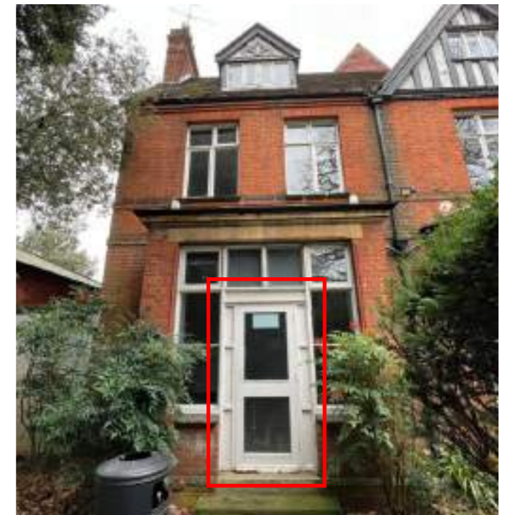
Photograph of door to be replaced
