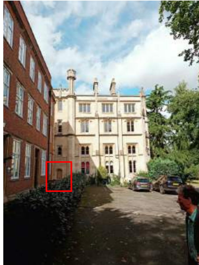
Location of entrance door to be altered
