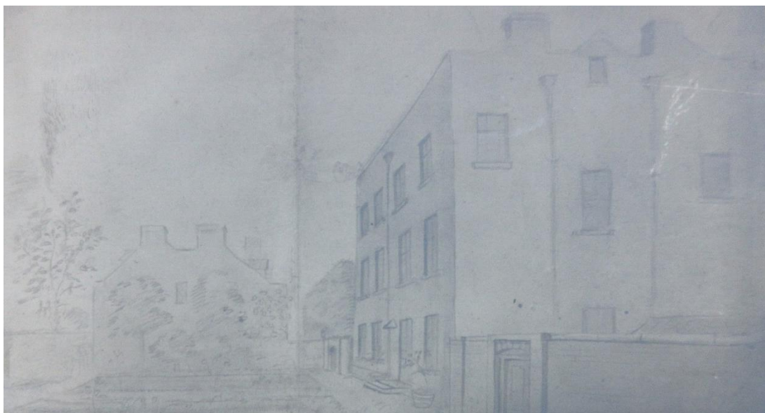
Figure 20: A sketch of the house owned by Captain Grose who lived on Richmond Hill – believed to be within the subject site.
