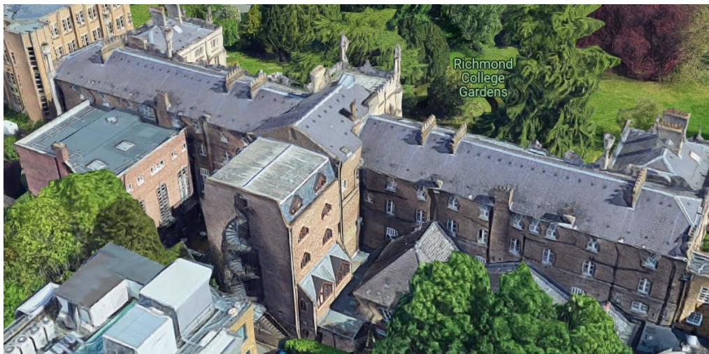
Figure 24: Aerial view looking eastward, showing rear extensions A, B, C, D & E. (Google, 2023.)
