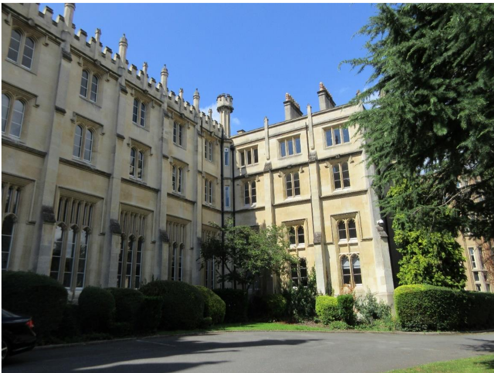
Figure 12: Front (north-east) elevation of central part, and south-east elevation of north wing, of the principal building.
