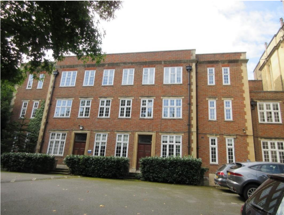
Figure 7 (left): Front (north-east) elevation of George House.
