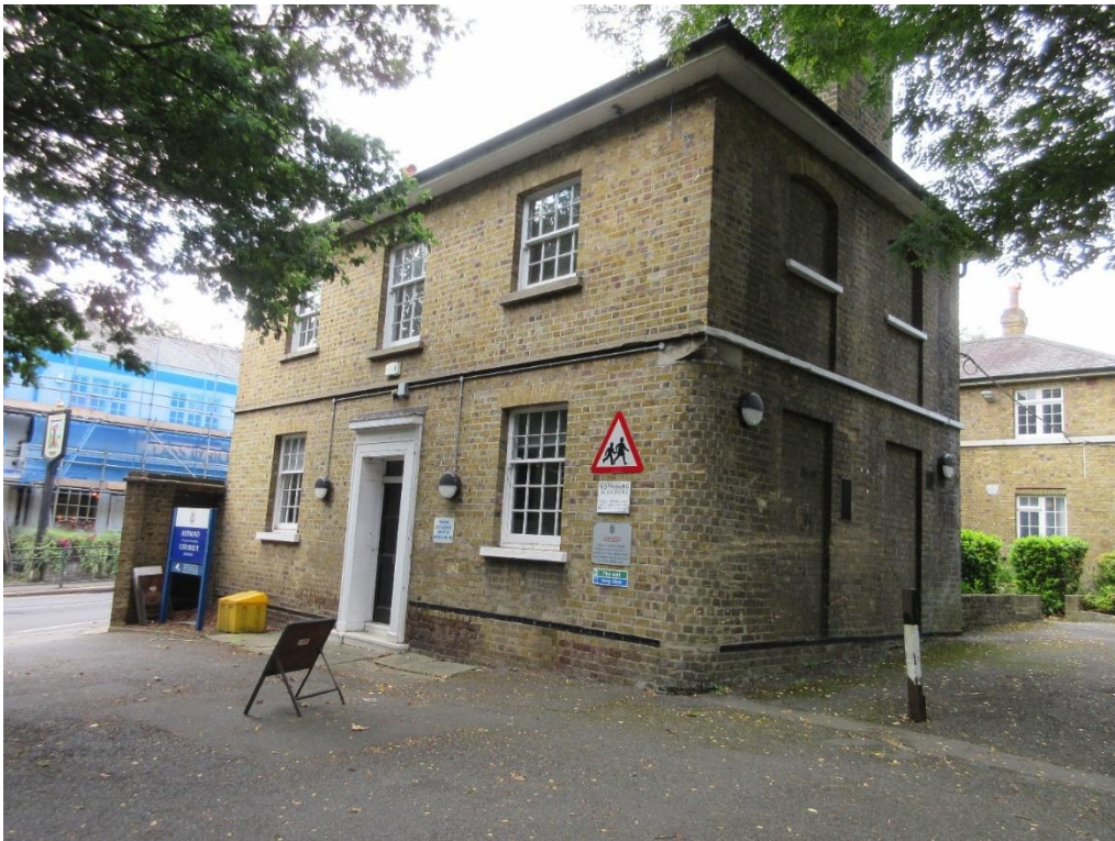
Figure 29: Front (north-east) elevation and side (north-west) of Lower Cottage in the foreground, and front (north-east) elevation of Upper Cottage to the right. (Lass O'Richmond Hill public house (locally listed) is on the other side of the road.)
