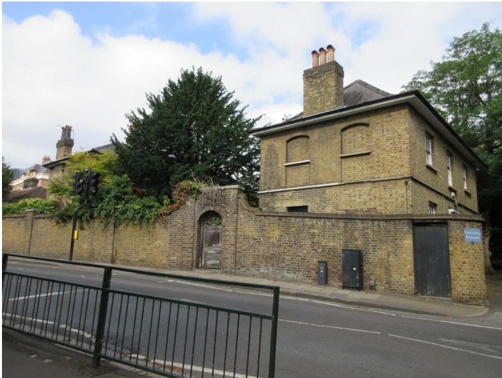
Figure 27: Side (south-east elevations) of Upper and Lower Cottages addressing Queen's Road, and the front boundary.
