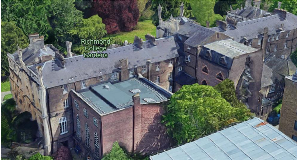
Figure 23: Aerial view looking south-eastward, showing rear extensions A and B. (Google, 2023.)
