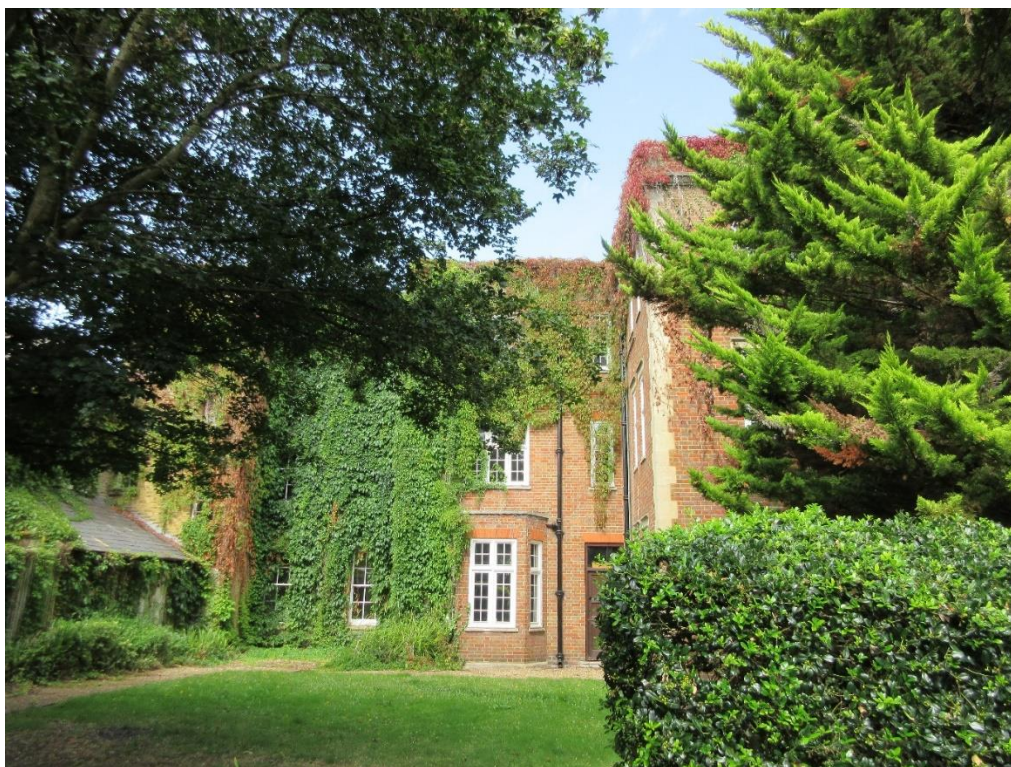
Figure 9: Side (south-east) elevation of George House.
