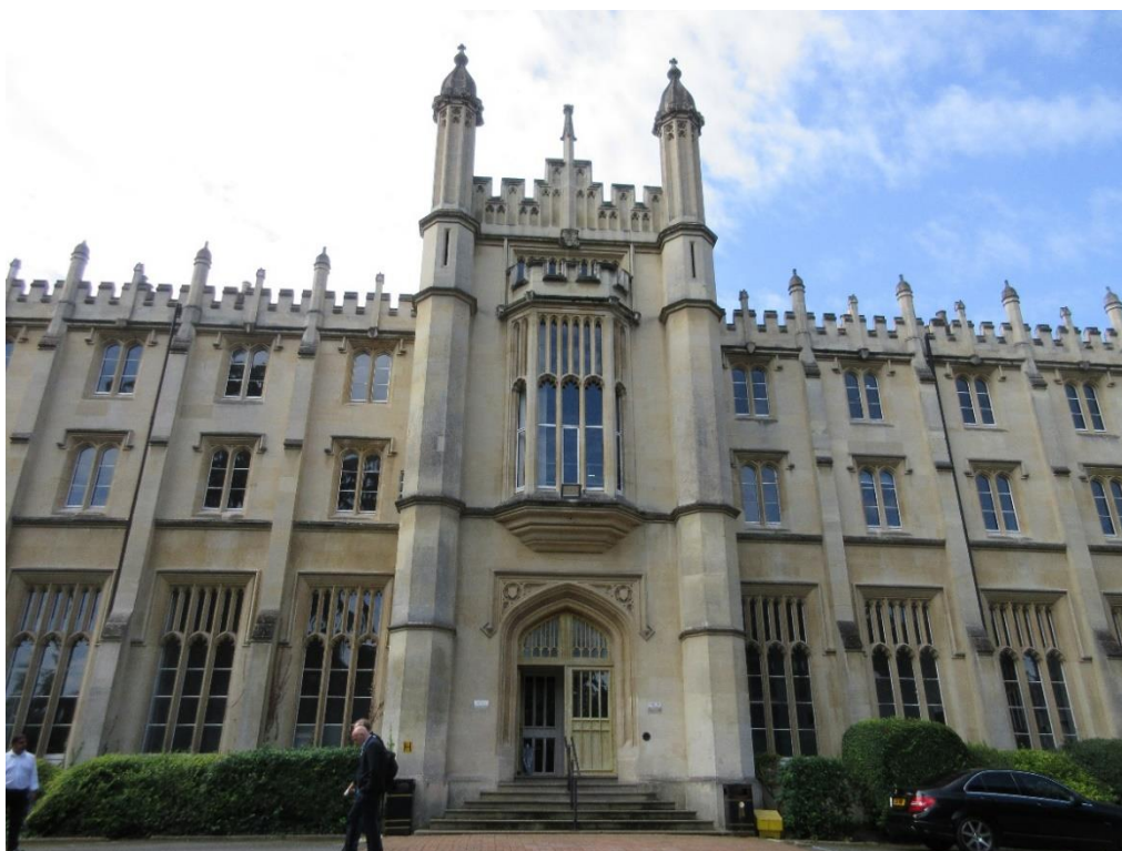
Figure 10: Front (north-east) elevation of the principal building.
