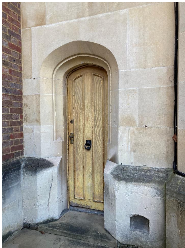
Figure 13: Side entrance door to south-east elevation. (See Figure 37, Appendix 4, for the interior of the door.)
