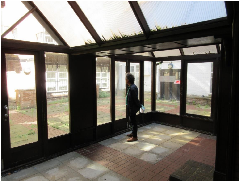
Figure 90: Basement floor of extension B.
