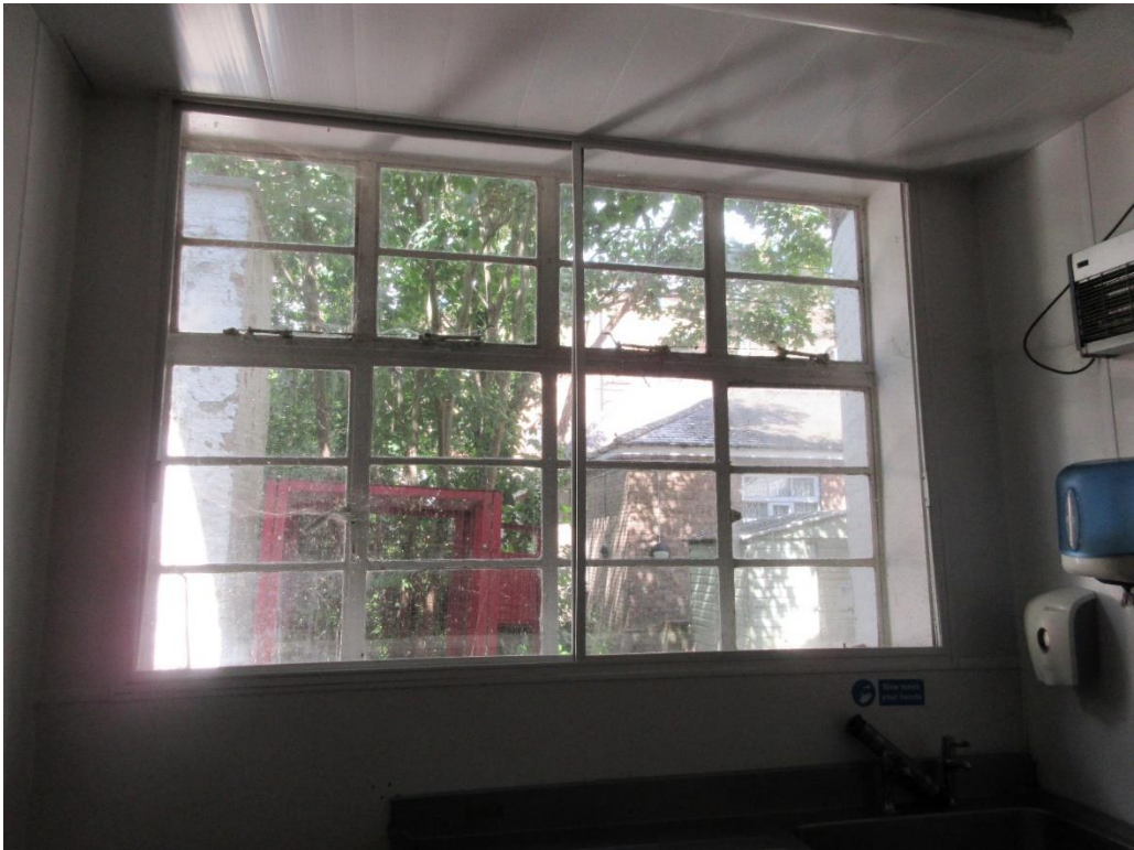
Figure 100: Ground floor of extension F.
