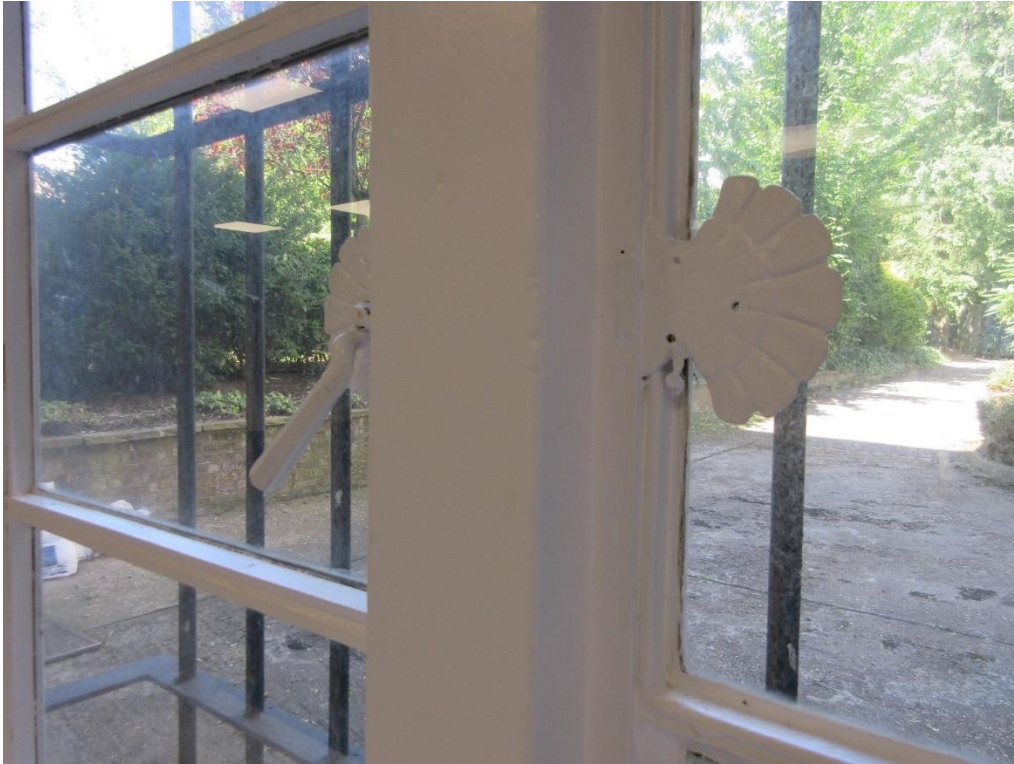
Figure 86: Basement of extension A – Ironmongery.
