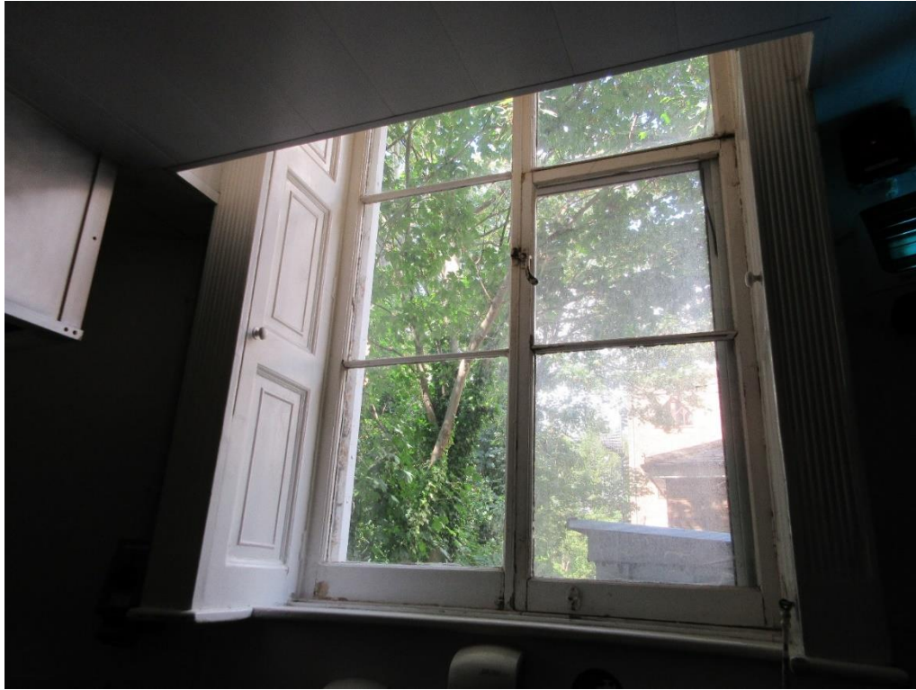
Figure 101: Ground floor of extension F.
