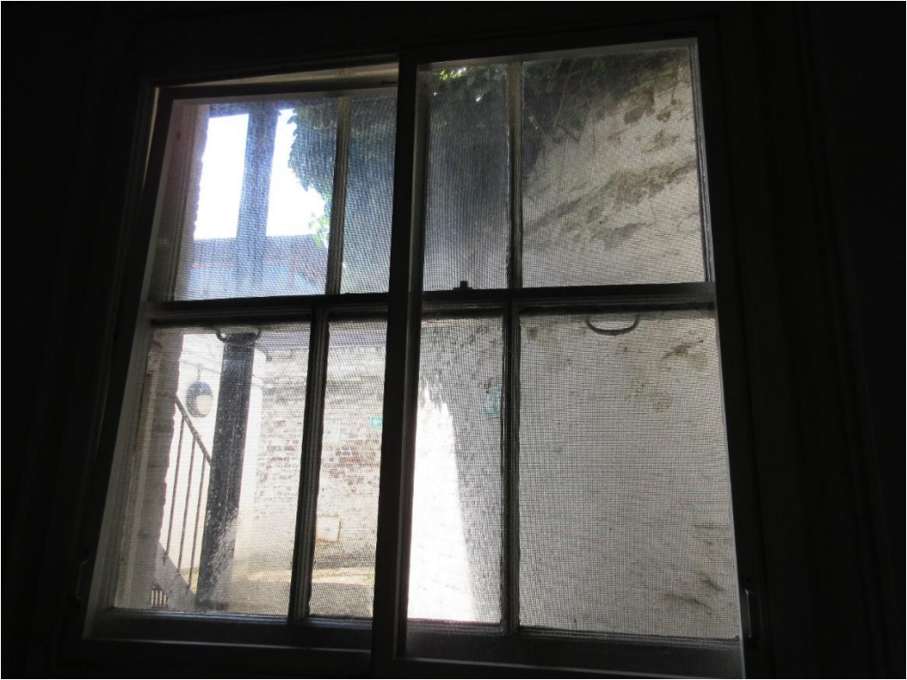
Figure 99: Ground floor of extension F.
