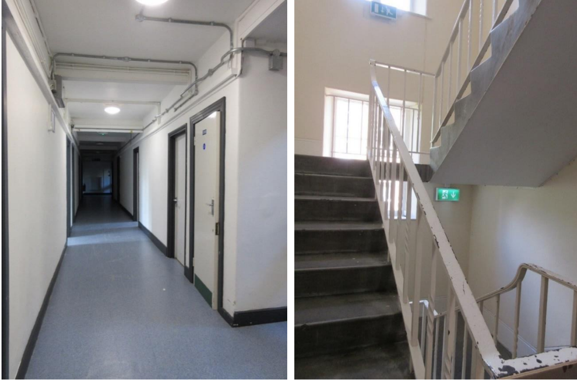
Figure 60 (left): Fourth floor corridor above central section of building.
