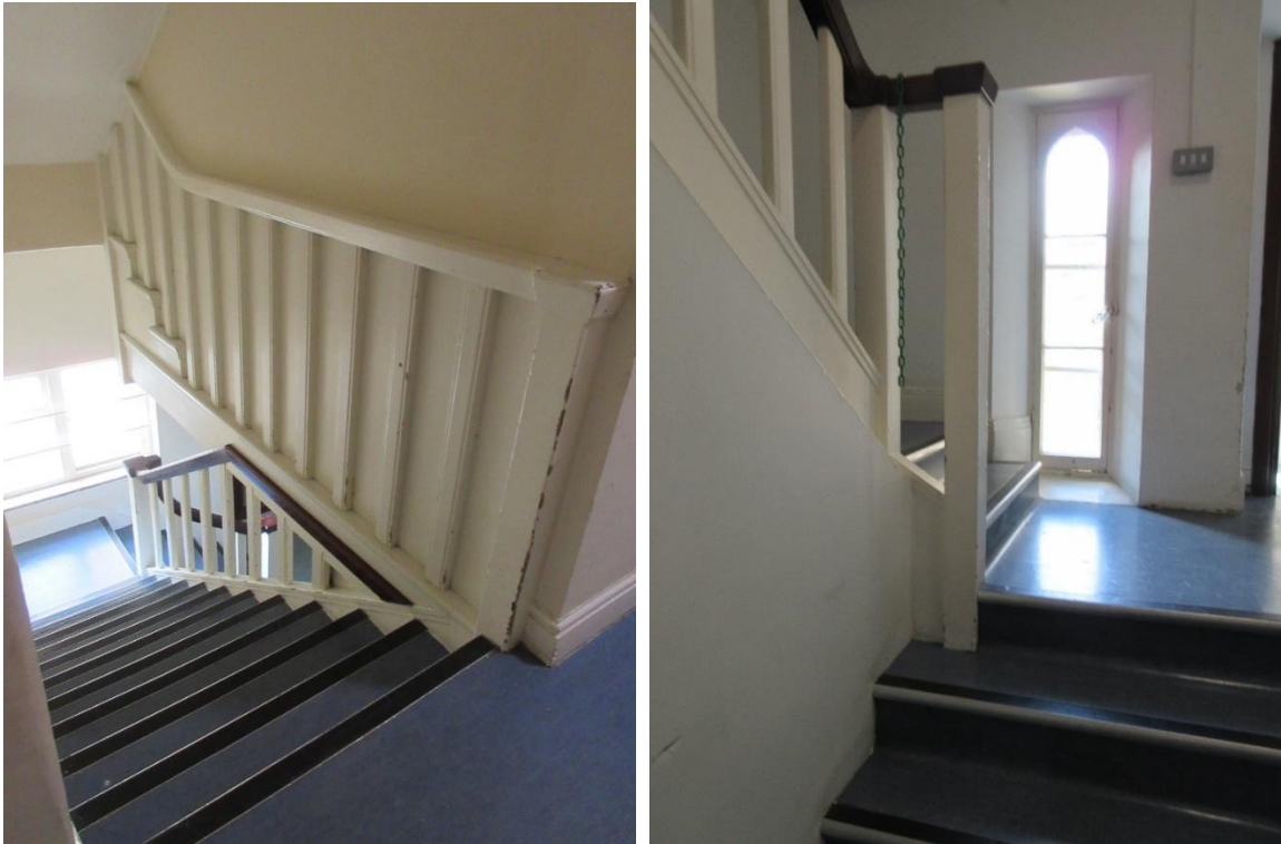
Figure 56 (left): Stairs between third floor and fourth floor.
