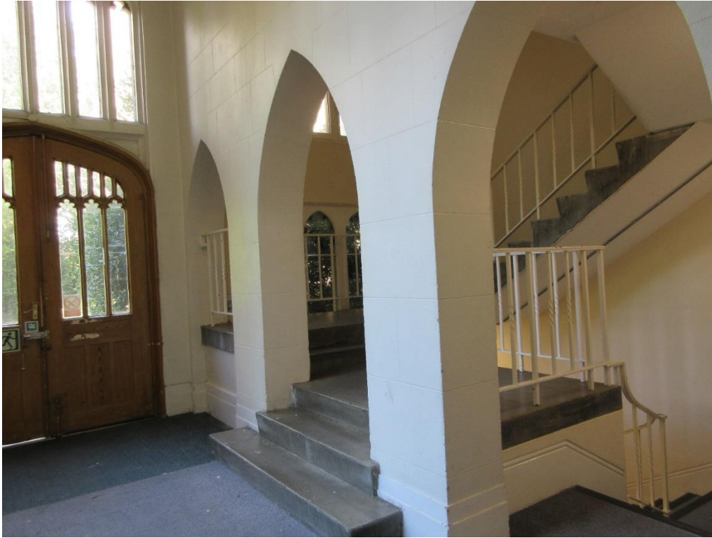
Figure 42: Secondary entrance (to north-west elevation).
