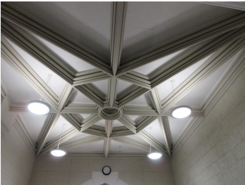
Figure 11: Ground floor – Hall (ceiling).
