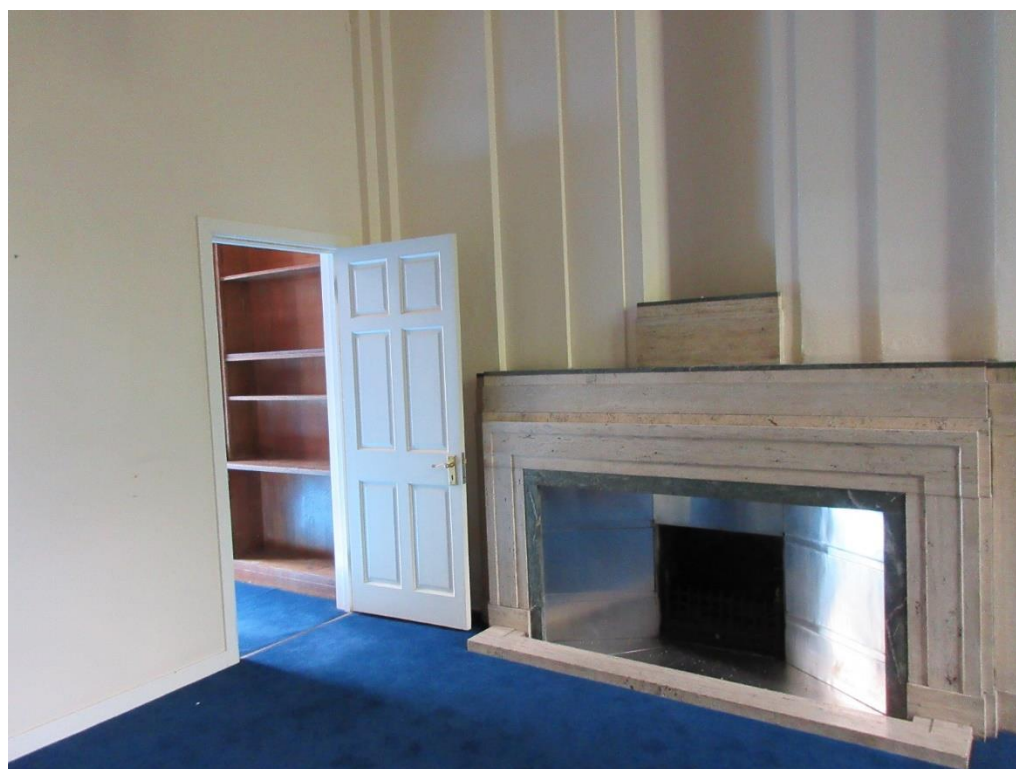
Figure 81: Ground floor of extension A. Note modern wall partitioning and door, and original 1930s fire surround.
