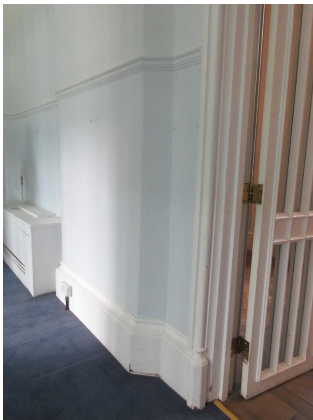
Figure 25: Ground floor – One of the rooms accessed from the north-west corridor. Note original architrave, skirting, and high “dado rail”.
