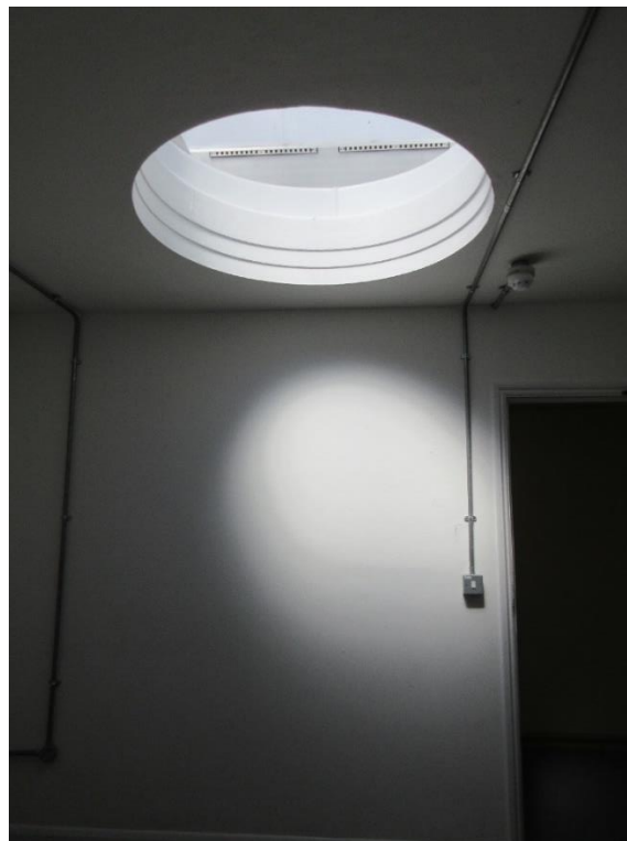
Figure 85: Second floor of extension A – Rooflight in one of the rooms.
