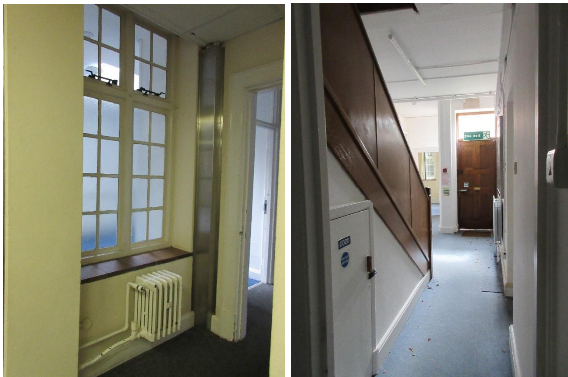
Figure 68 (left): Ground floor of George House – Corridor.
