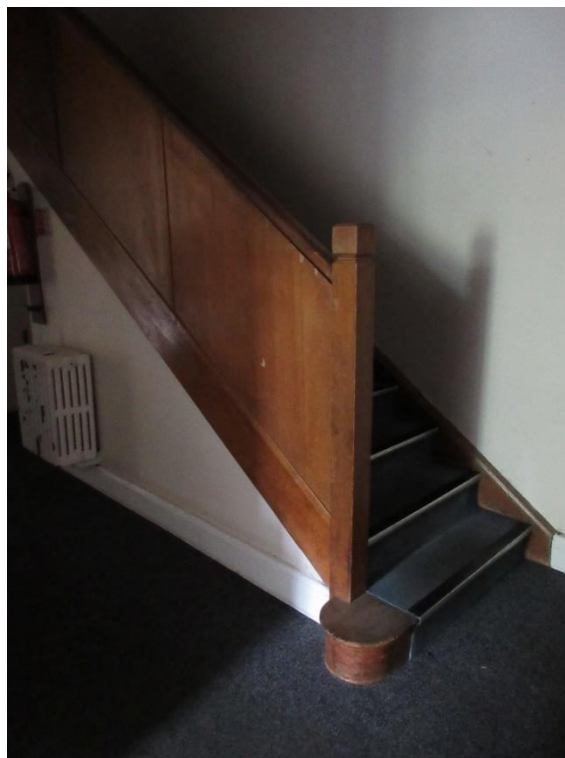
Figure 71: Ground floor of George House – North staircase.
