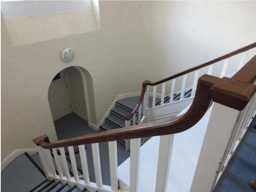
Figure 84: Stairs between second and third floors, with a door opening to extension A at second floor level.
