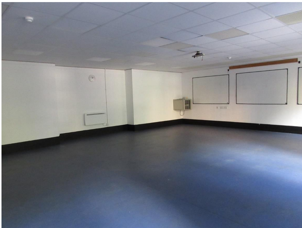
Figure 87: Basement of extension A.
