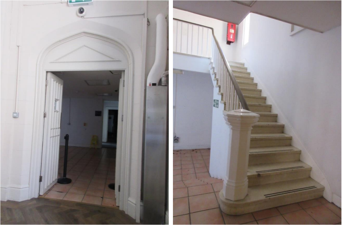
Figure 35 (left): Ground floor – South-east corridor, looking south-eastward towards end door. Figure 36 (right): Main staircase by the south wing.
