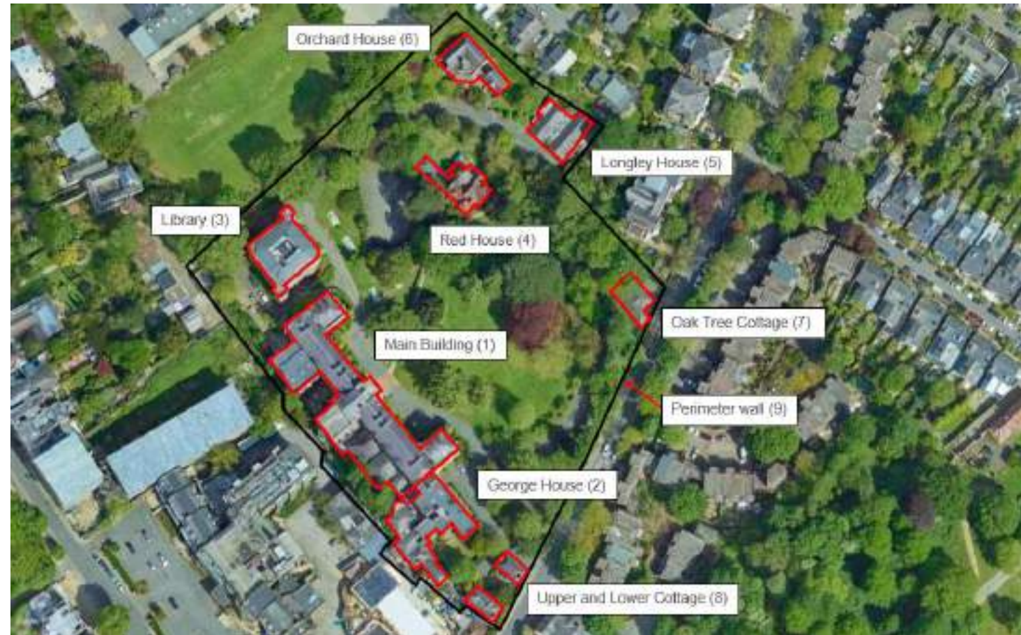
Site overview of existing buildings
