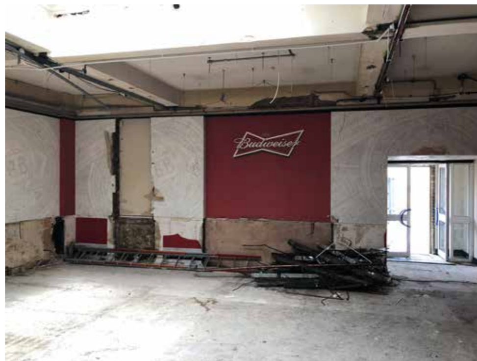
Stripout completed at eastern area canteen building
