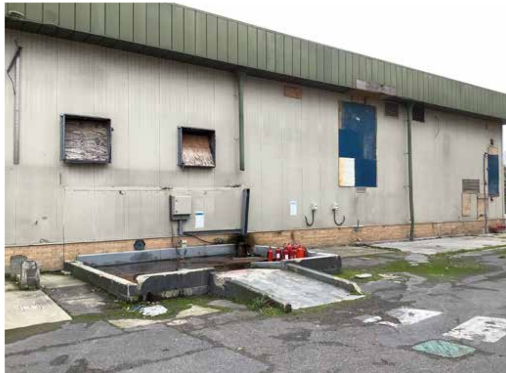
Bund for former oil tank at East Site bottling building, now removed from Site
