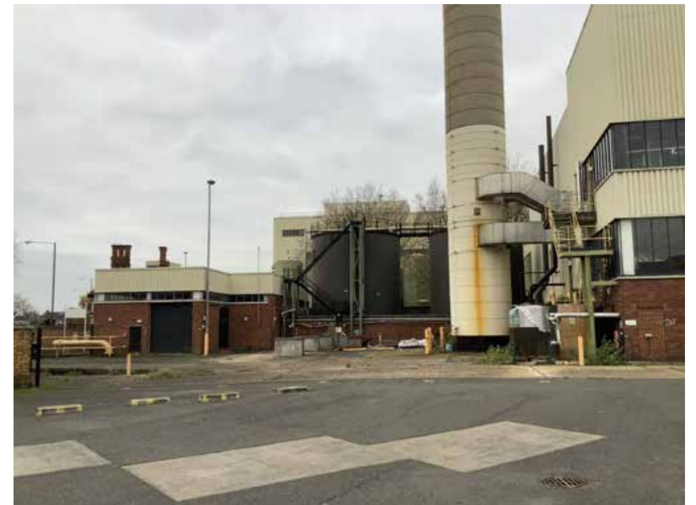
Remaining tanke south of Energy Centre at brewery East Site
