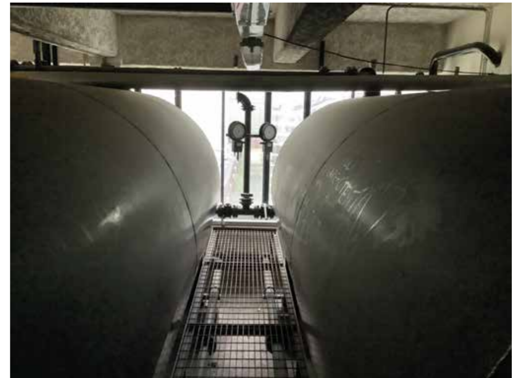
Residual former Dilac tanks at west site, empty but not yet removed
