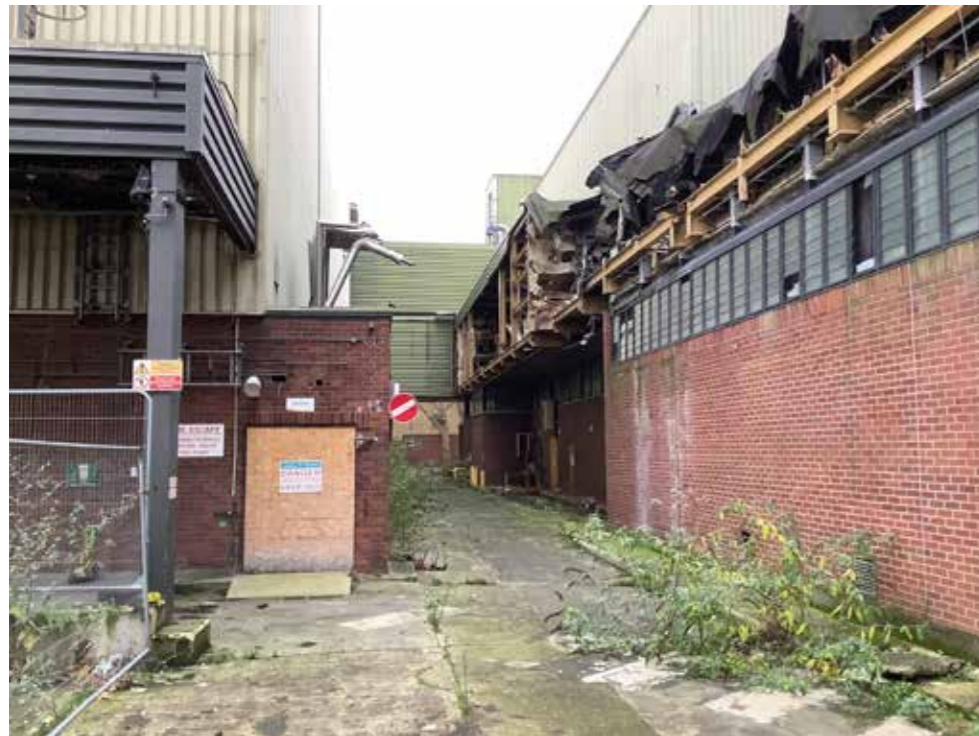
Partial demolition of West Site brewery structures as part of tank removal
