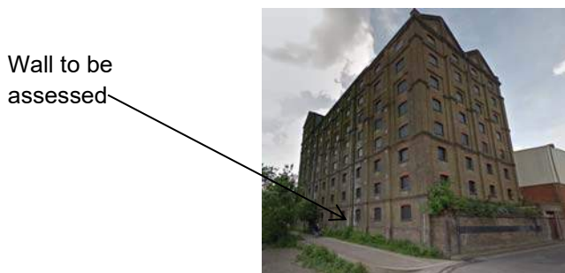
Figure 3: Wall to be assessed
