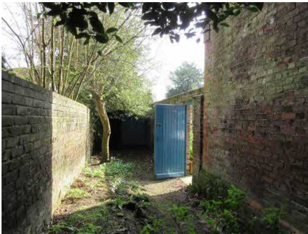
Figure 59: Area by side passageway (north side), with timber door leading to rear garden.
