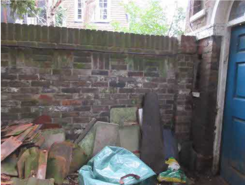
Figure 77: Boundary wall adjacent to room to east of wash house.
