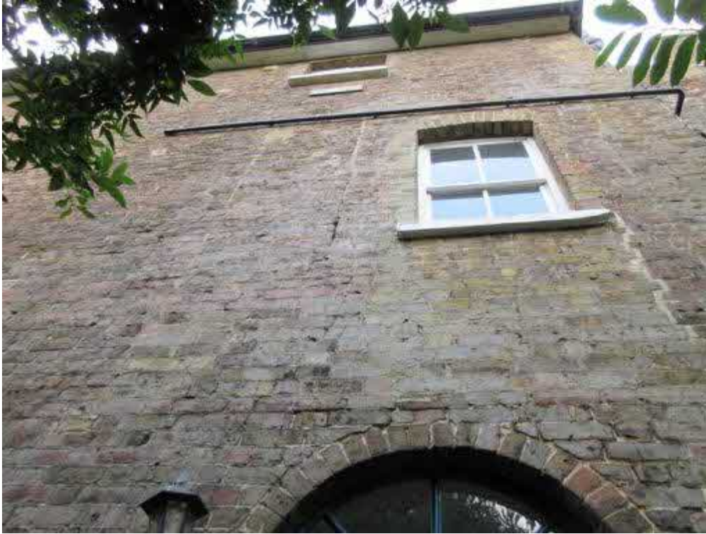
Figure 61: Side (north) elevation above side entrance. Note bricked in window opening.
