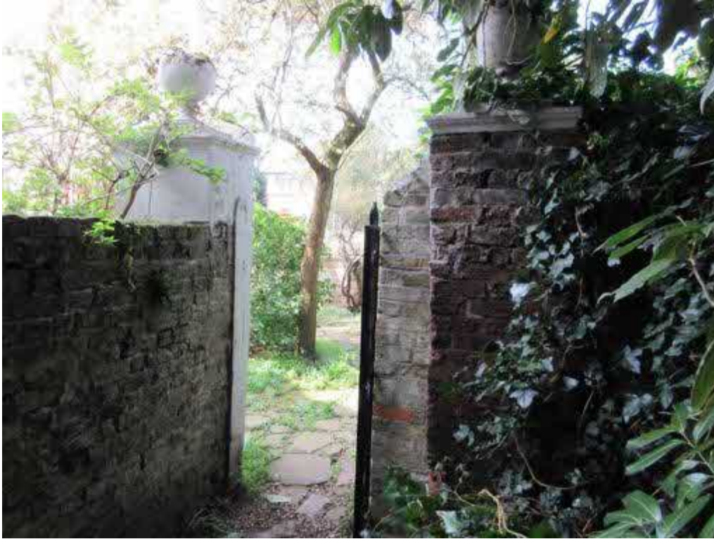
Figure 63: Side entrance piers. (See also Figure 45.)
