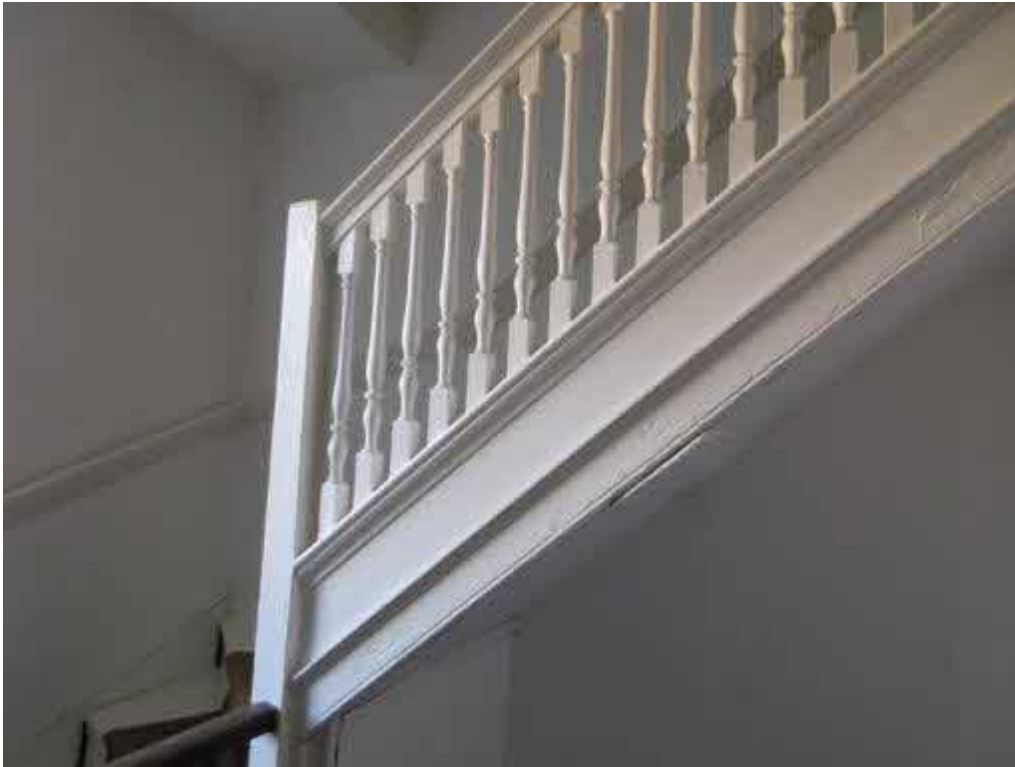
Figure 131: Stairs to Flat 90A.
