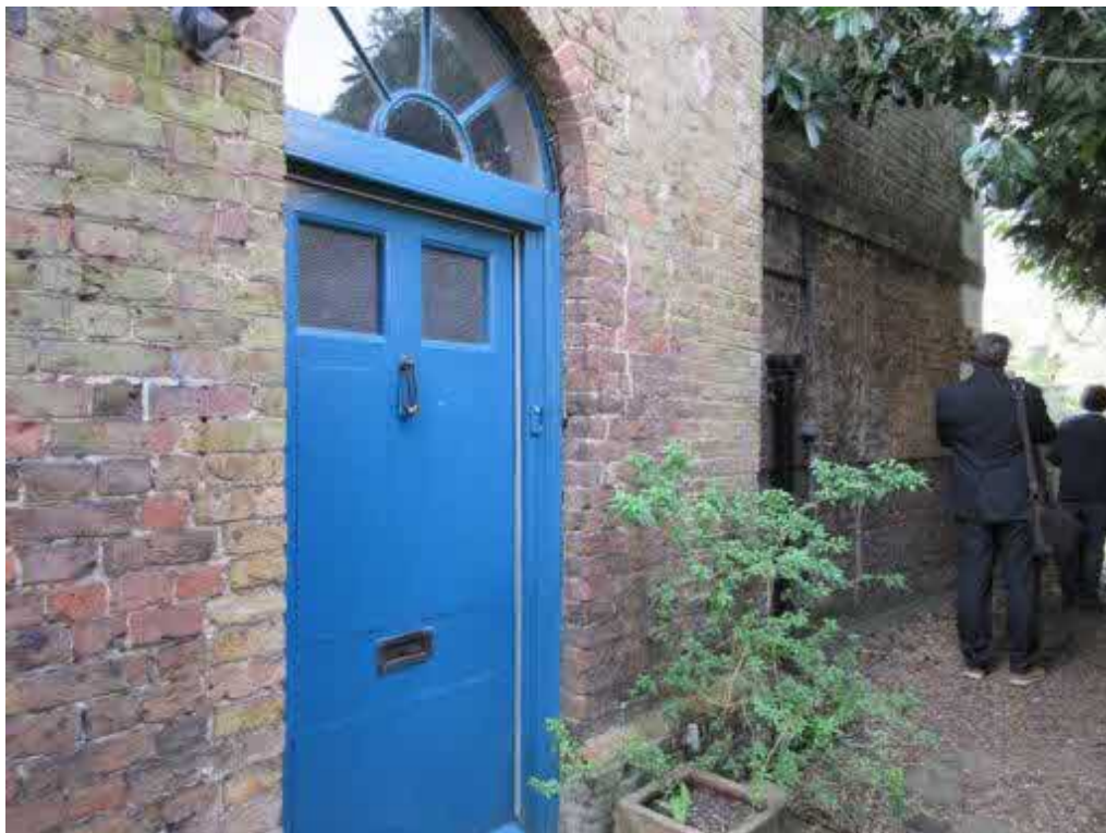
Figure 62: Side entrance (to Flat 90A), and side access (north side) between front garden and rear garden.
