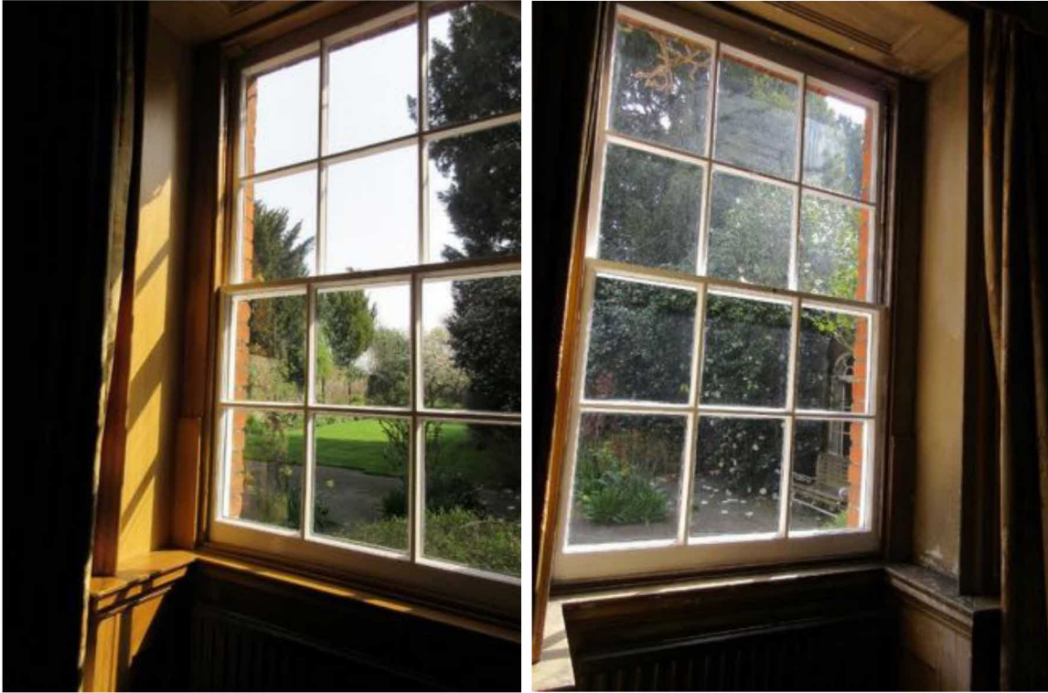
Figure 101 (left): Ground floor – North window to rear dining room.
