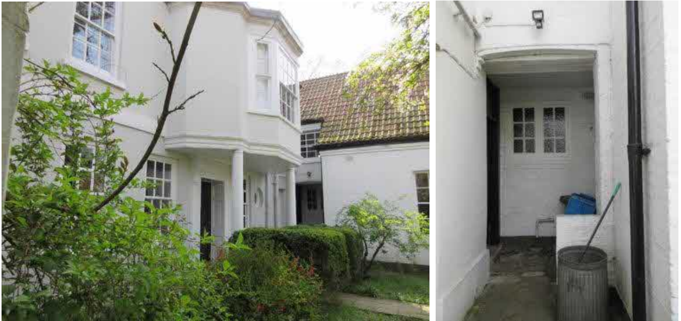
Figure 40 (left): Front elevation and garden, and side (north) elevation of garage/Flat 90B.
