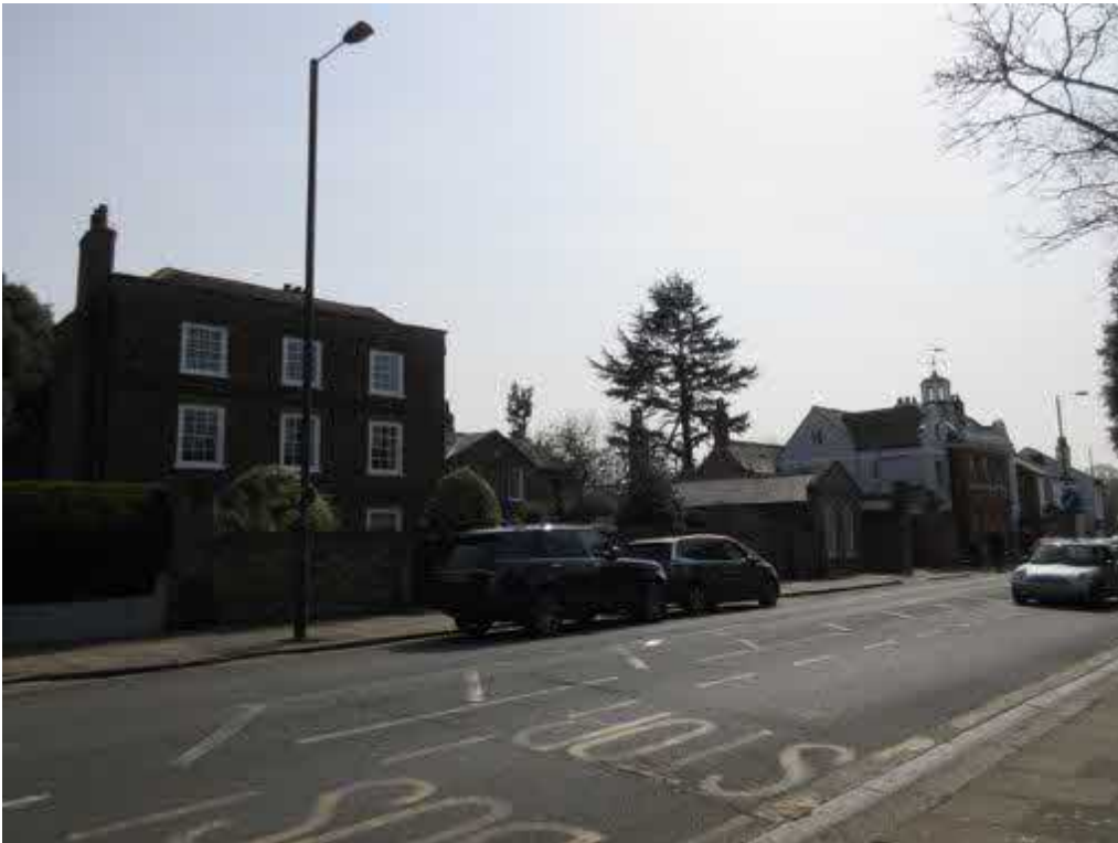
Figure 10: No. 84 (Grade II), no.s 80 & 82 (Grade II) and no. 78 (Grade II) High Street.
