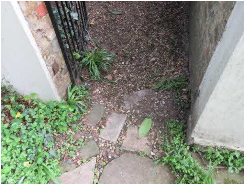
Figure 46: Gate piers to side entrance. Note different front building lines.
