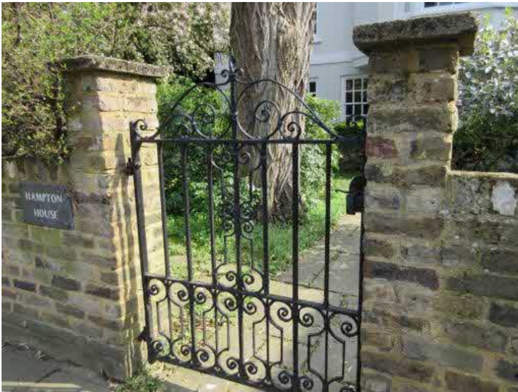
Figure 44: Front gate and piers.
