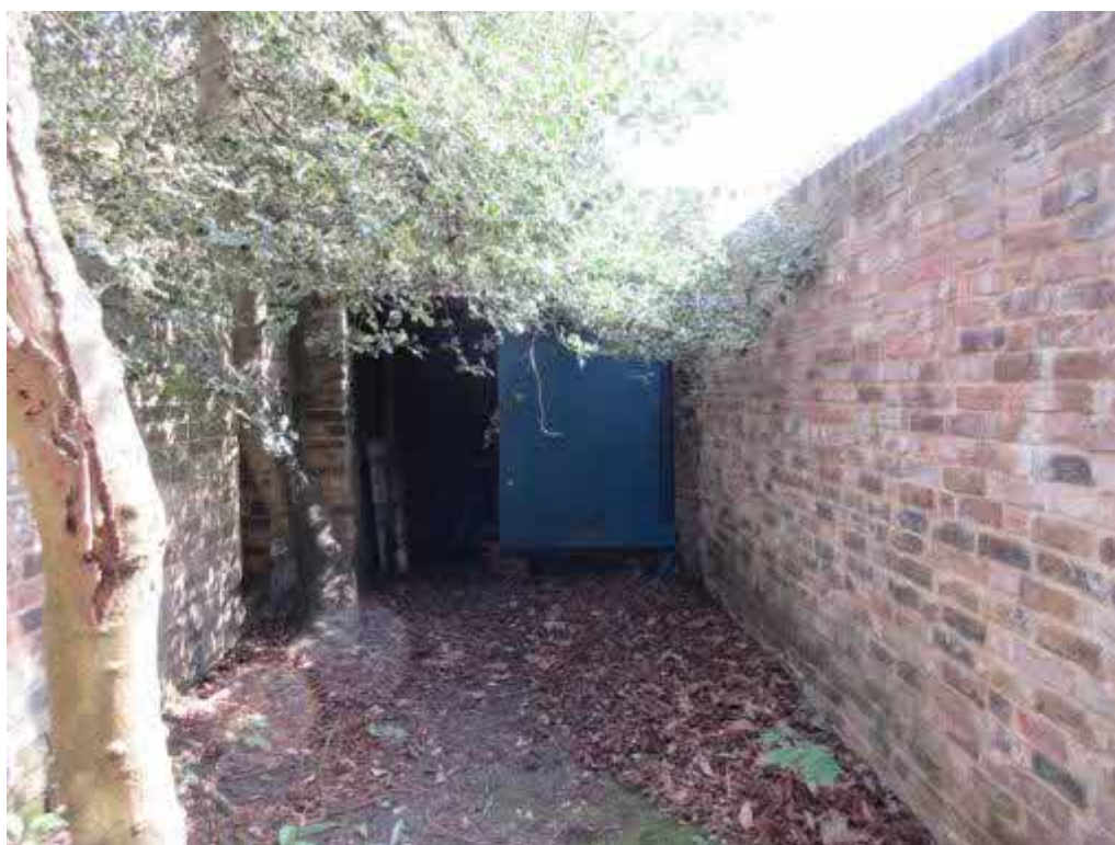
Figure 60: Storage area by side passageway (north side).
