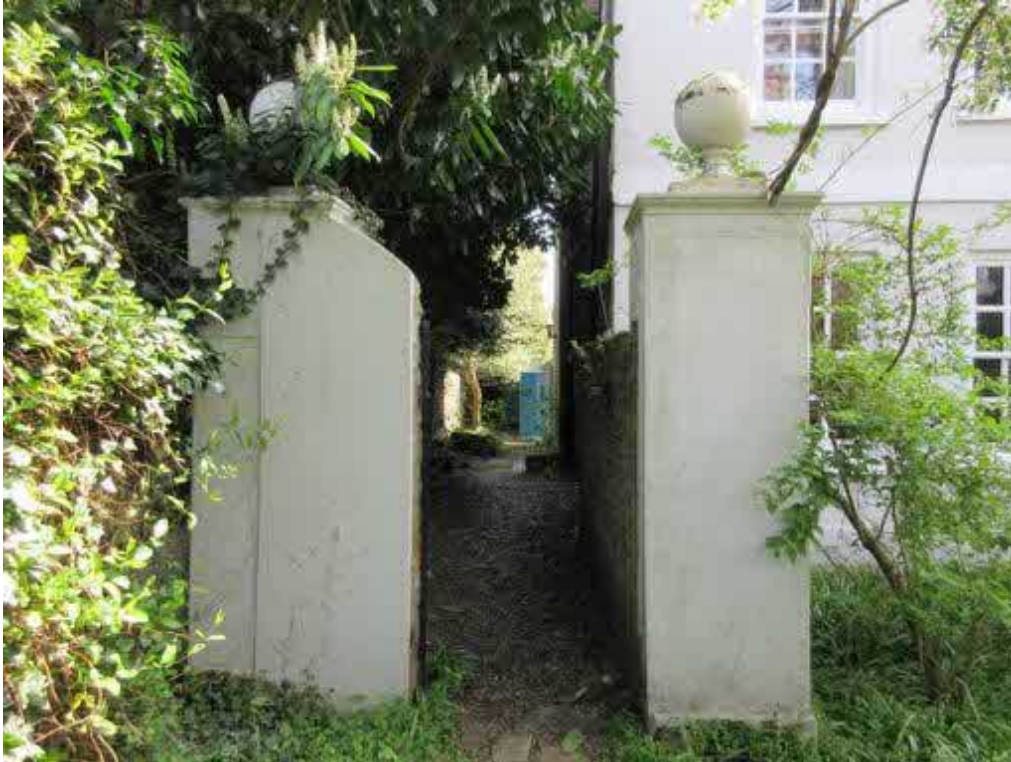
Figure 45: Side entrance gate piers.
