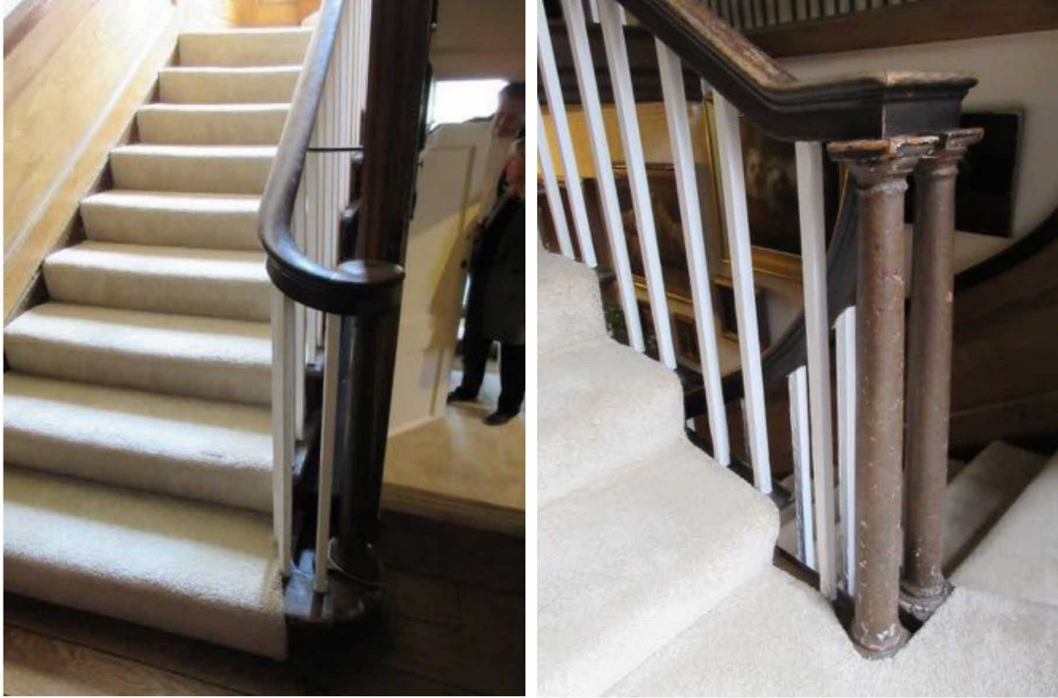
Figure 104 (left): Ground floor – main staircase.
