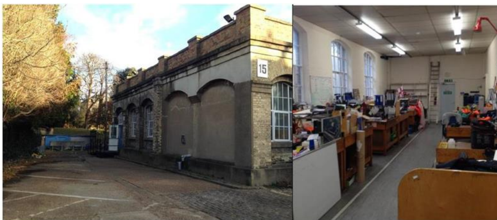
Photo 1 (Ruston Building- formerly Office/Workshop)
