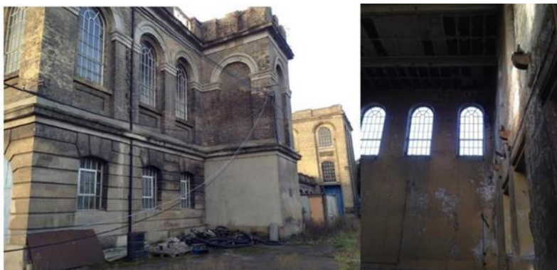
Photo 4 (Karslake Building- The Bull)
