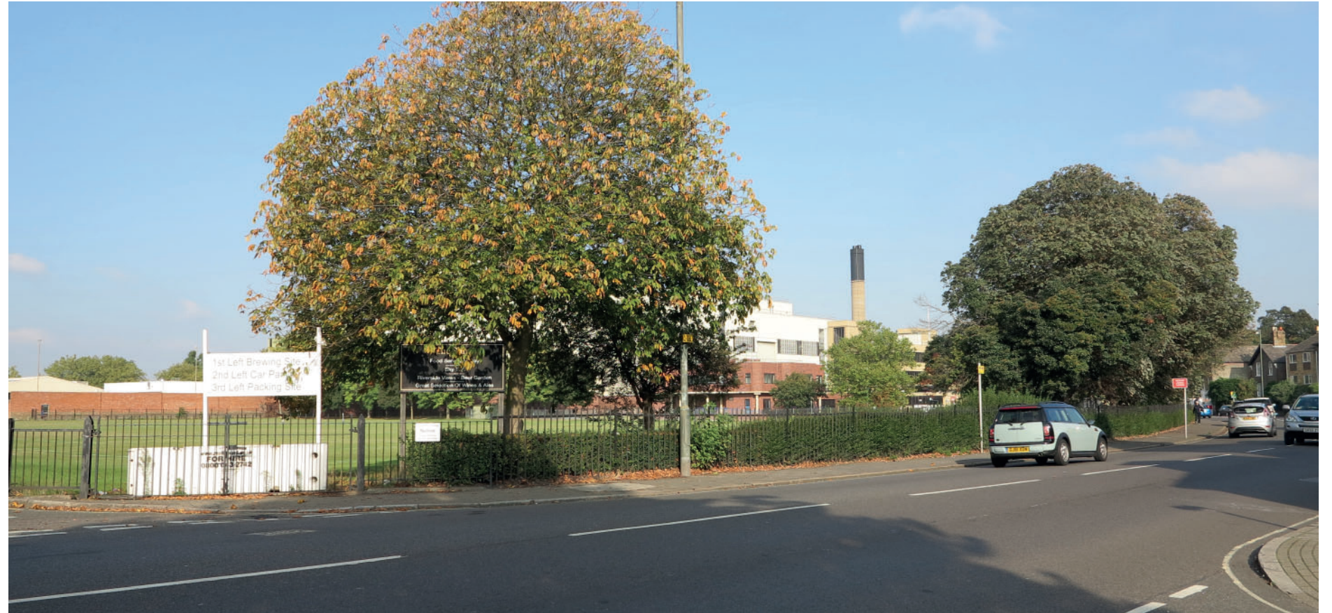
View along Lower Richmond Road - from West
