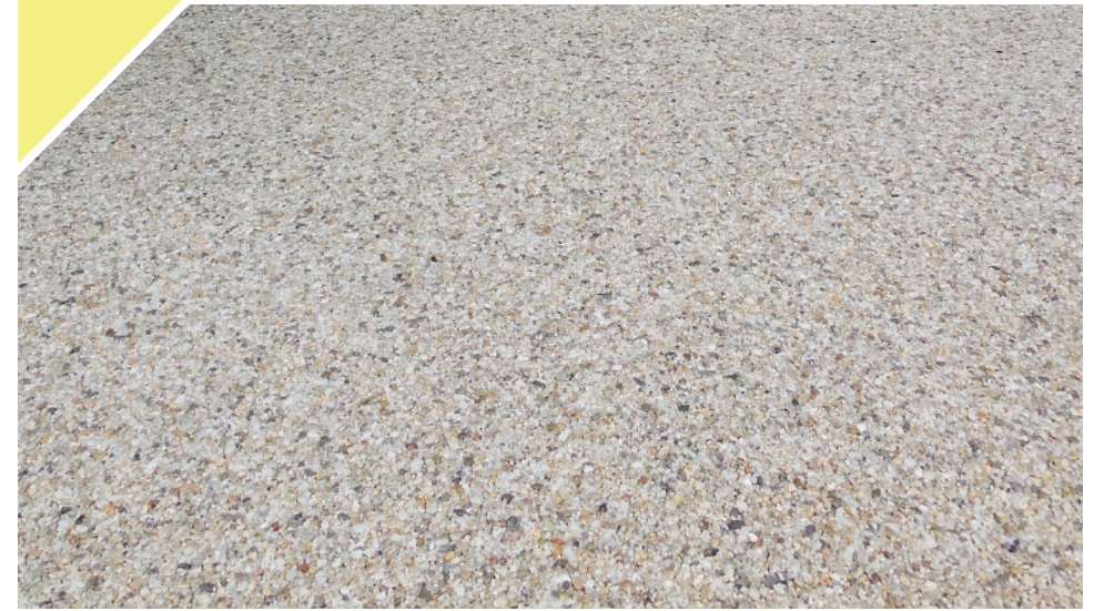
Resin Bound Aggregate
