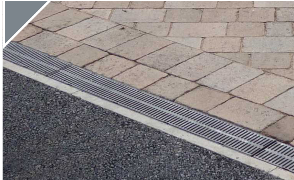
Hot Rolled Asphalt
