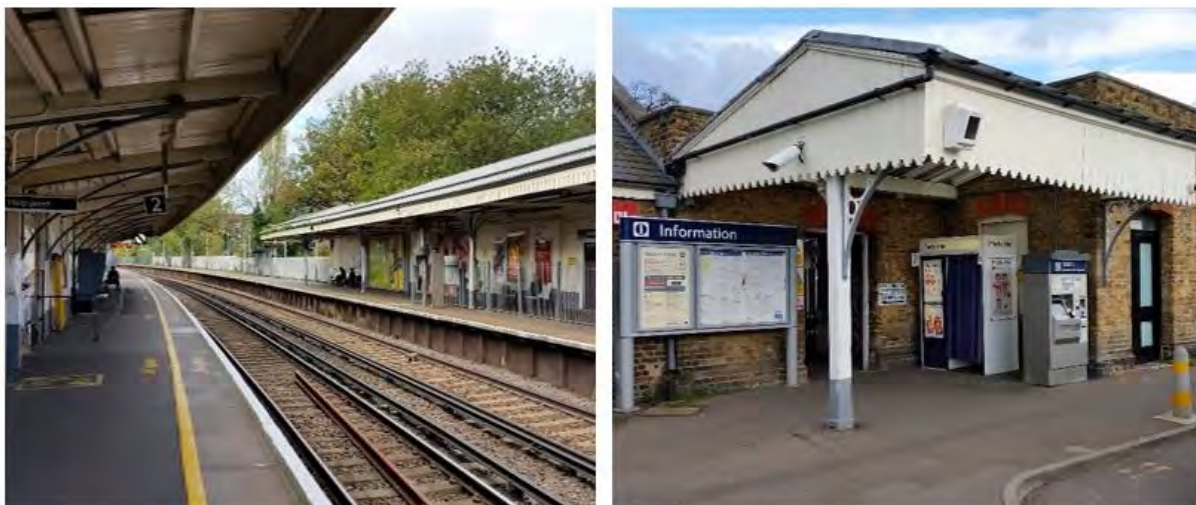
Figure 4-9: Mortlake Station Platforms and Its Southern Entrance
