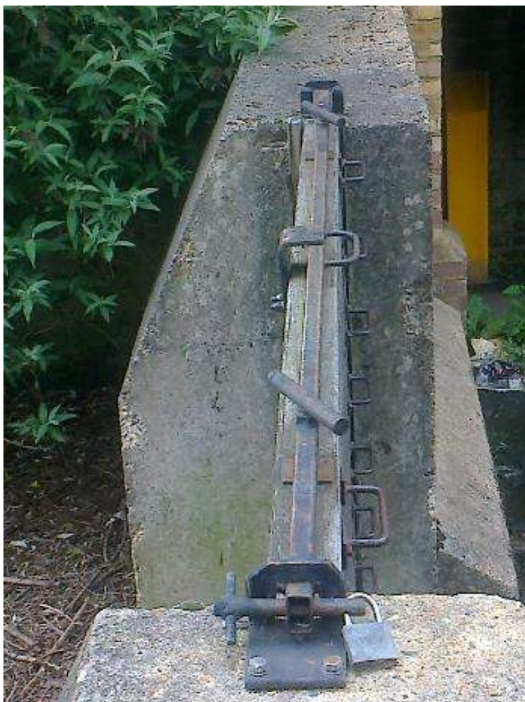
Figure D-5 Stop-logs at Bull's Alley – from above
