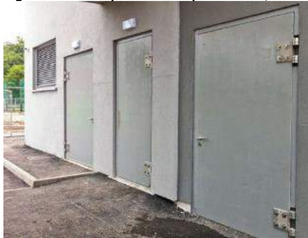
Figure 4-17 Examples of flood proof doors, suitable for sub-station facility
