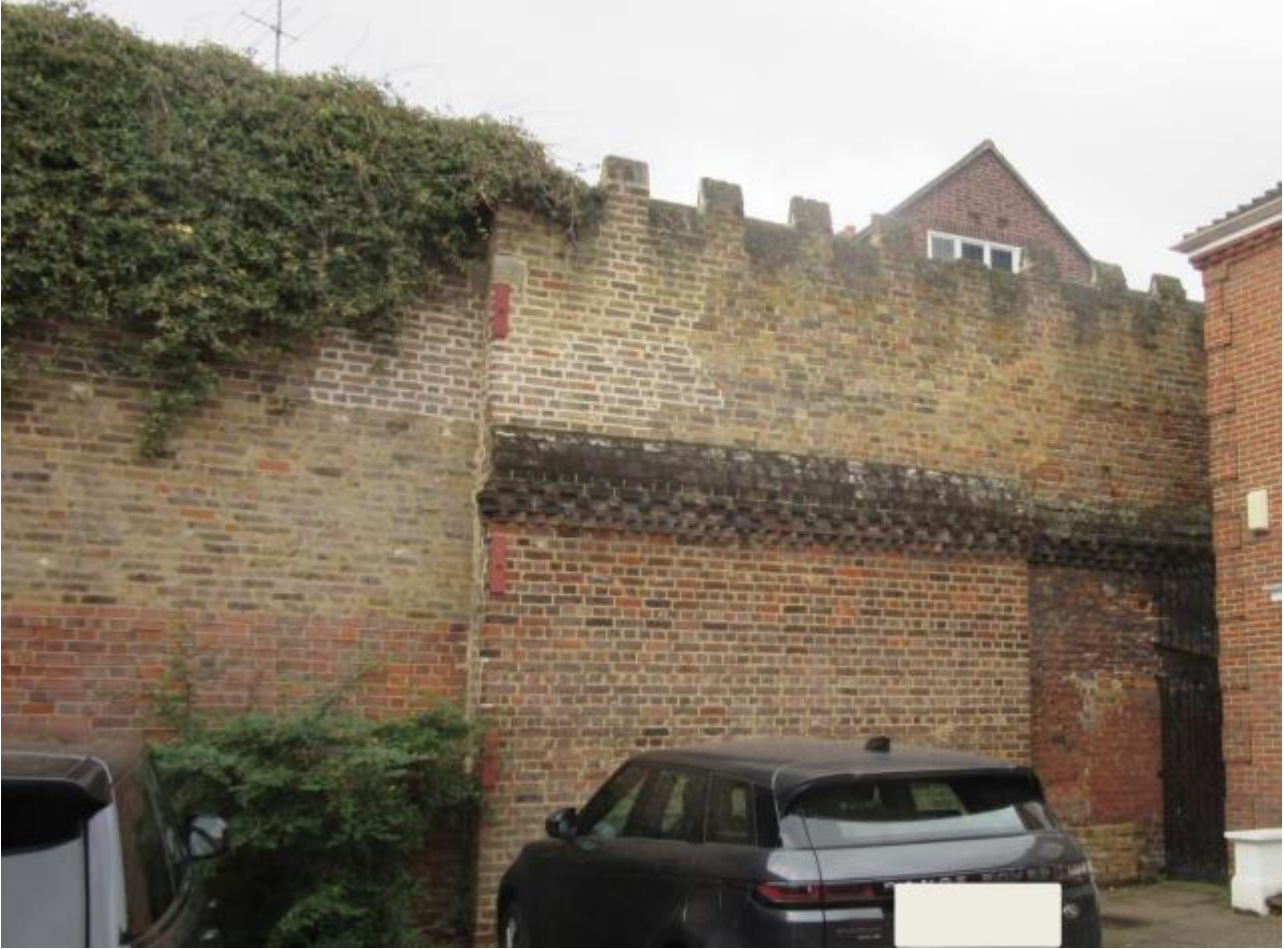
Figure 4 - The older (possibly Tudor) crenelated brickwork is set away from Hunters Lodge (see Figure 3).
