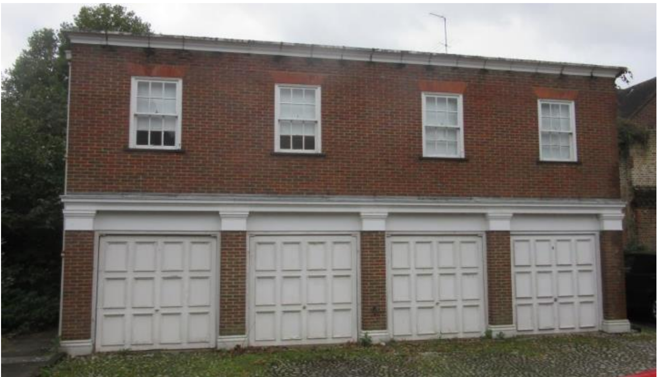
Figure 2 - The front (north-east) elevation of Hunters Lodge.
