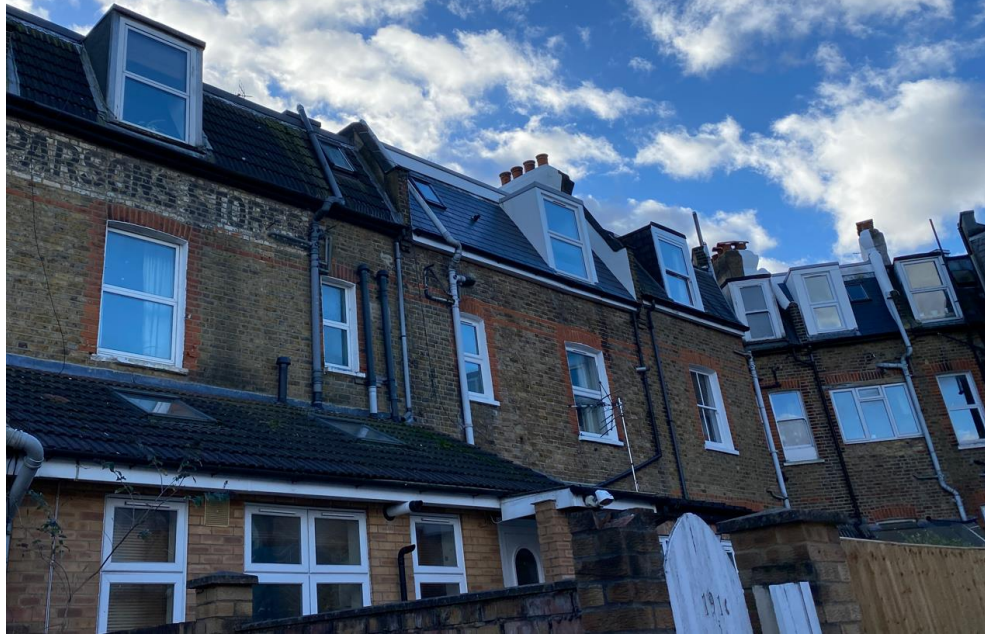
Fig 6: View of the rear elevations of 183 – 191 Richmond Road, whereby virtually all windows are replacement uPVC “two-pane” style casements
