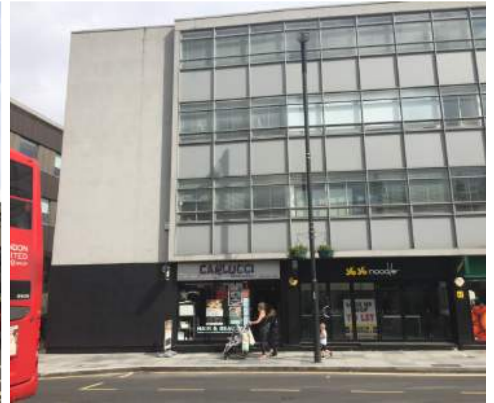
Northern end of the building on Kew Road
