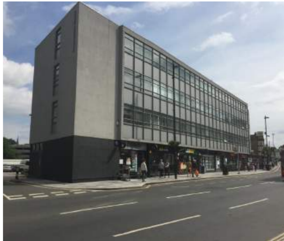
View from the north west
