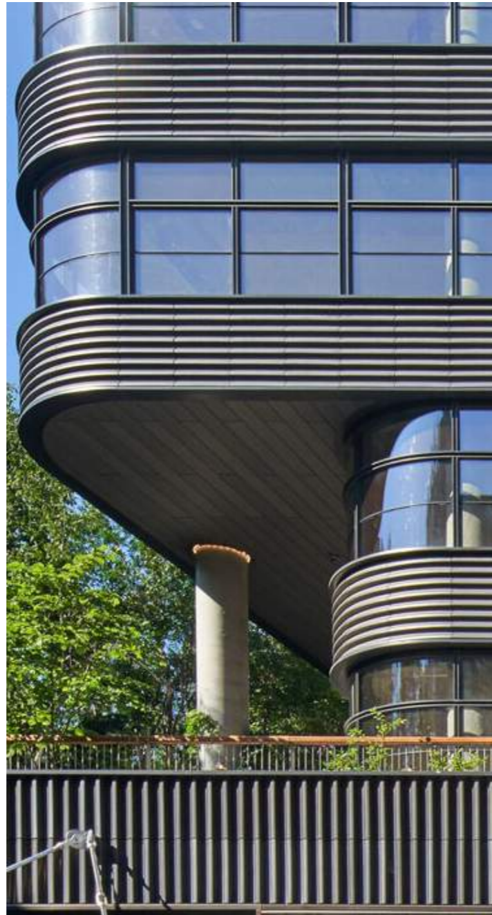
Ribbed terracotta rainscreen cladding to the office level spandrel panels, in glazed dark grey.
