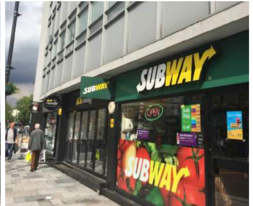
Typical ground floor retail in Westminster House
