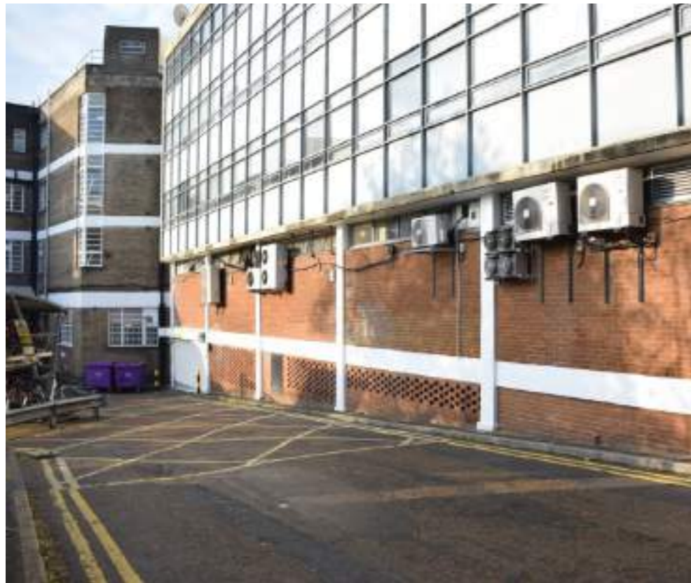
Sloping access road to the east (rear)
