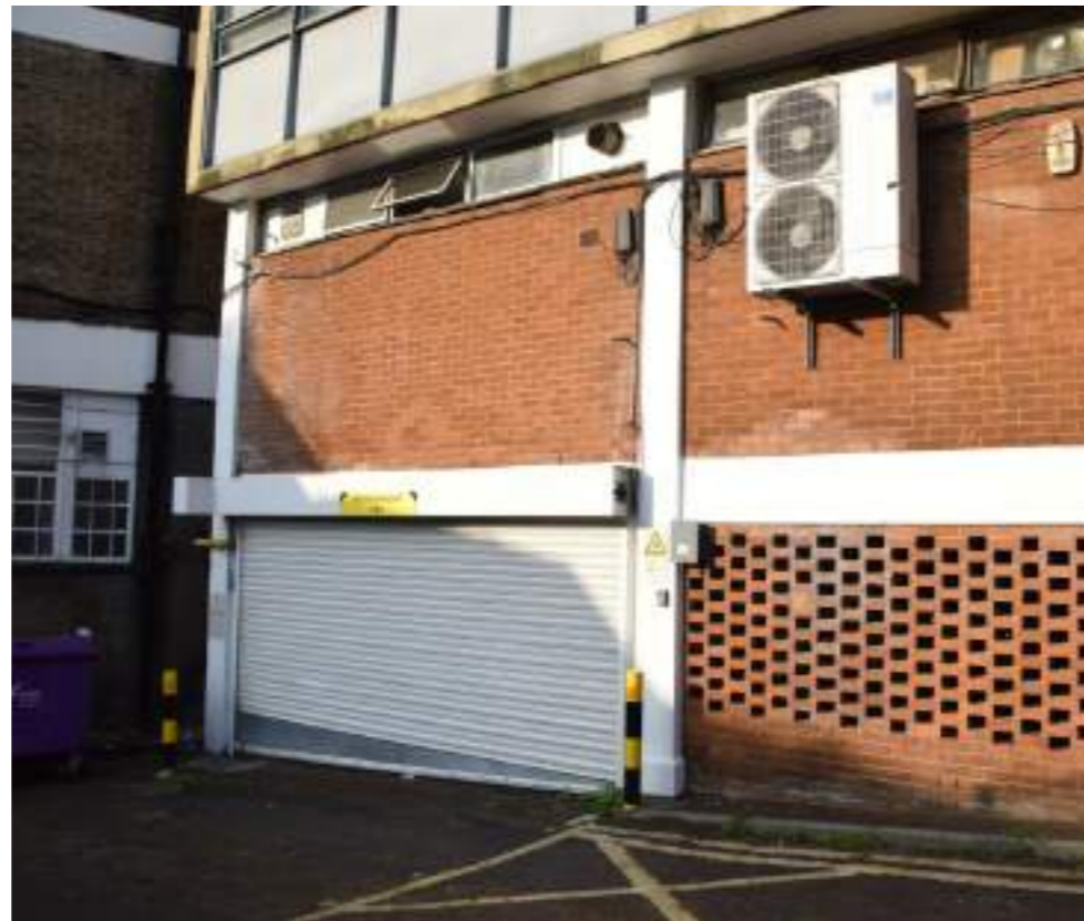
Basement level access from rear
