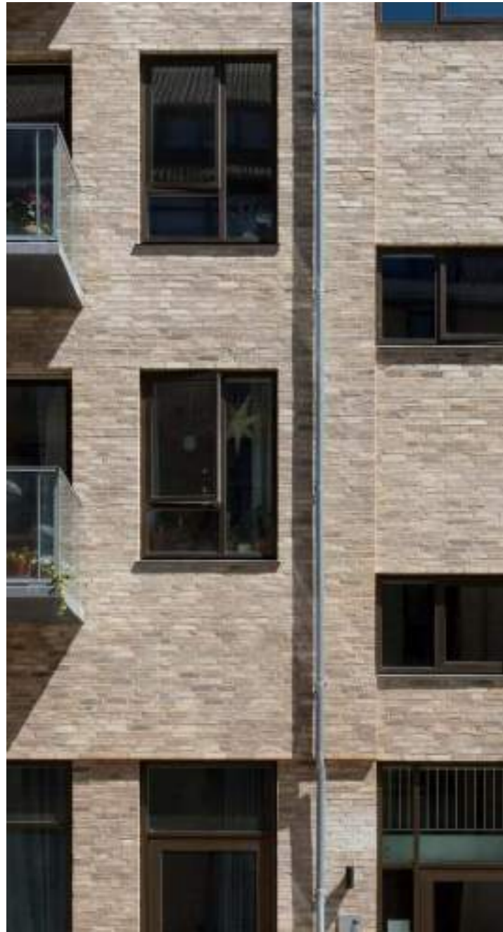
Grey/beige brick to the north and south facades – panellised brick slip system.
