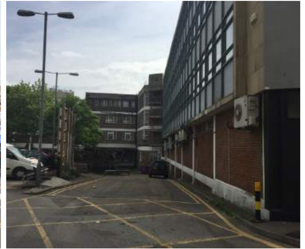
Sloping access road to the east (rear)
