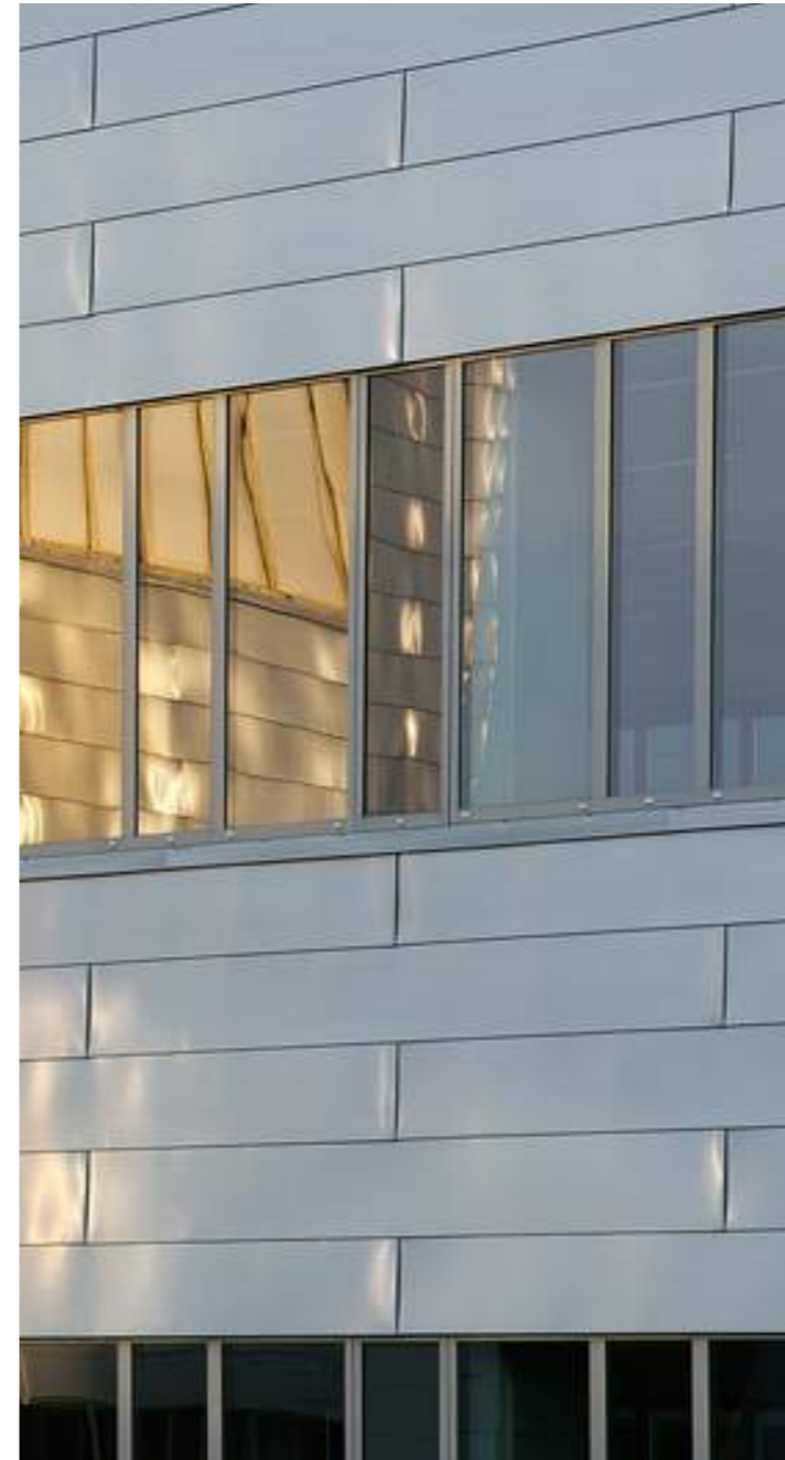
Silver/blue anodized aluminium (or similar) cladding to upper storey facades.
