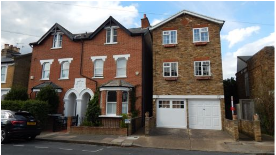
Image 01 – Front : South Elevation – No17 left, No19 centre, No19b at right, No21 extreme right.
